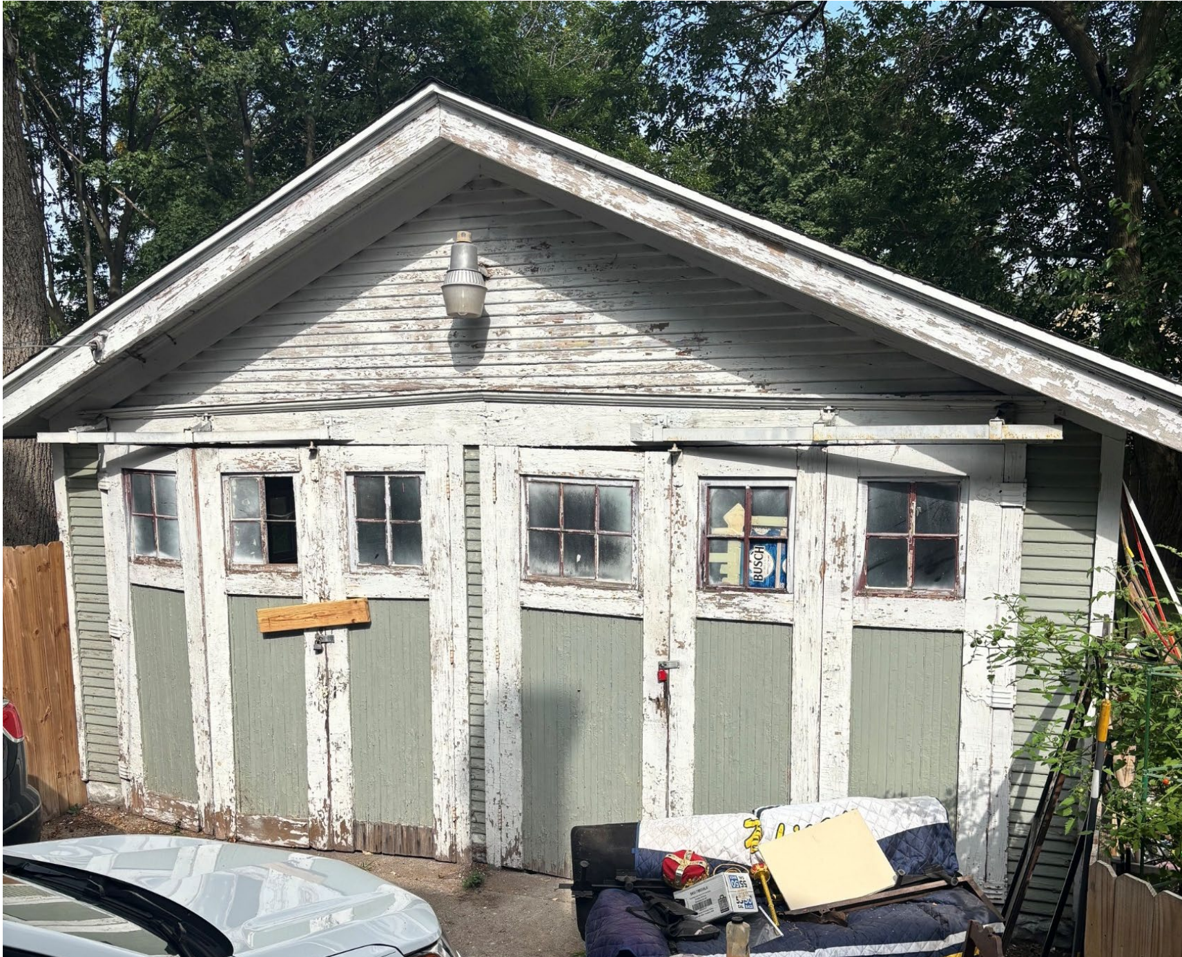
Existing garage doors.
