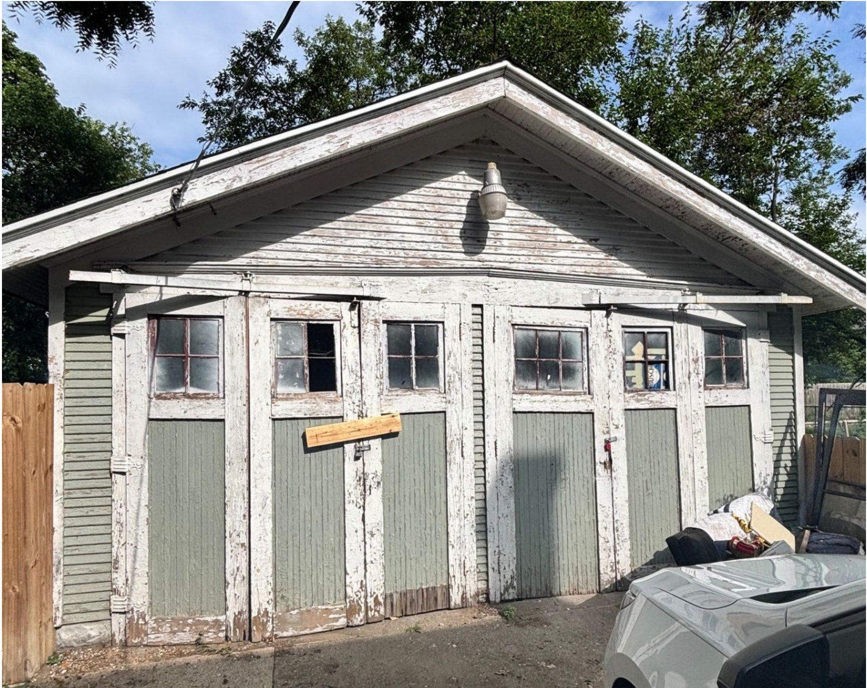
Existing garage doors.
