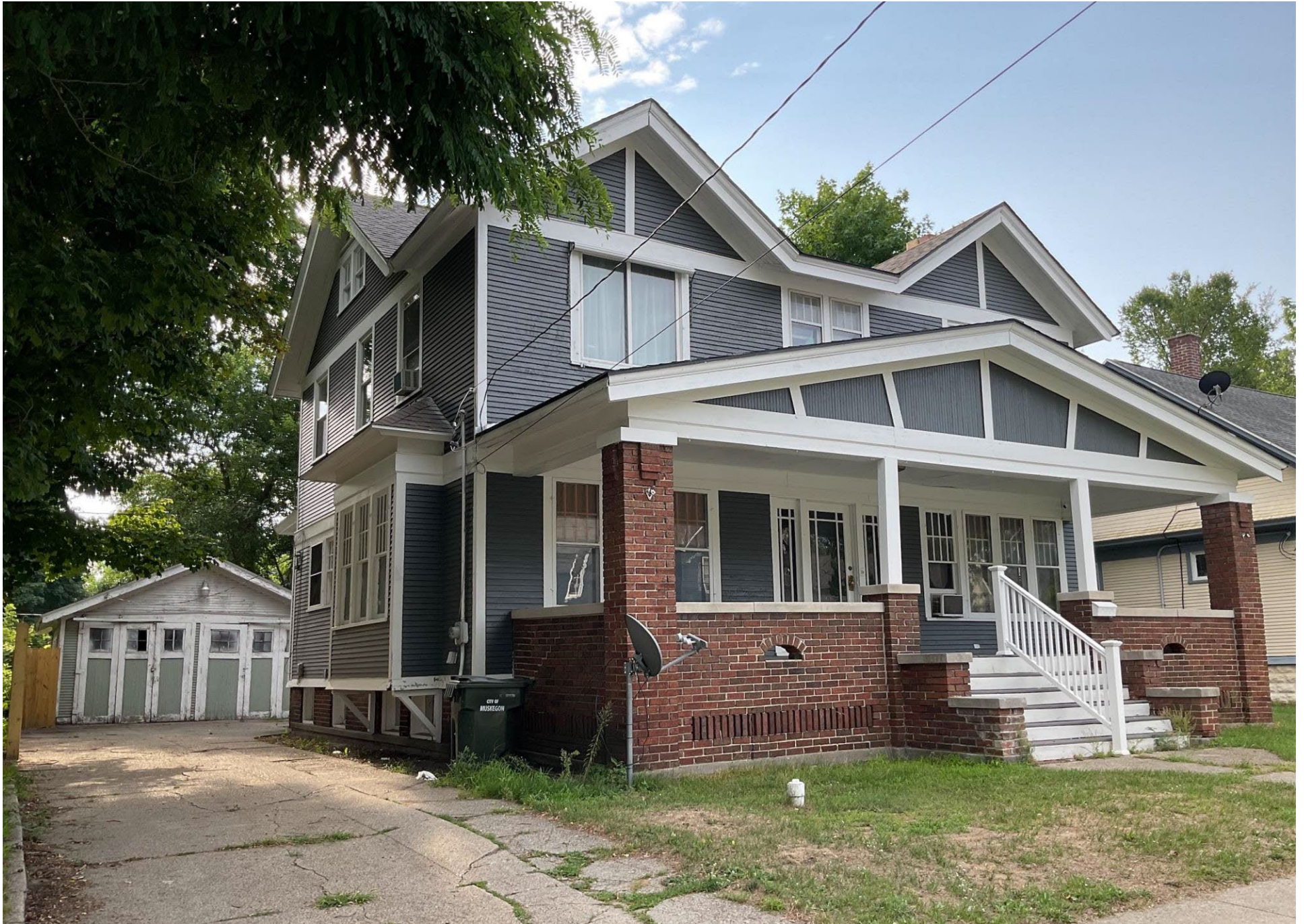
House and garage viewed from Clinton Street, looking east (photo from August 2023).
