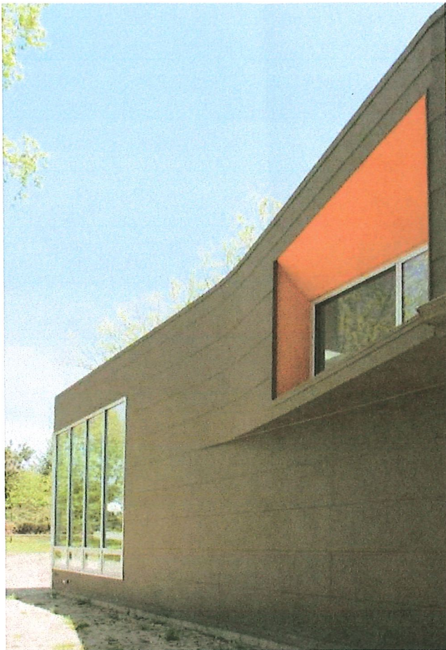
- The loft window at the second floor projects beyond the wall below, turning a functional element into a feature from street.
