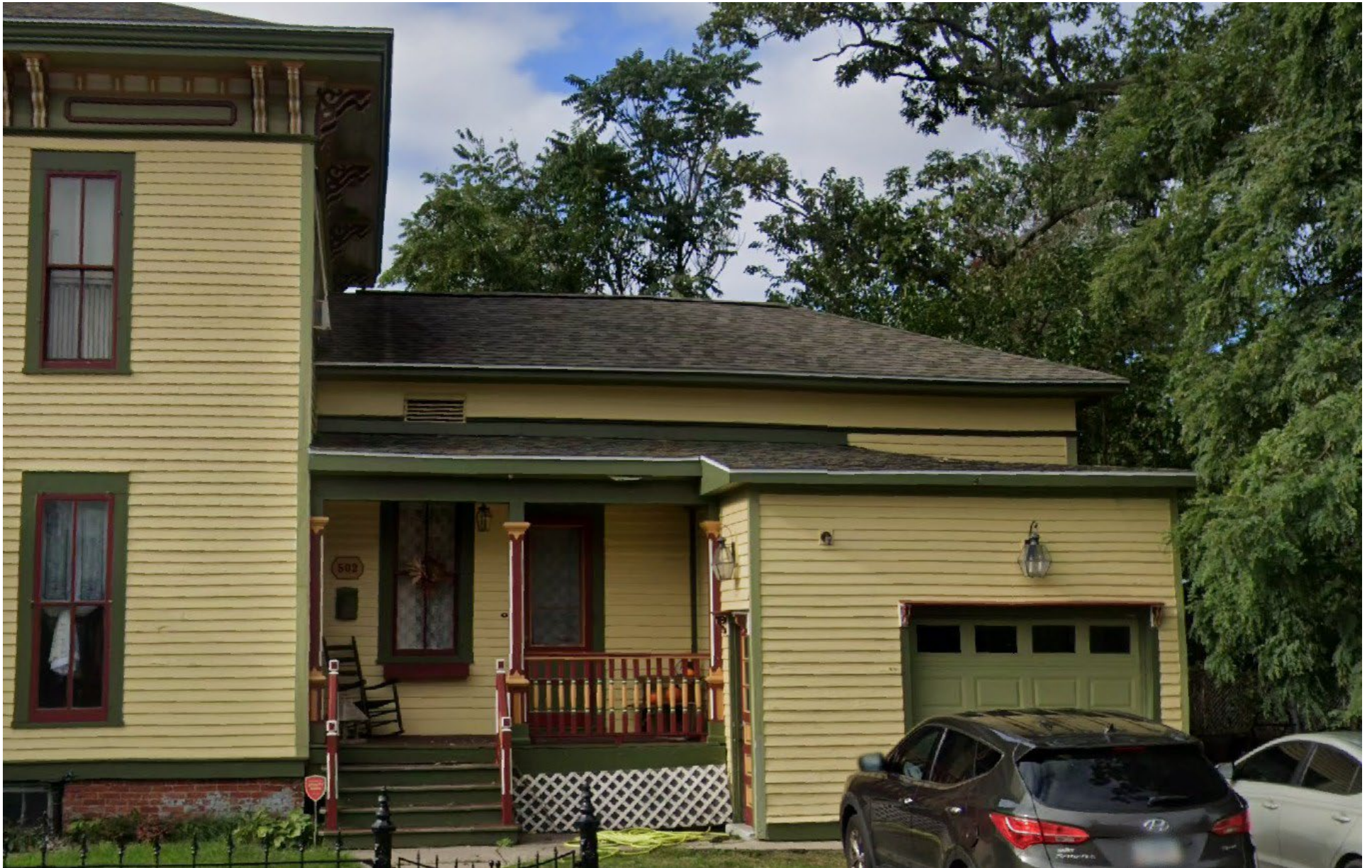
View of rear addition from 6 th Street prior to fire (photo from October 2019).
