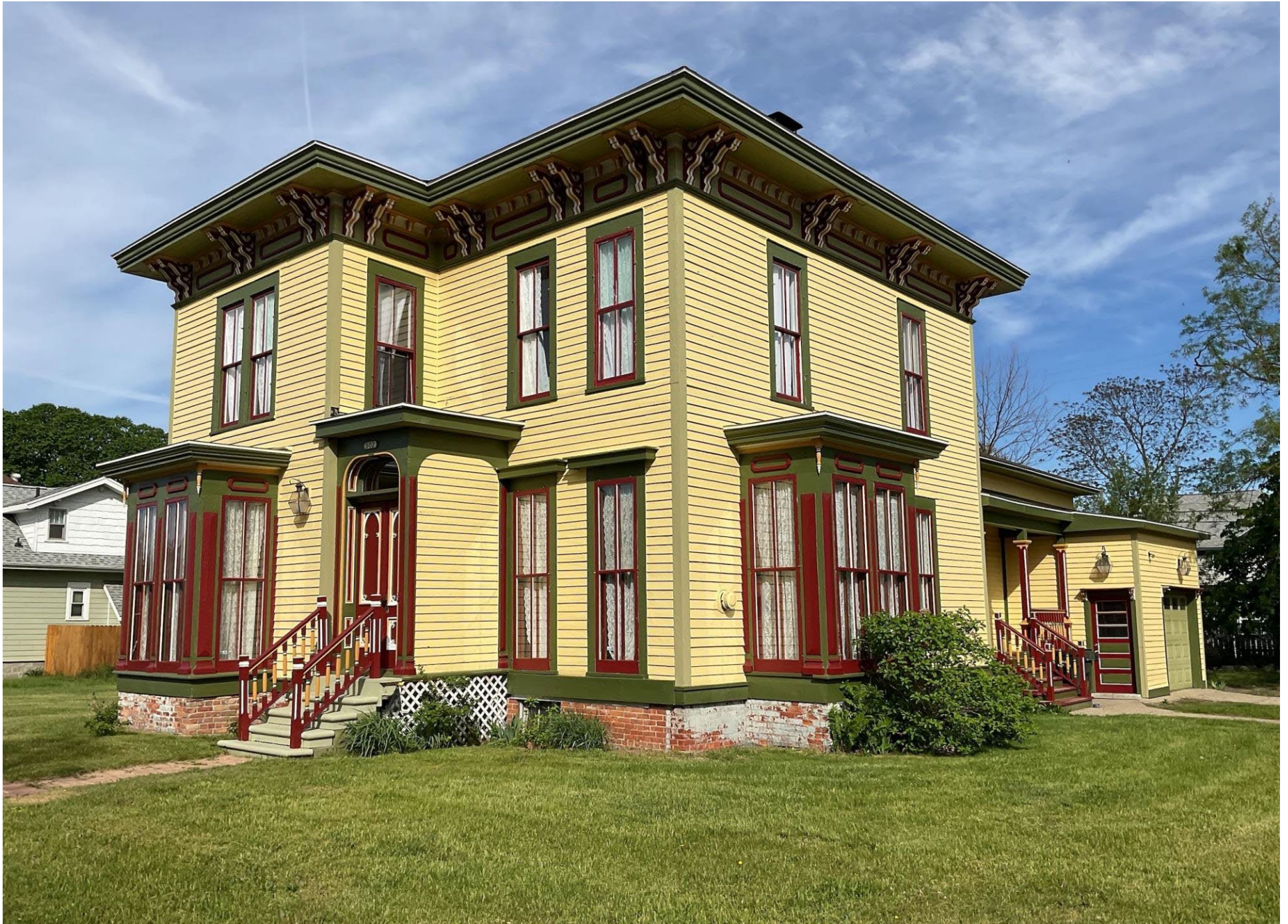
View of house from W. Webster Avenue, looking west (photo from May 2026, prior to the fire). Former rear addition/attached garage visible at right.
