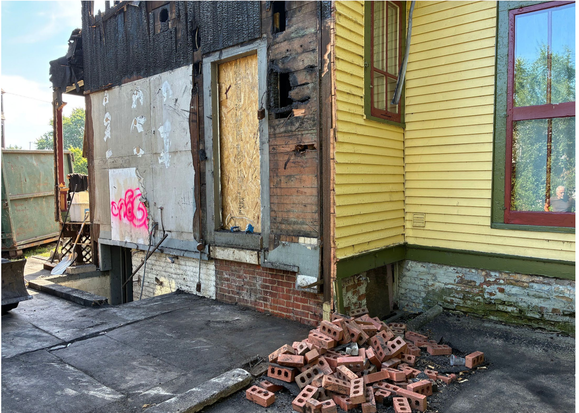
View of west (side) elevation after demolition.
