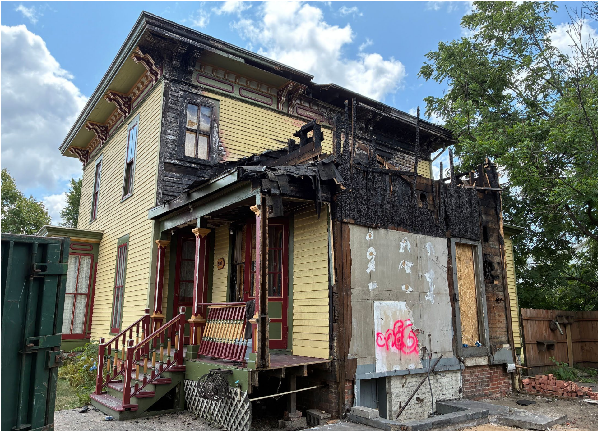
View of side porch and south (rear) elevation after demolition of garage.
