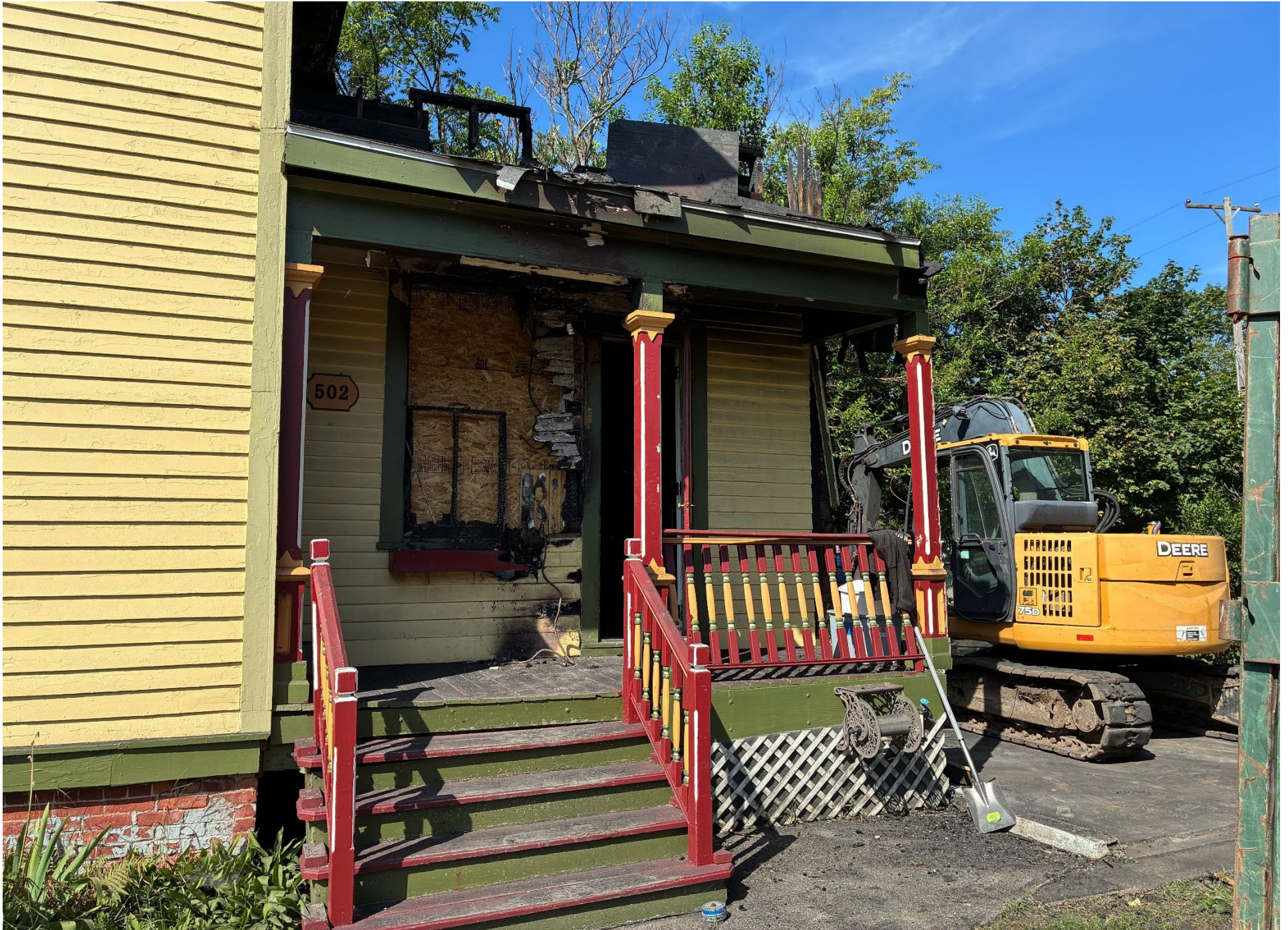
View of rear addition from 6 th Street after demolition.
