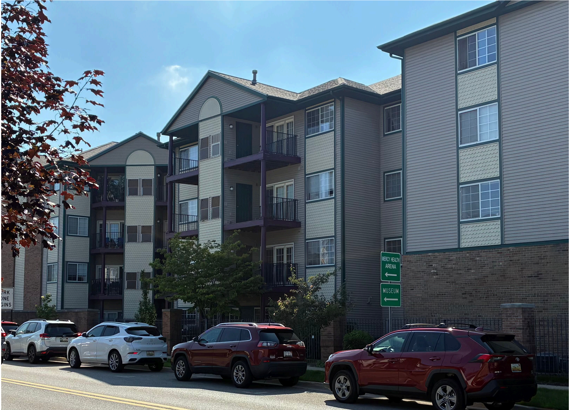
View of building from W. Muskegon Avenue, looking east; Stack 2 balconies facing proposed to be reconstructed are visible at center.
