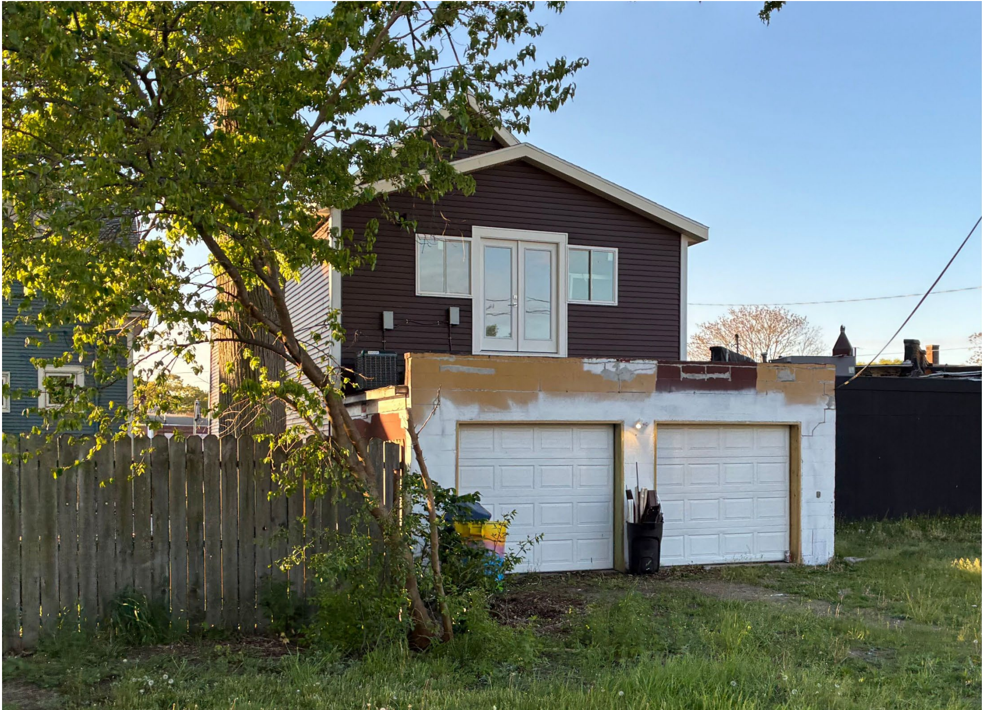
View of rear deck from rear alley, looking south; French doors (that replaced former slider door) visible.
