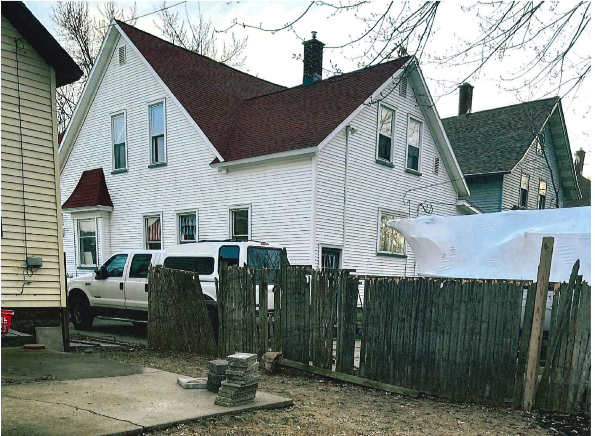
View of previous wood privacy fence (since removed) from back yard, looking southwest.
