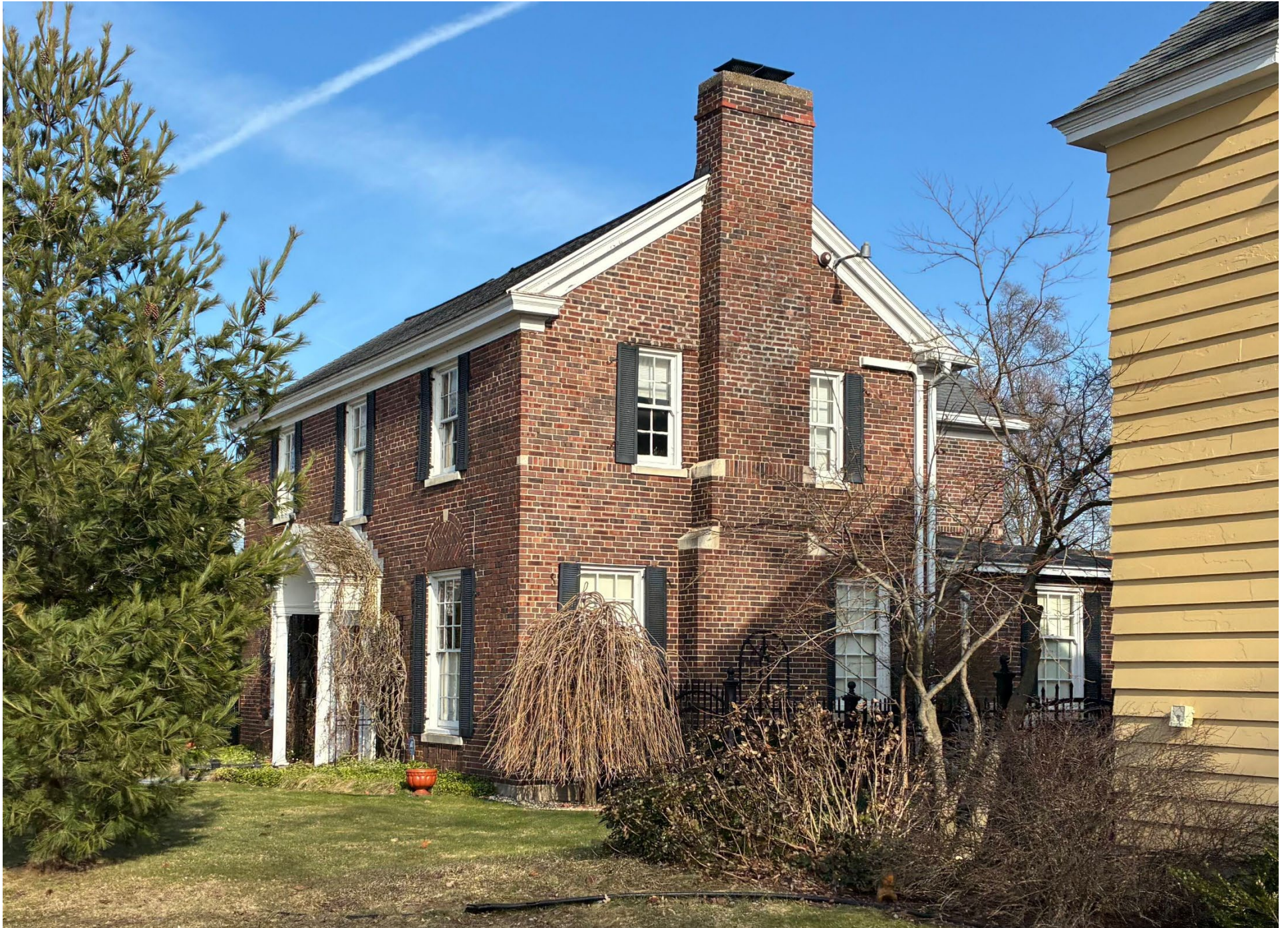
View from W. Webster Avenue, with rear addition visible at right.
