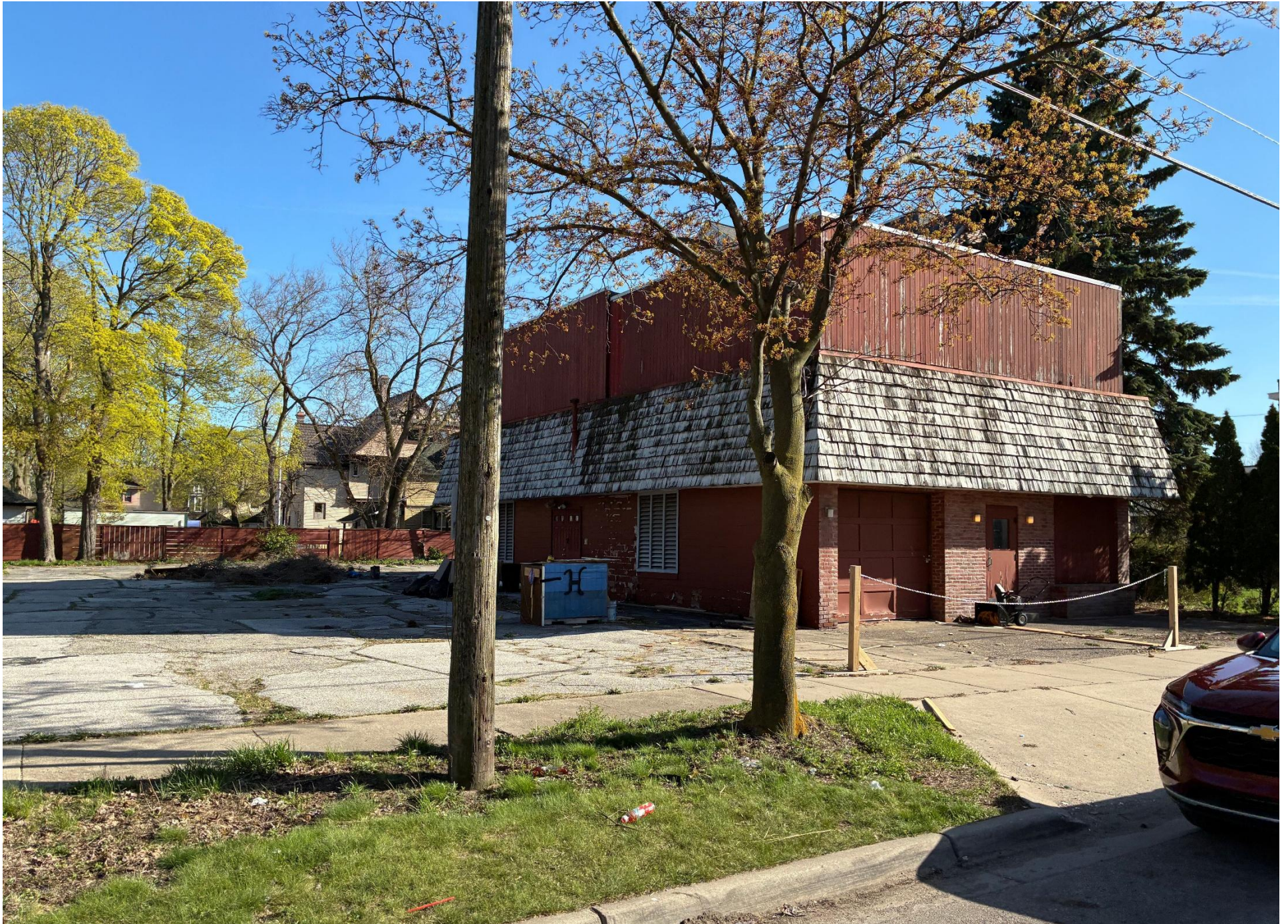
View of east (rear) elevation from Hartford Avenue, looking southwest.
