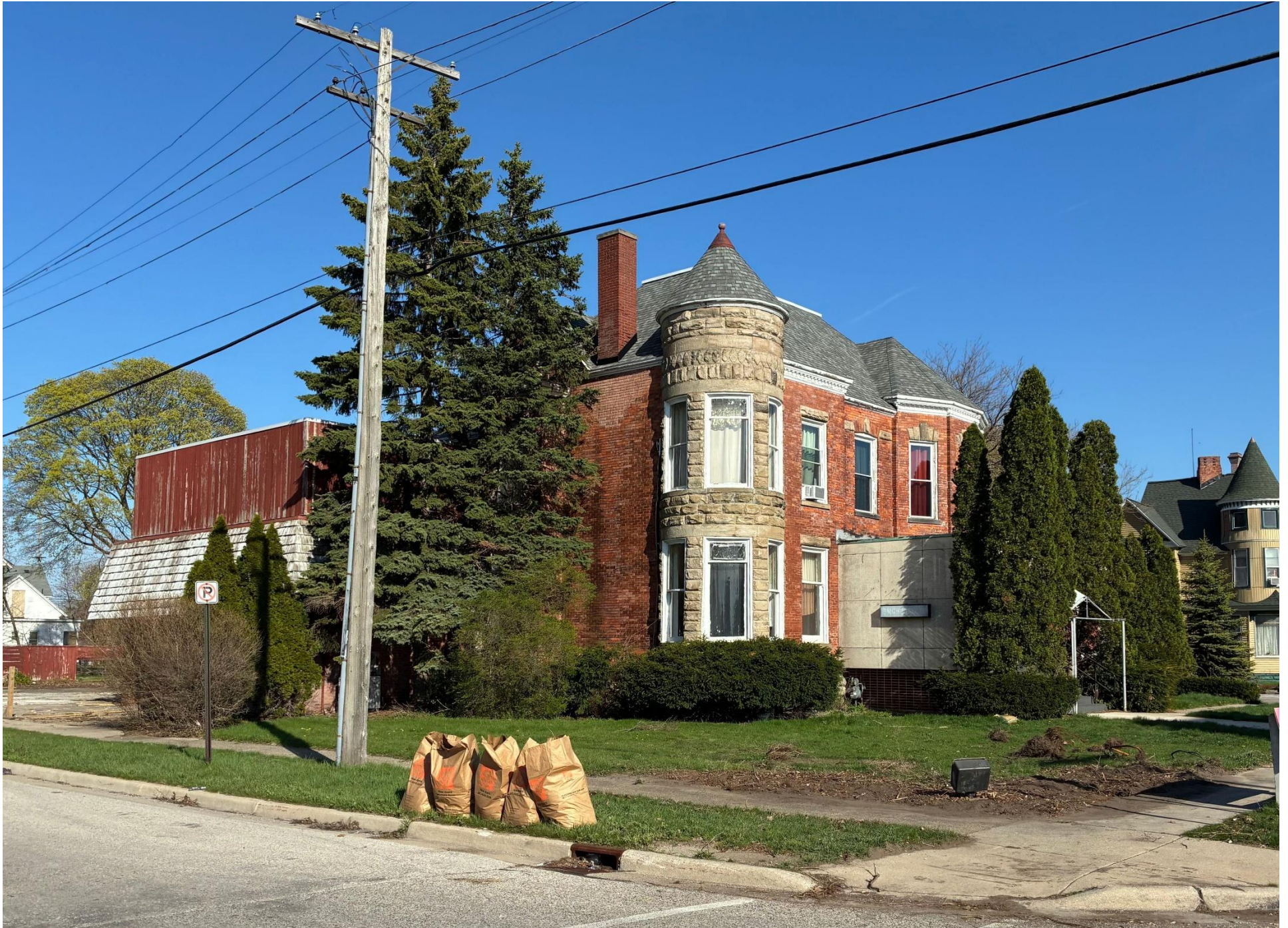
West (front) and north (side) elevations from Hartford Avenue, looking southeast.
