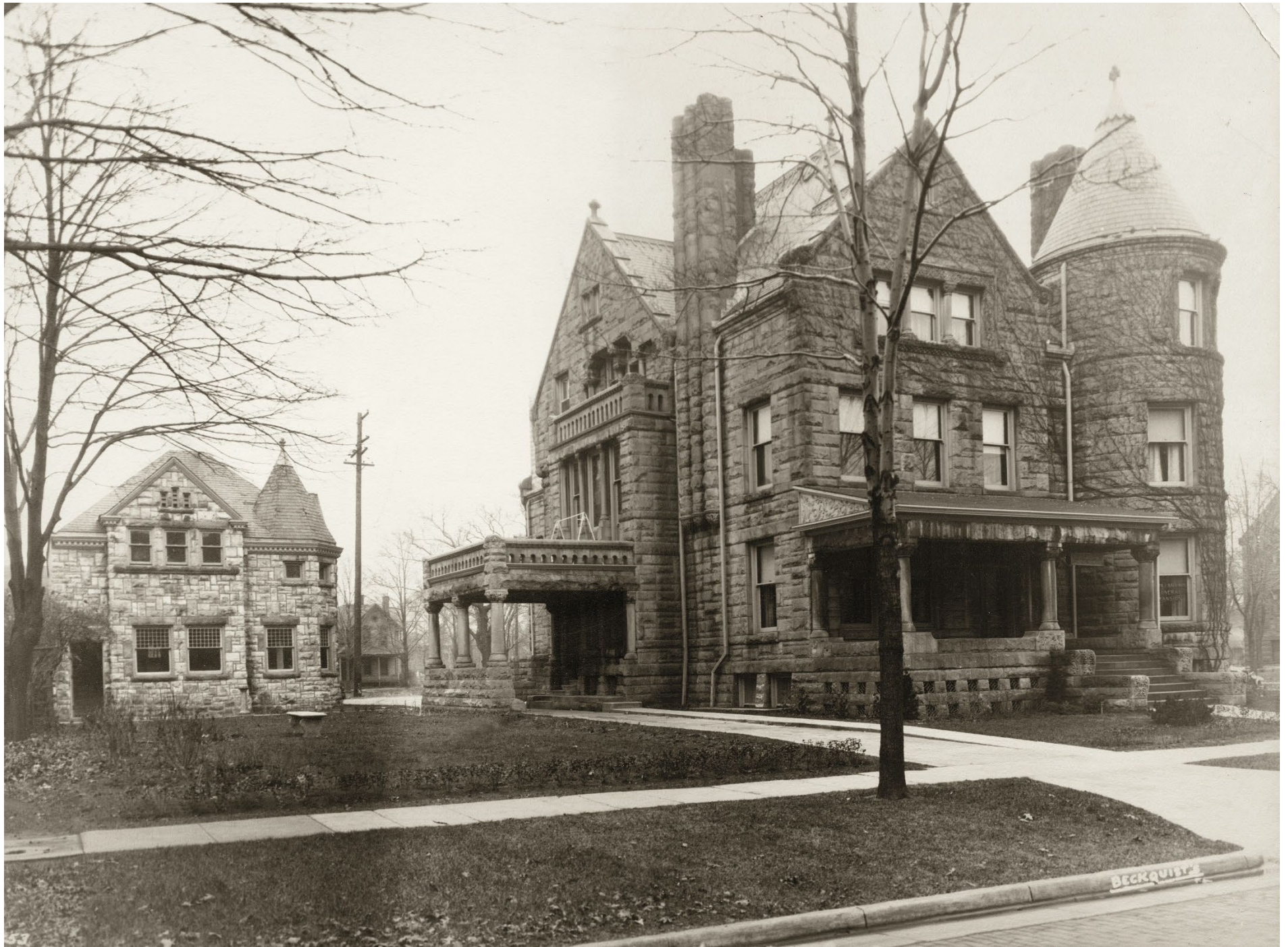
Similar view prior to demolition of the porte-cochère and chimney, and construction of the 1950s building addition (photo from 1929-1942).
