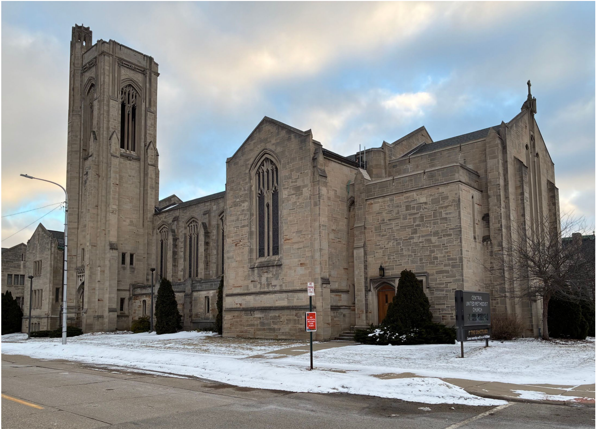
View of building from intersection of 2 nd Street and W. Webster Avenue, looking south.
