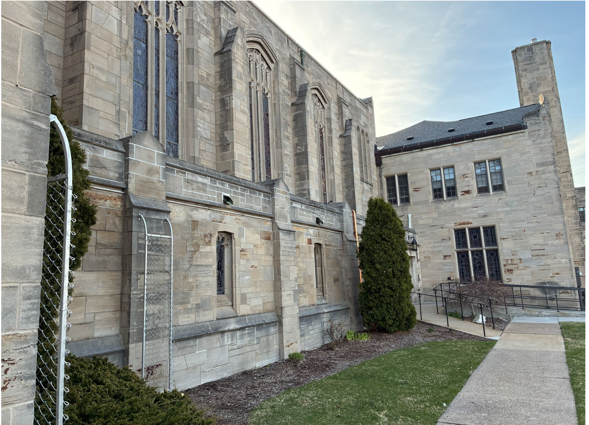
Proposed location for ground-mounted unit; copper downspout visible is similar to proposed appearance of copper pipe containing coolant lines.
