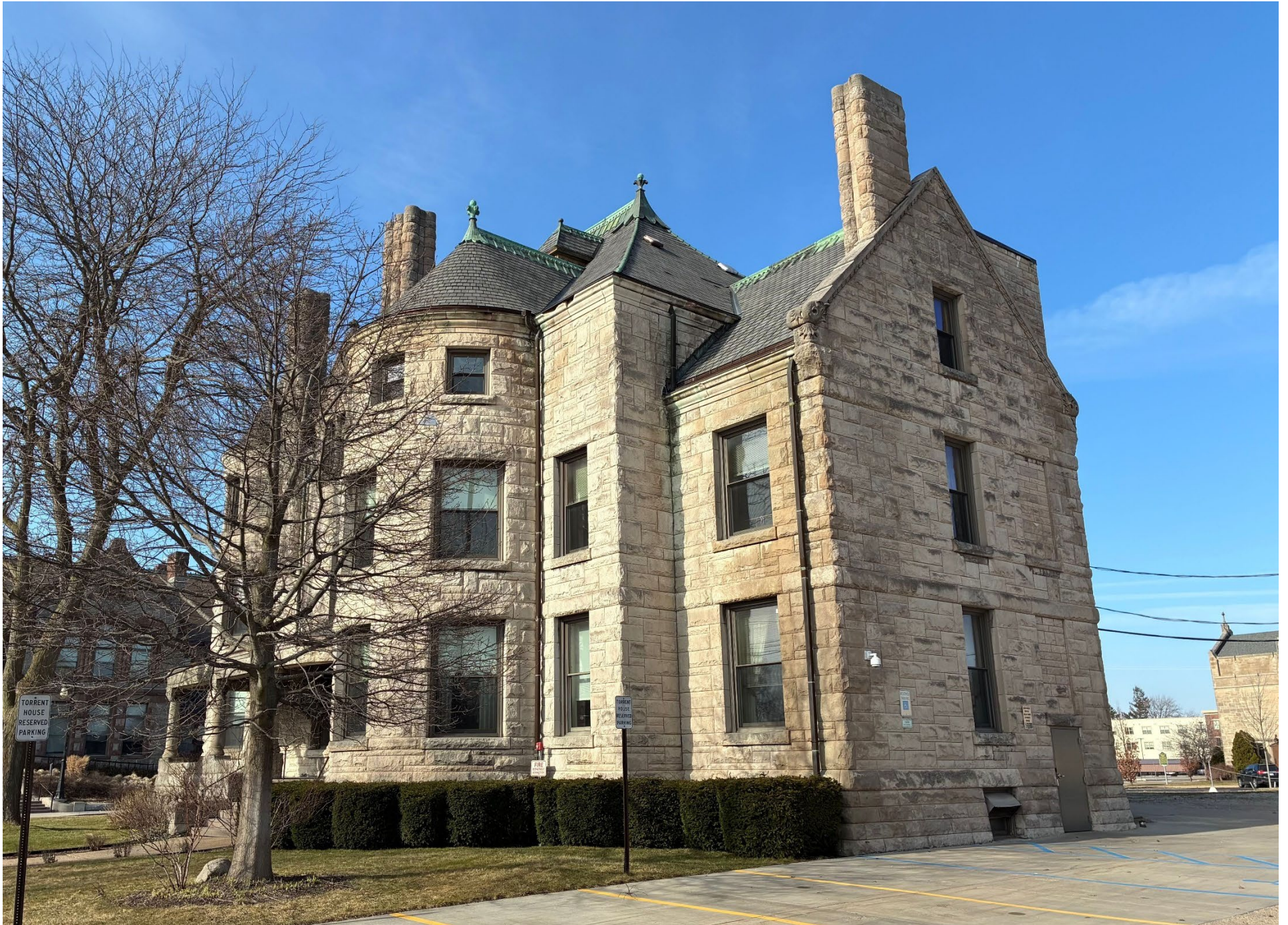
View of east (rear) and south (facing 3 rd Street) elevations from 3 rd Street, looking northeast.
