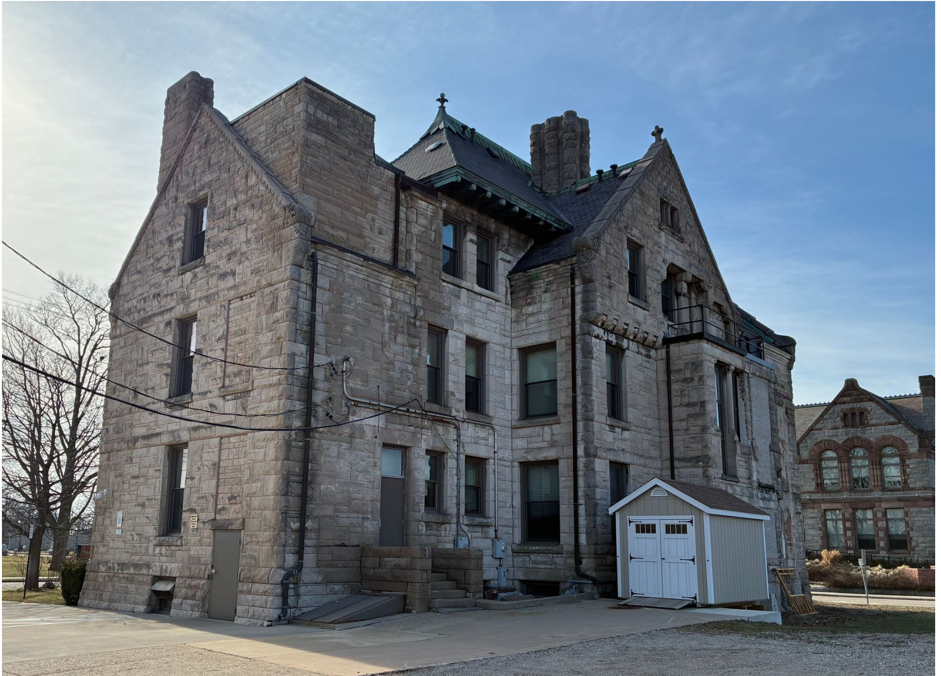
View of the east (rear) and north (side) elevations, looking northwest.
