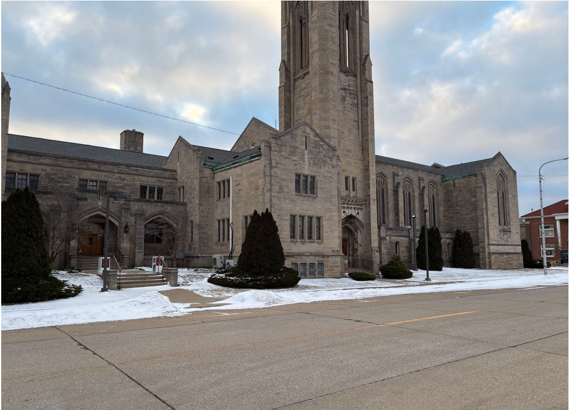
View of building from 2 nd Street, looking west, with existing ground-mounted units visible at center.
