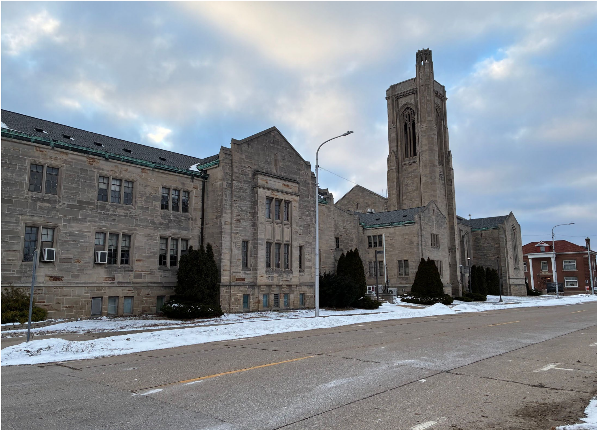
View of building from 2 nd Street, looking west.
