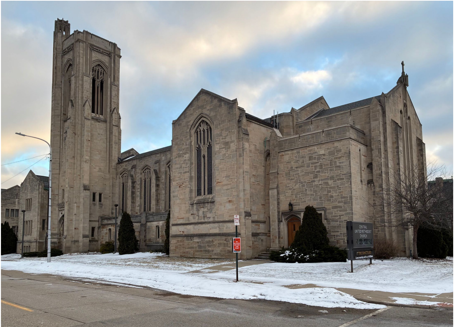
View of building from intersection of 2 nd Street and W. Webster Avenue, looking south.
