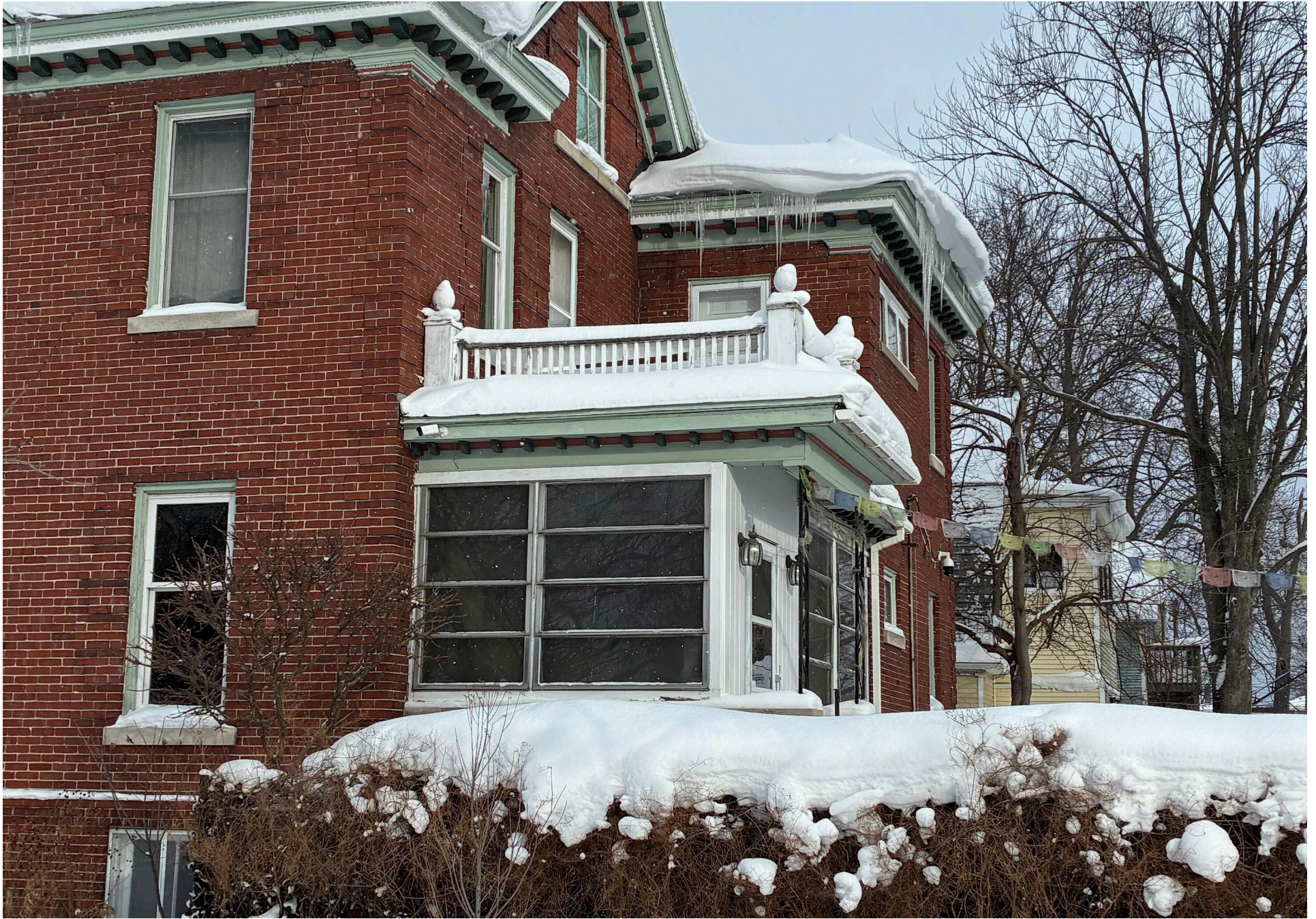
View of rear porch from E. Forest Avenue, looking north.
