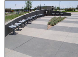
COLORLED CONCRETE PAVING BANDS
