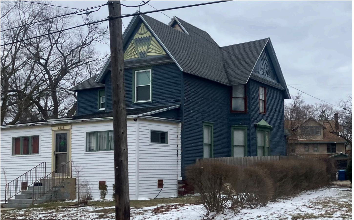
View of south (side) and west (front) elevations from Peck Street, looking northeast; two windows in bay proposed to be replaced on south elevation visible at right (photo from March 2025).
