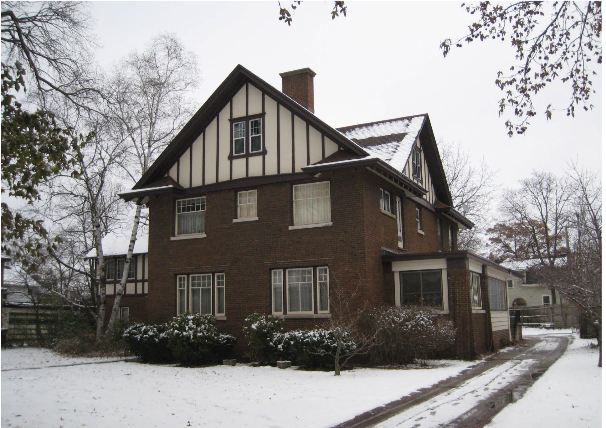
View of west (front) and south (side) elevations from Jefferson Street, looking northeast (photo from December 2019).
