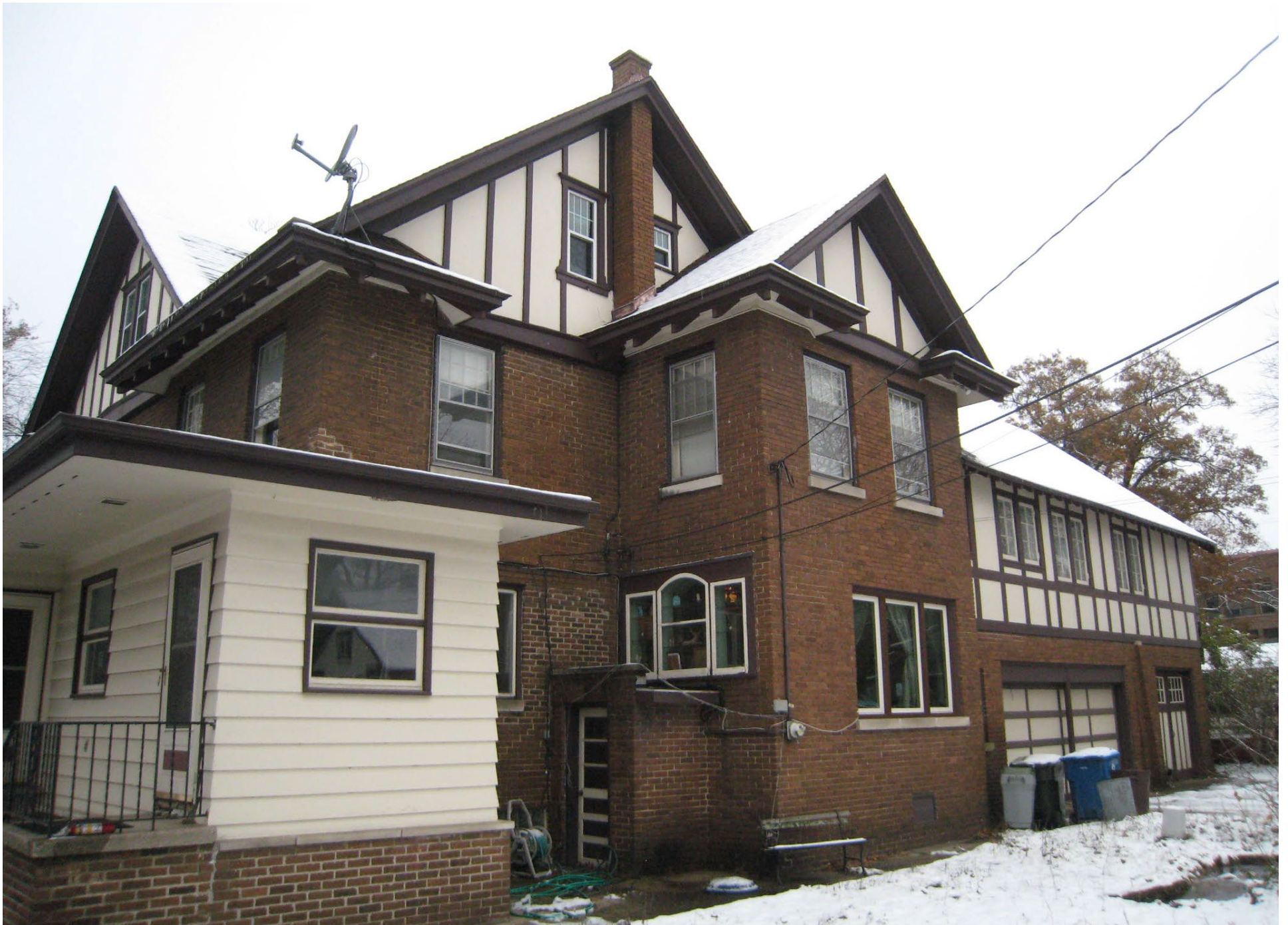
View of south (side) and east (rear) elevations from rear yard with two doors proposed to be replaced visible at left (photo from December 2019).
