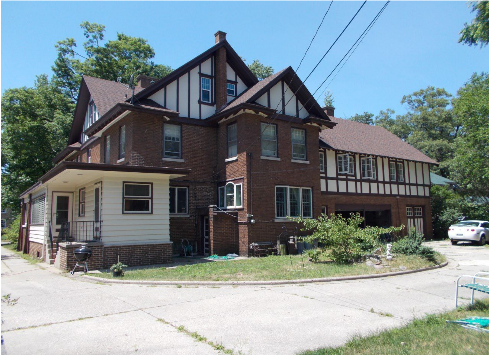
View of south (side) and east (rear) elevations from rear yard with two doors proposed to be replaced visible at left (photo from June 2017).
