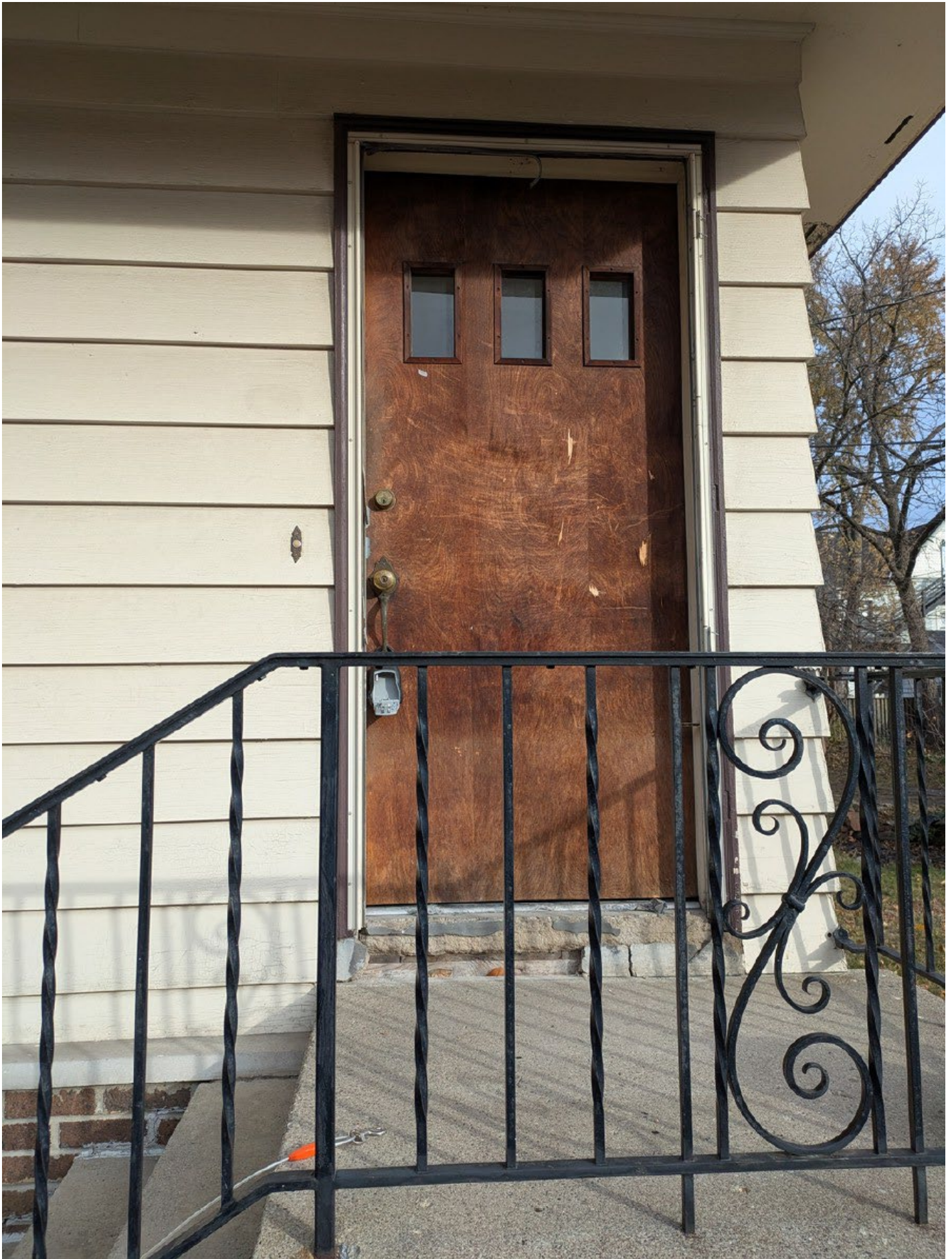
View of existing door proposed to be replaced on south-facing wall.
