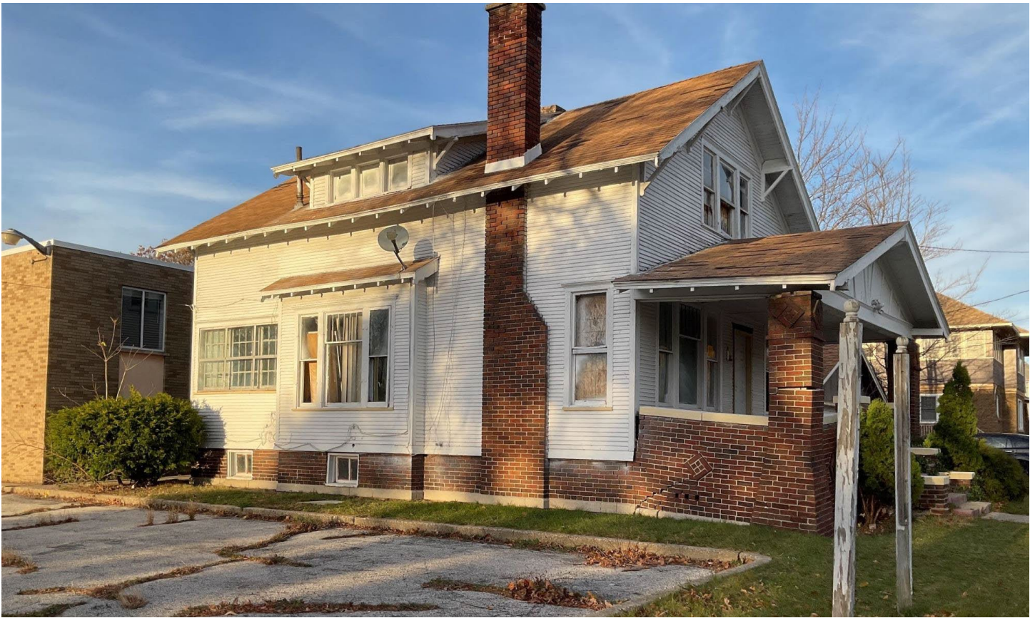
View of west (side) elevation (photo from November 2022).
