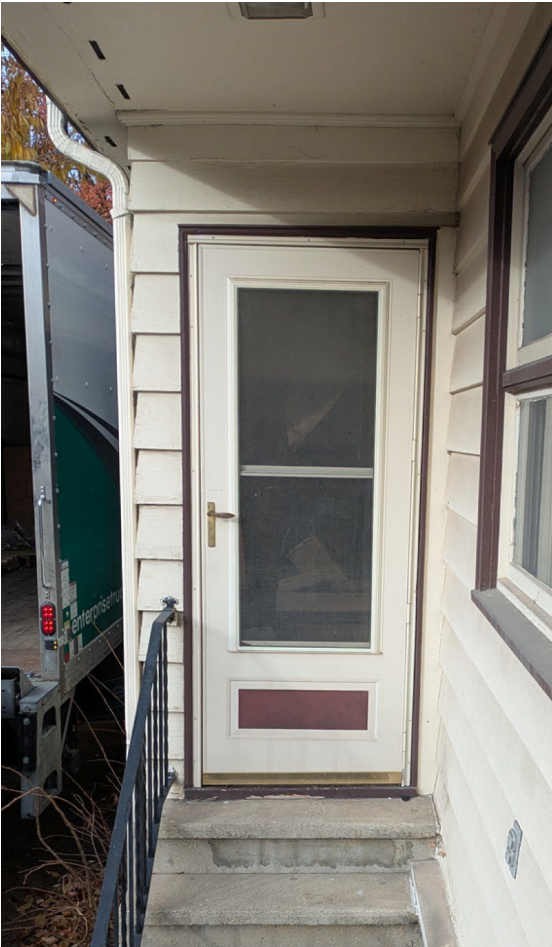
View of existing door proposed to be replaced on east-facing wall.
