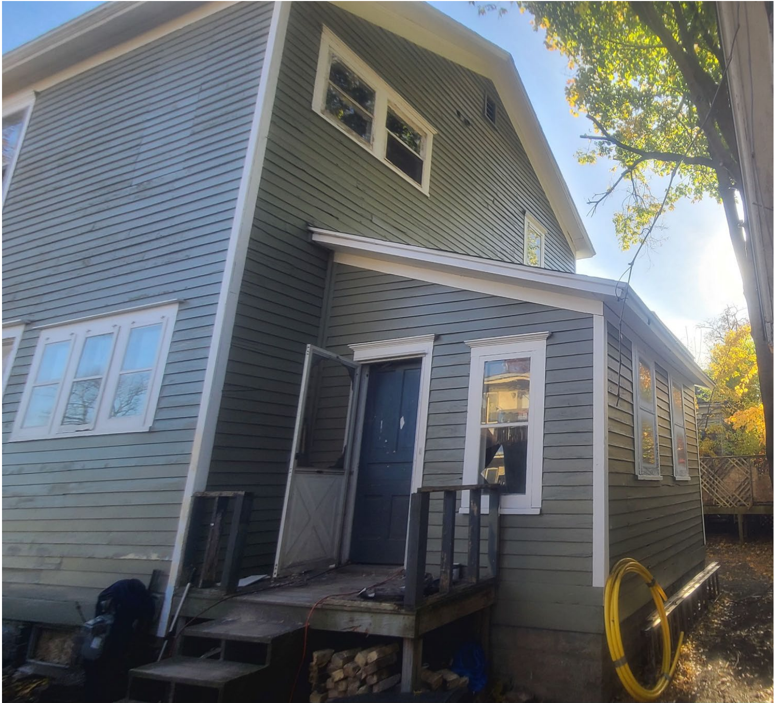
View of west (rear) elevation from rear yard.
