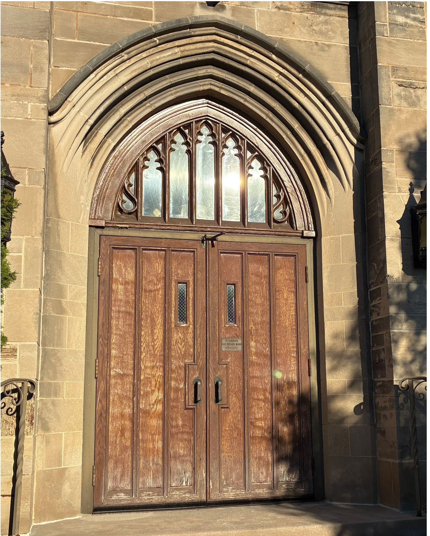
Entry doors on south elevation proposed to be replaced
