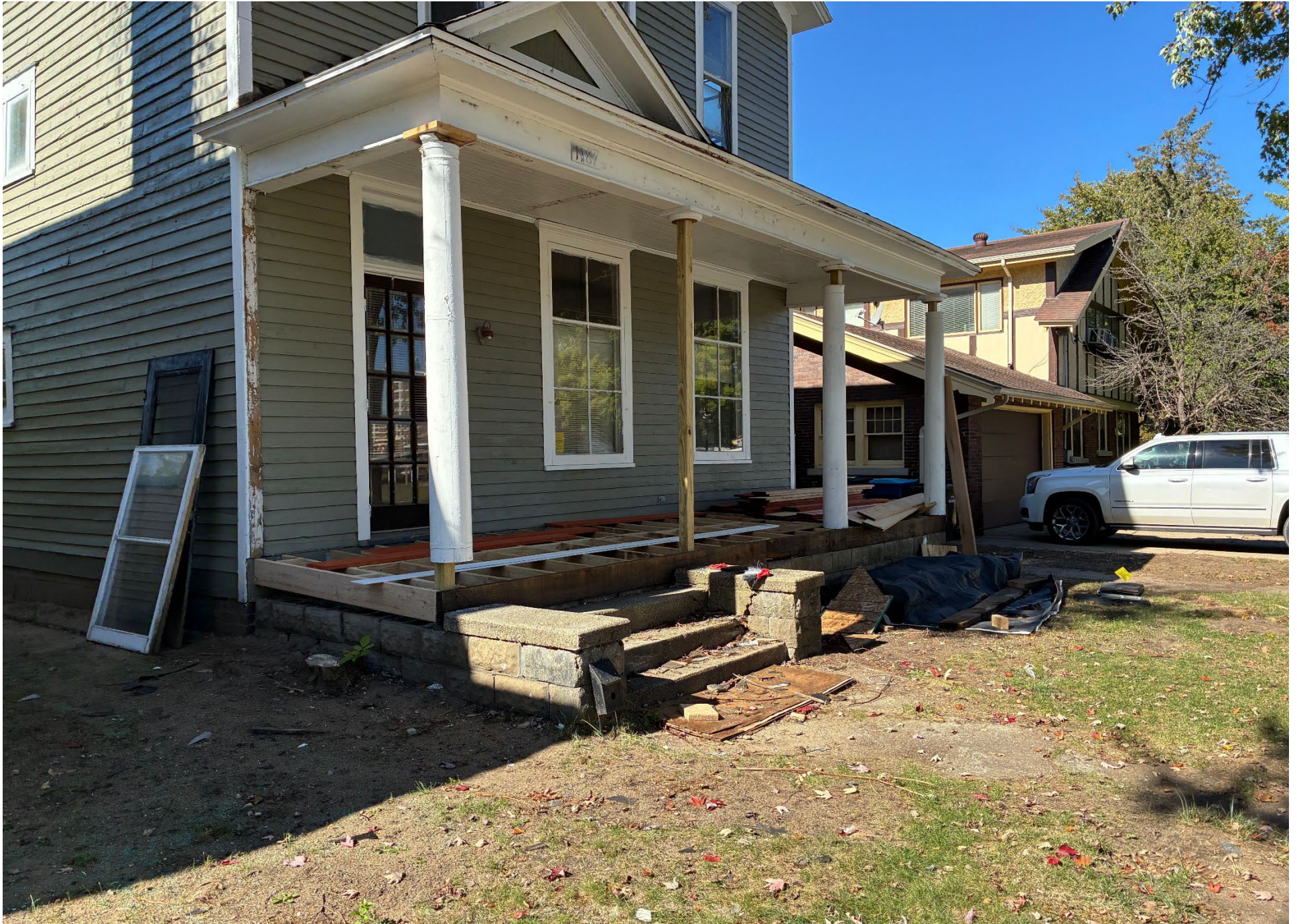
View of front porch during construction
