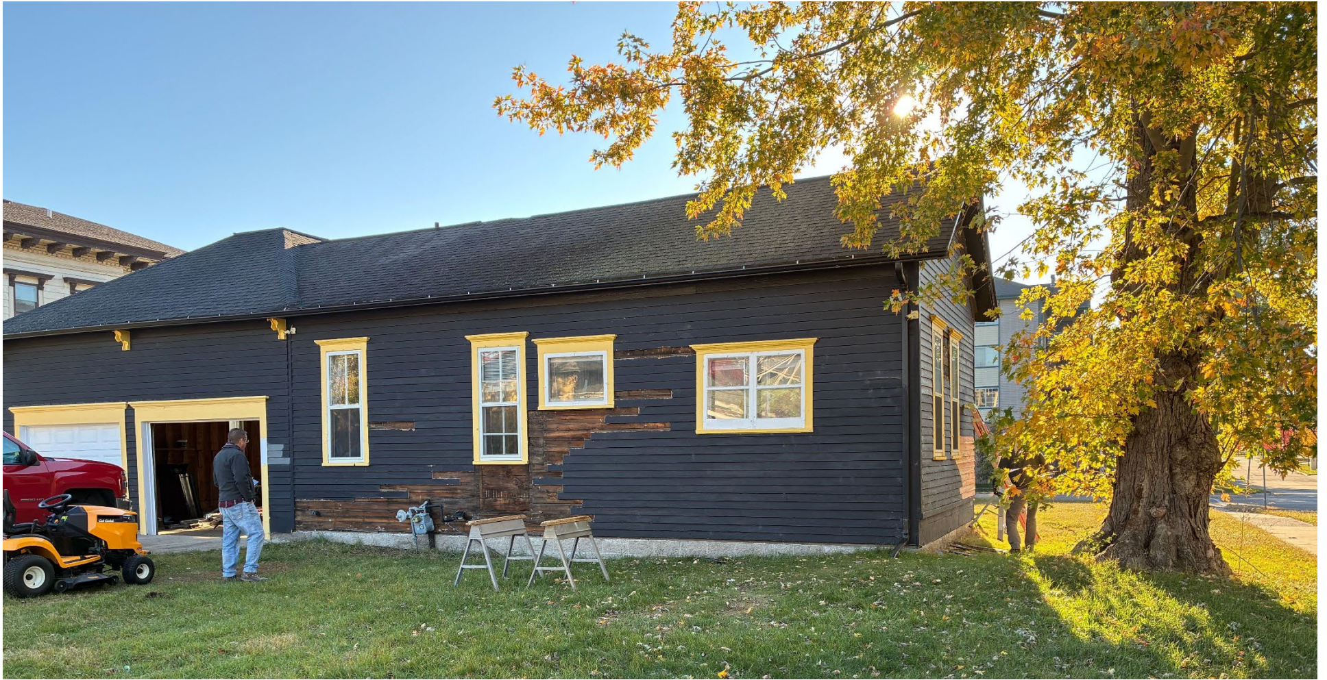
View of north (rear) elevation from alley with window second from right to be removed and window third from right to be reduced in size to 30"x36"
