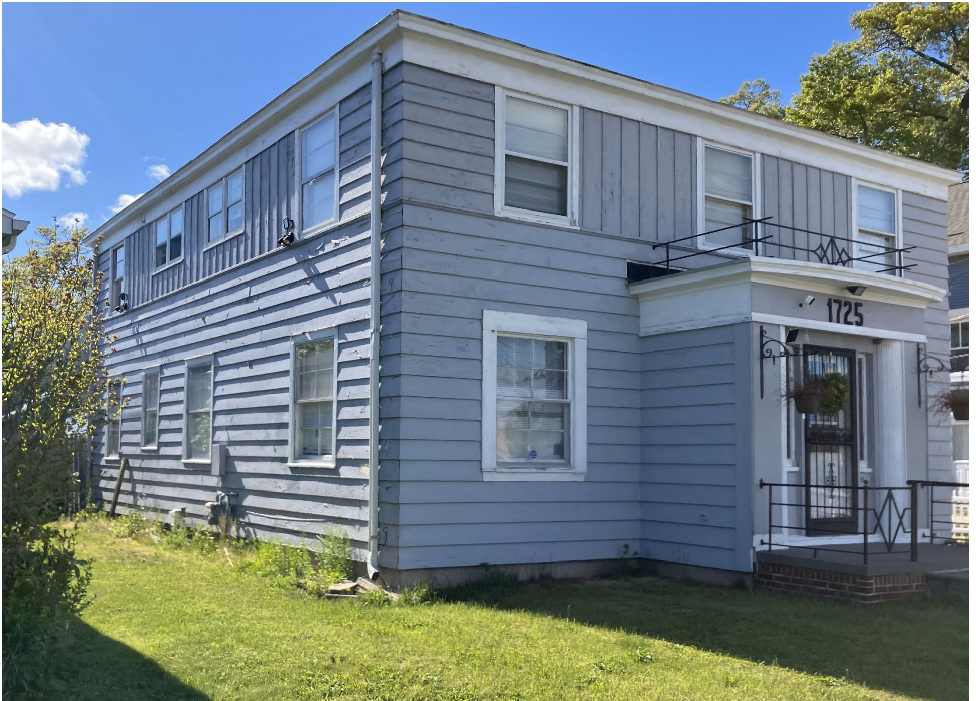
View of east (front) and south (side) elevations from Peck Street, looking northwest (photo from May 2025)
