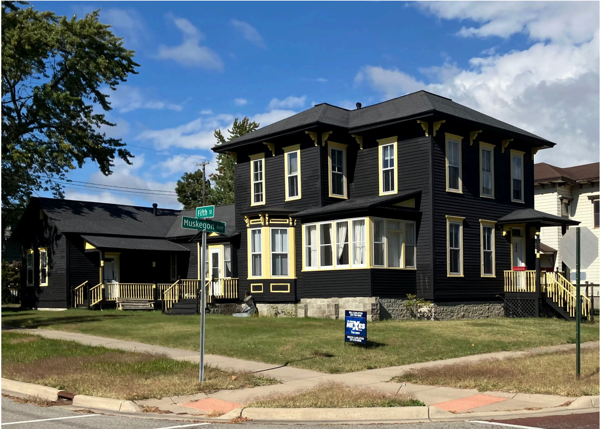
View of west (side) and south (front) elevations from the corner of W. Muskegon Avenue and 5 th Street
