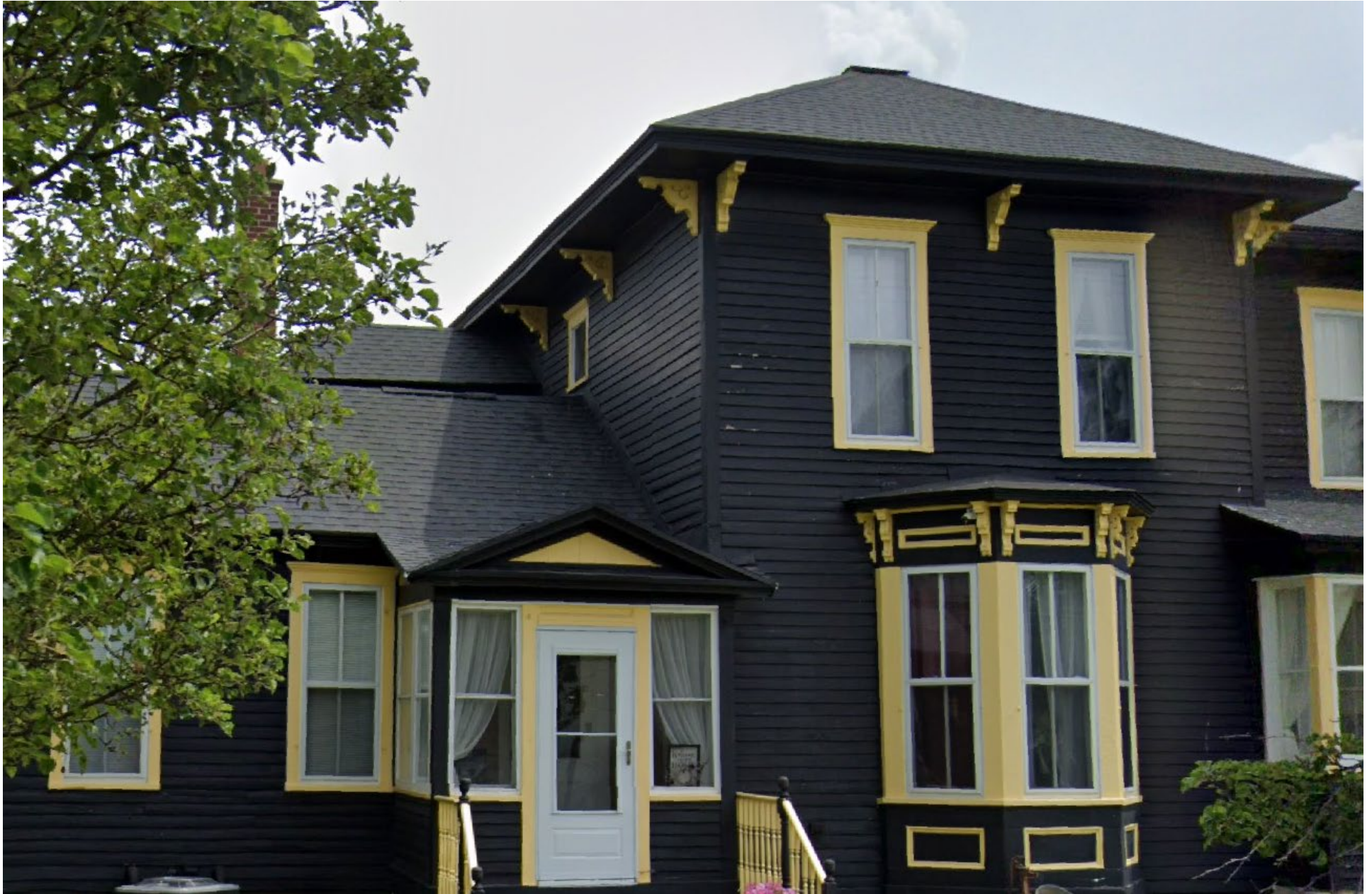
Small, second story window on north (rear) elevation to be removed
