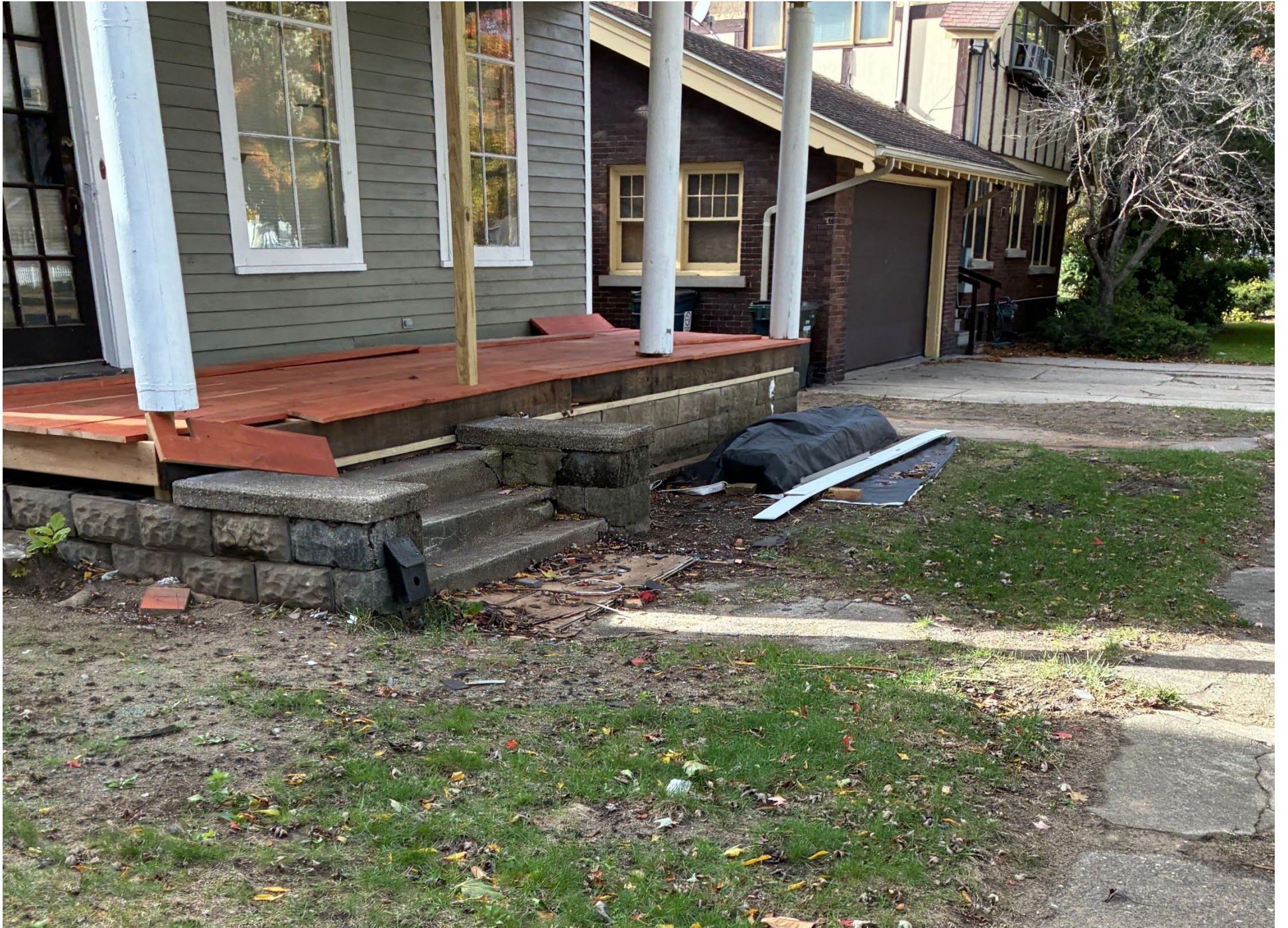
Front porch during construction with proposed deck boards
