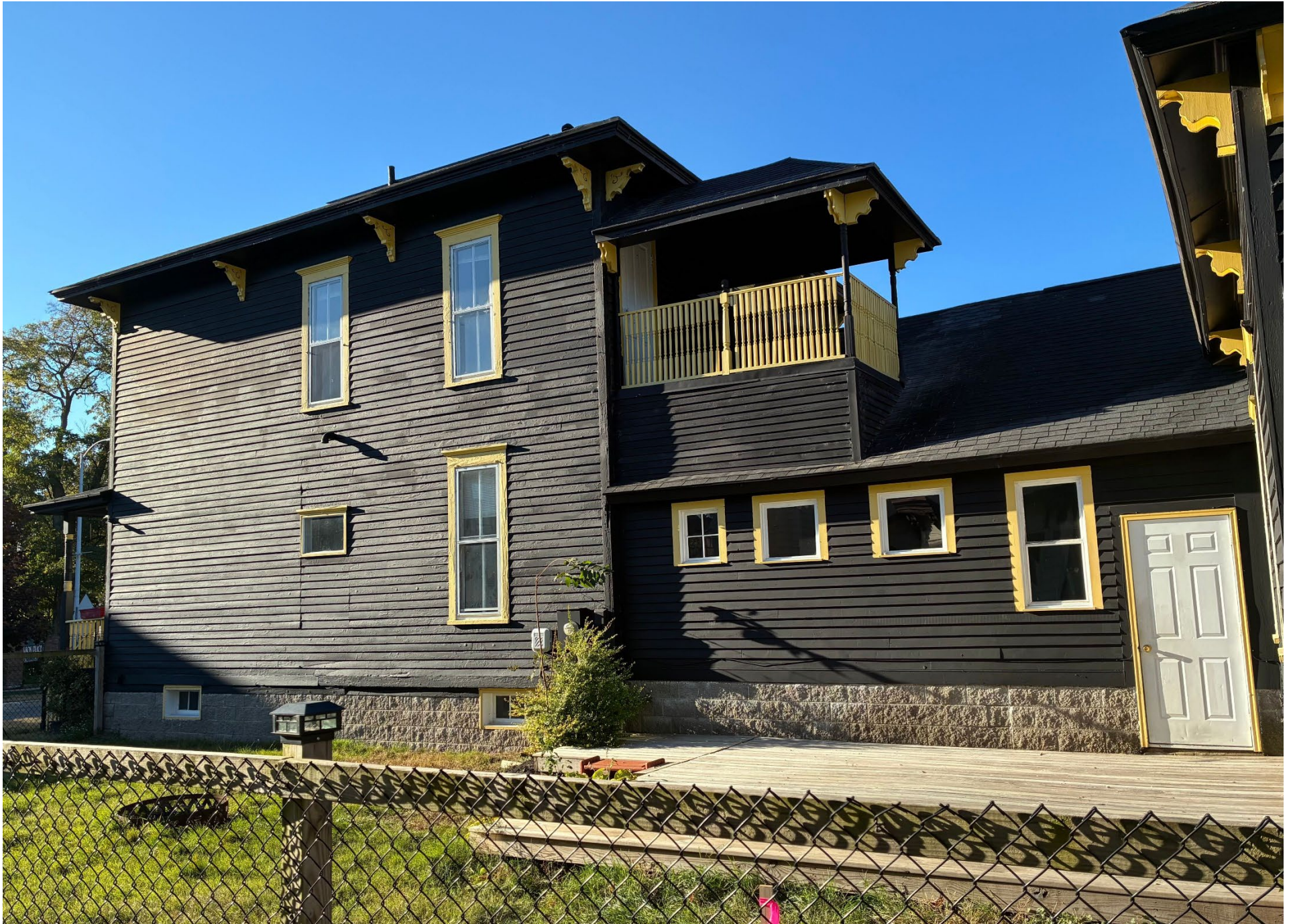
View of east (side) elevation
