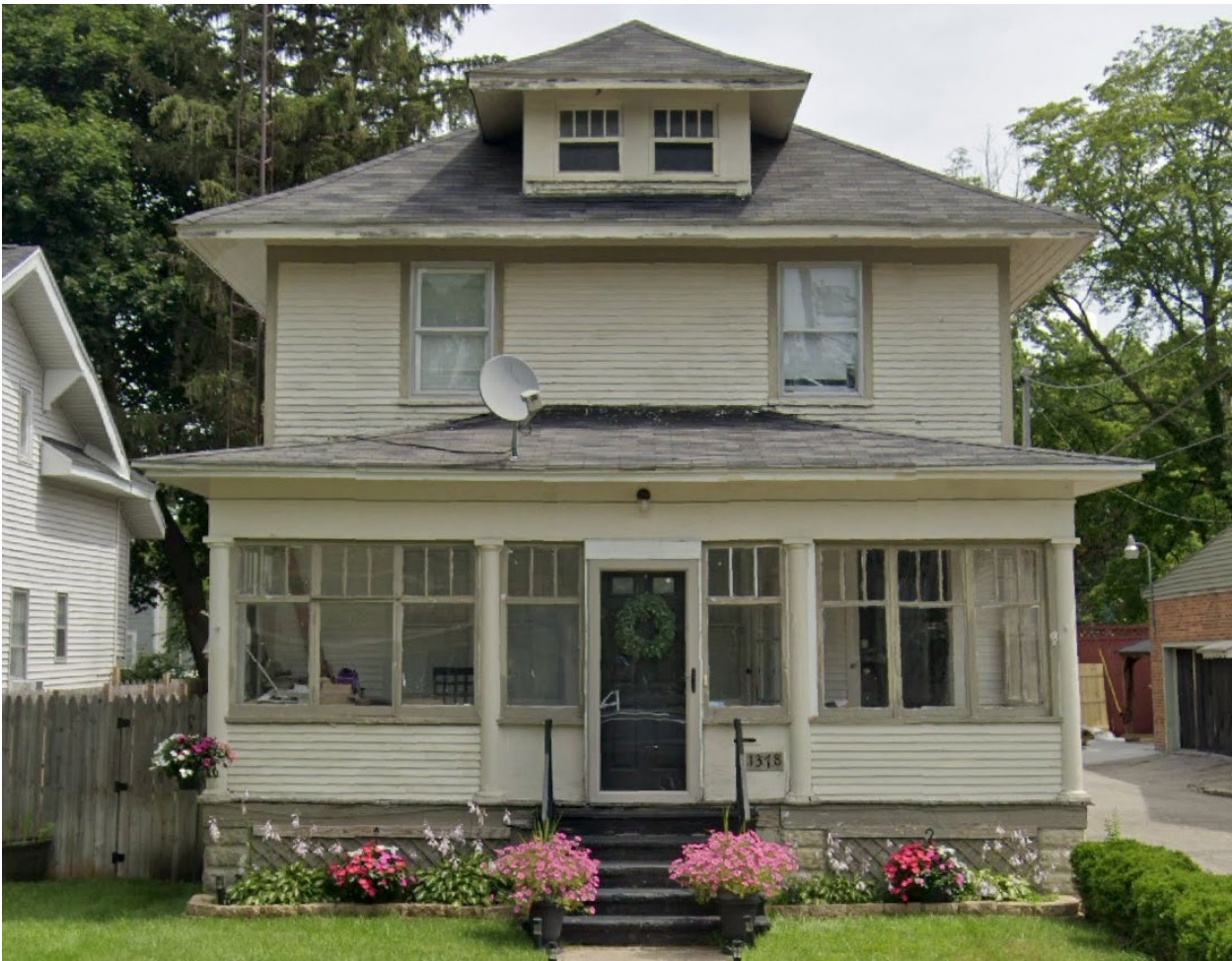
View of west elevation from 5 th Street (photo from July, 2024)
