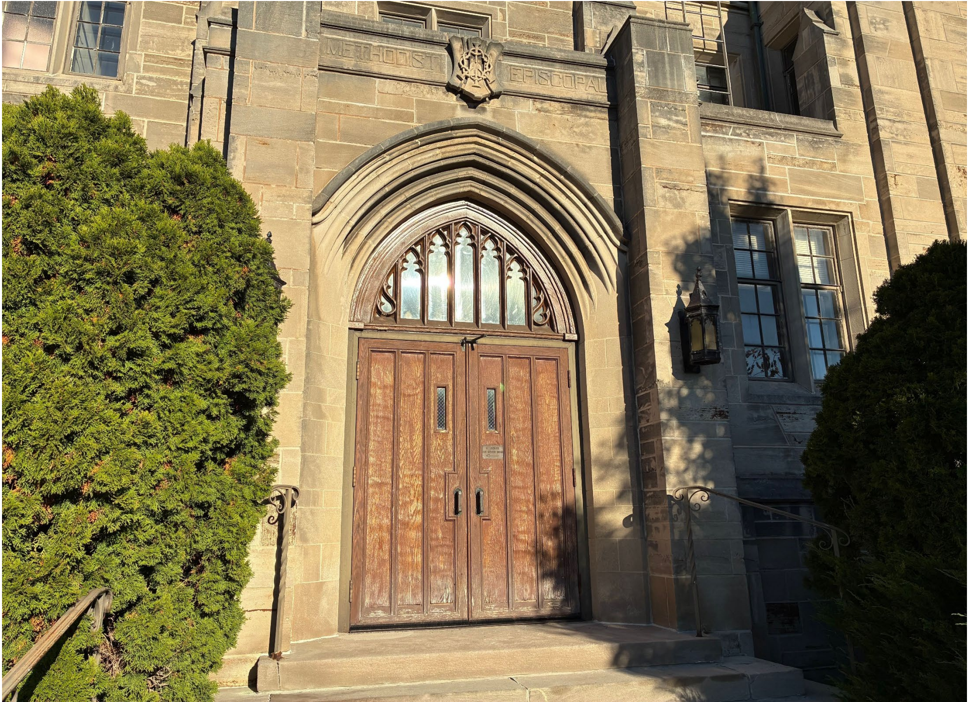
Entry doors on south elevation proposed to be replaced
