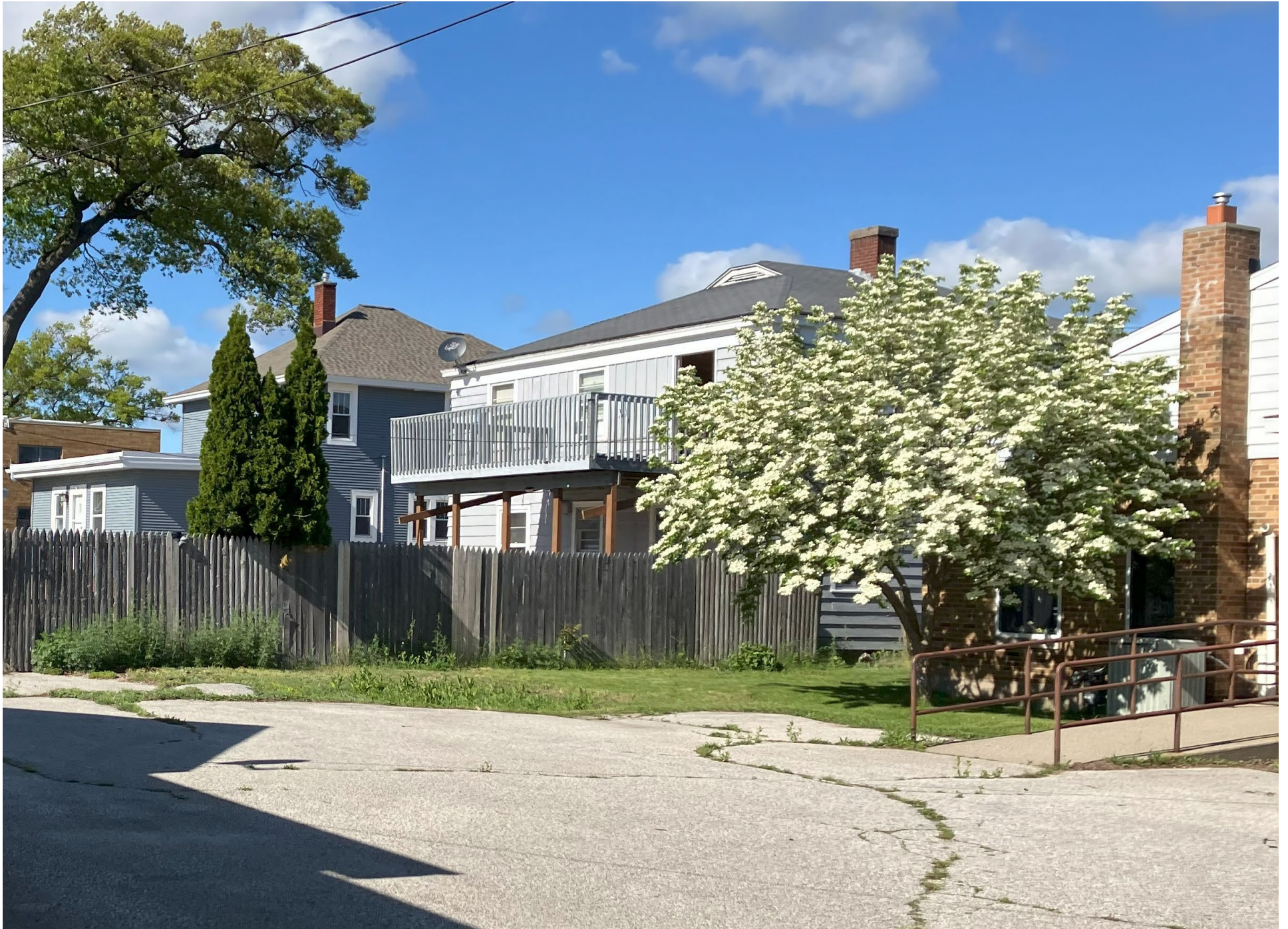
View of west (rear) elevation from Larch Avenue, looking northeast (photo from May 2025)
