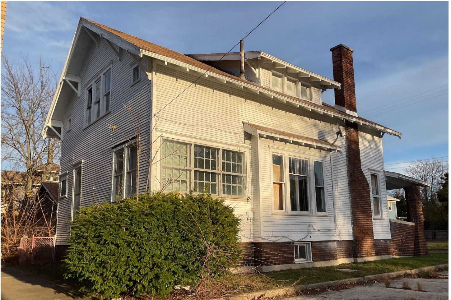
View of west (side) and north (rear) elevation (photo from November 2022).
