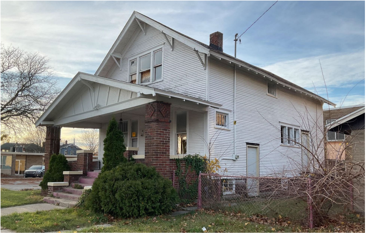
View of east (side) and south (front) elevations from Delaware (photo from November 2022).
