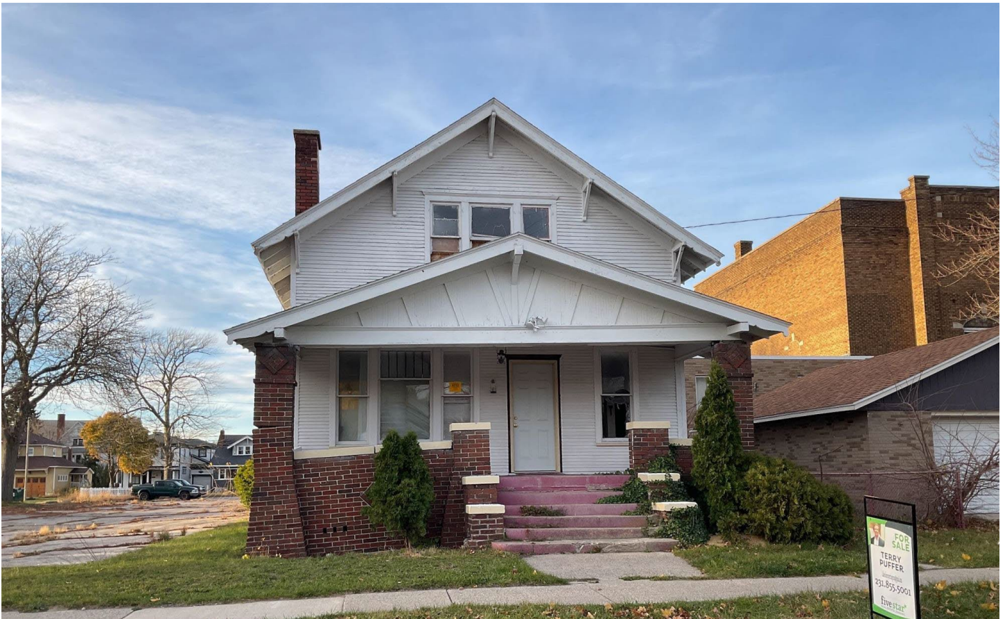
View of south (front) elevation and damaged porch (photo from November 2022).
