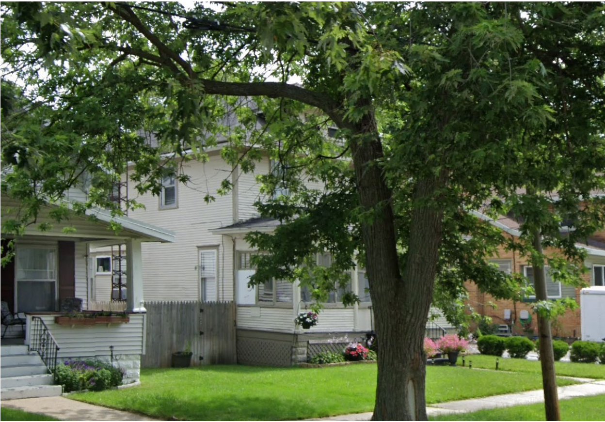
View of north (side) elevation from 5 th Street (photo from July, 2024)
