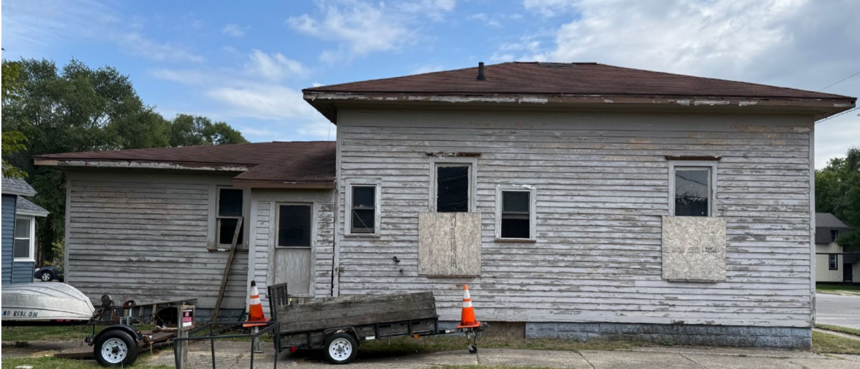
North elevation showing two small windows on main body of house to be removed; new 30"x72" window to be installed at far left
