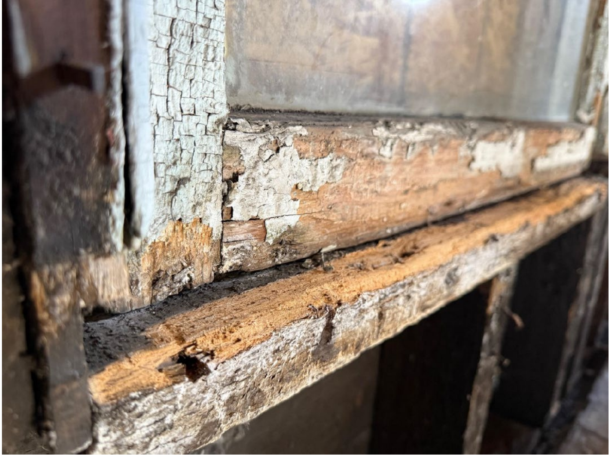
Detail photo of existing window sash
