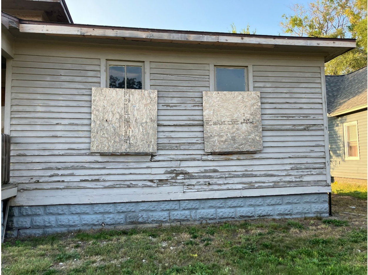
Two windows on south elevation to be replaced
