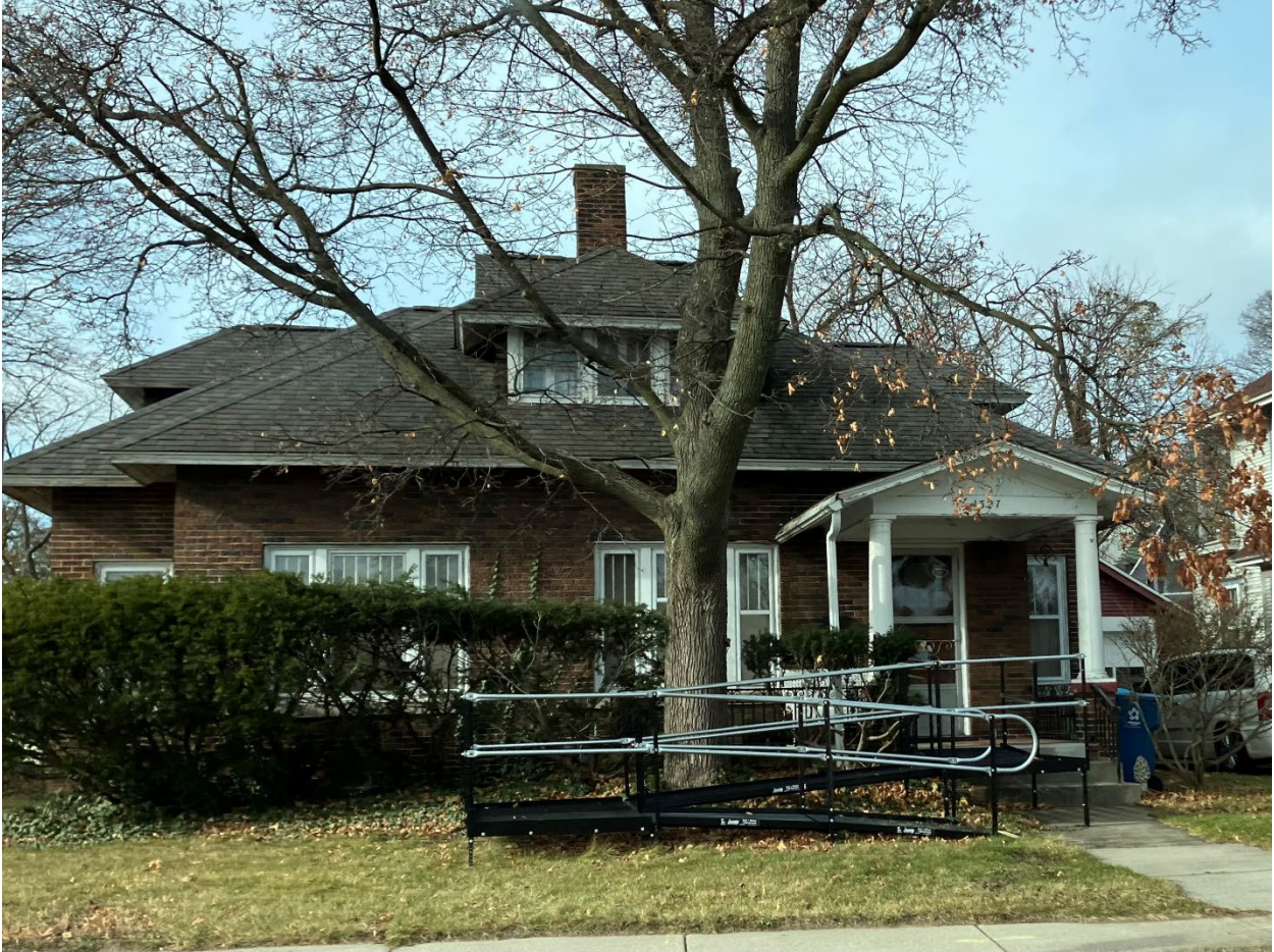
Ramp installed on Jefferson Street
