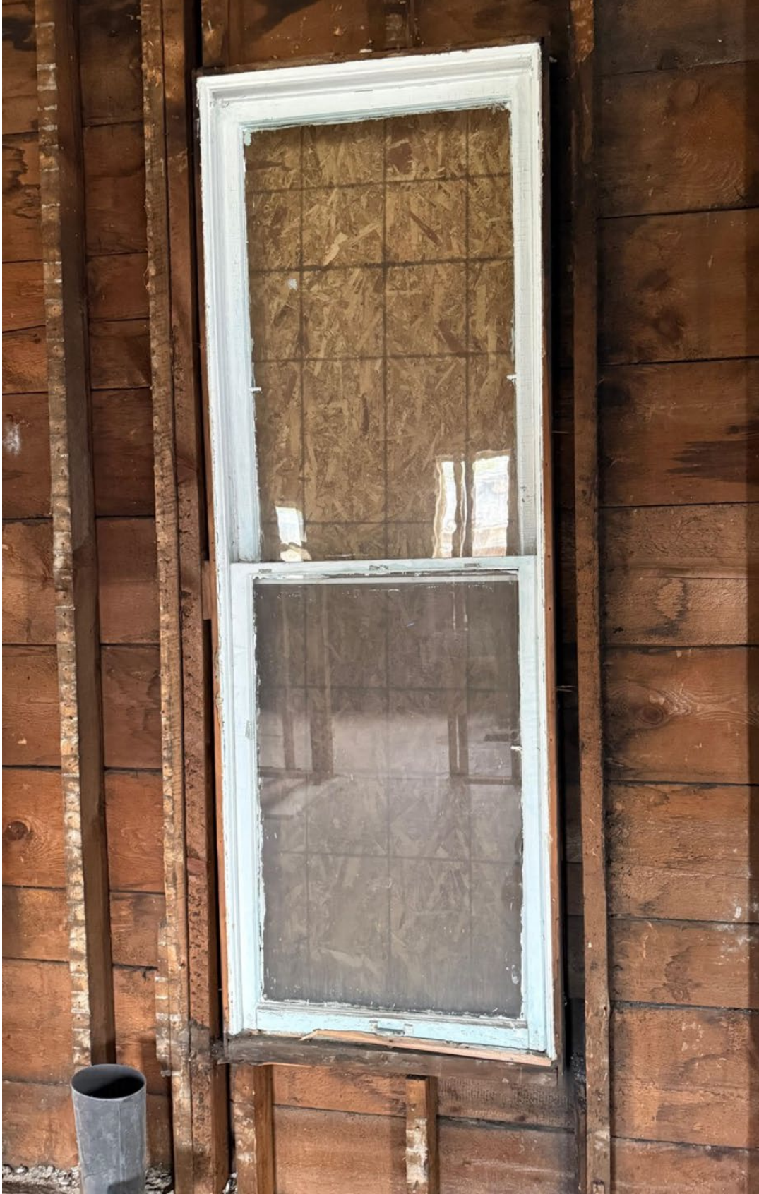
Photo of existing window viewed from the interior
