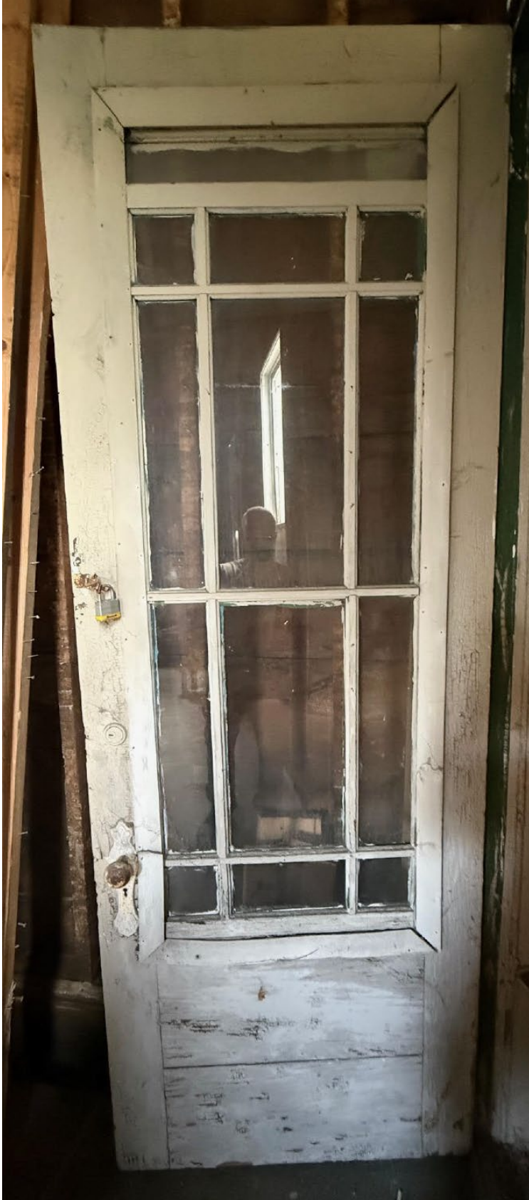
Existing 32"x90" front door and proposed 36"x96" fiberglass replacement door
