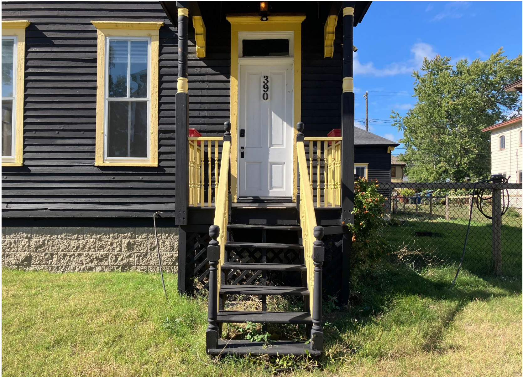
View of front porch staircase
