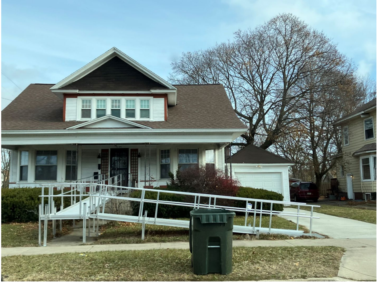
Ramp installed on Terrace Street
