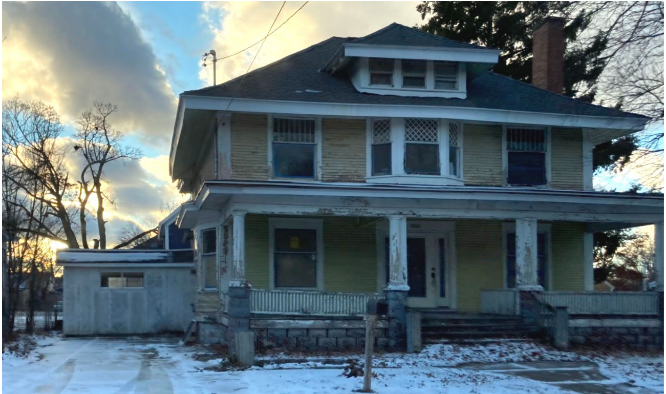
View of house from Ransom Street; existing house addition (built between 1911 and 1950) proposed to be converted to garage visible at left
