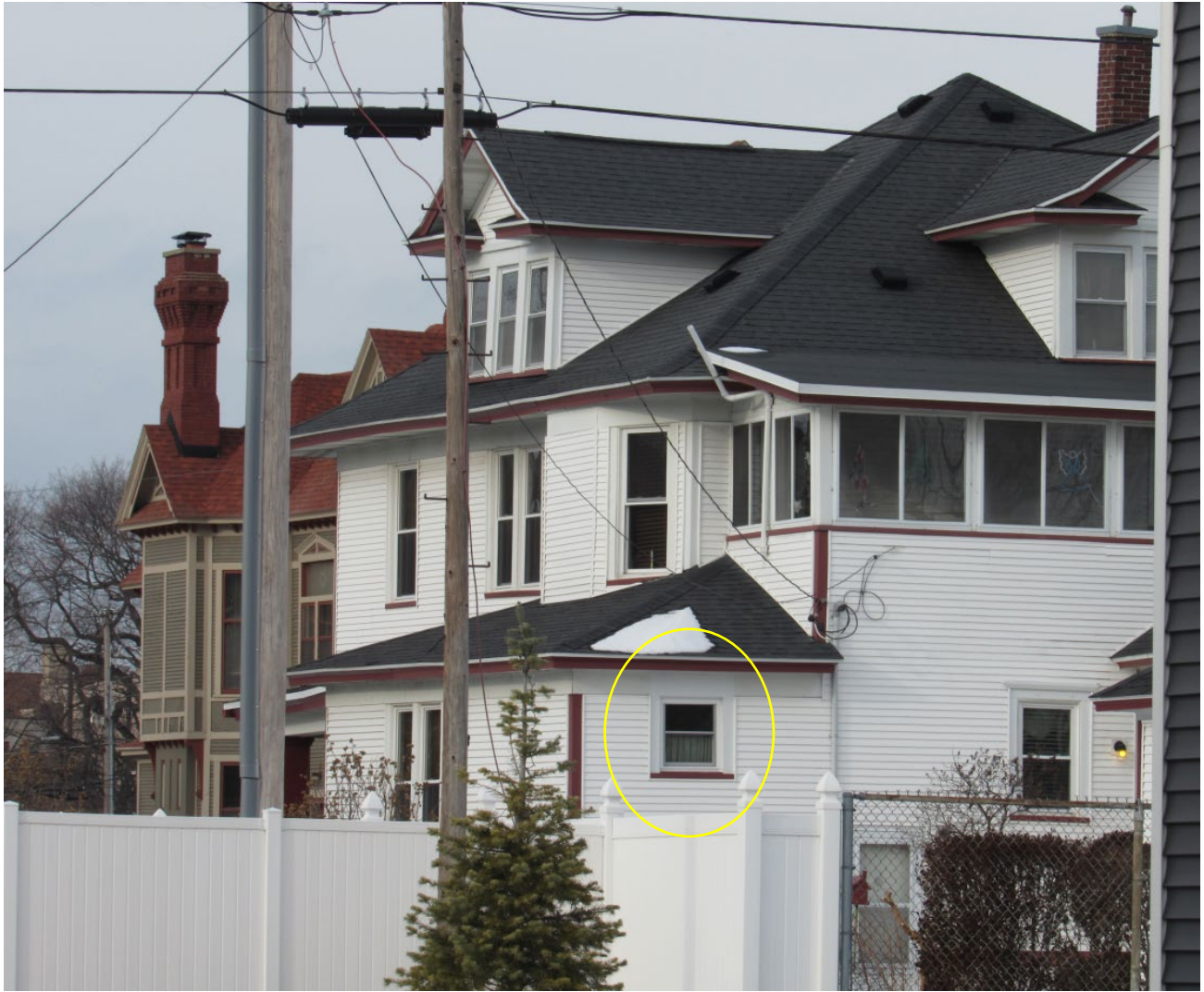
Rear of house viewed from Monroe Avenue. Third replacement window circled.
