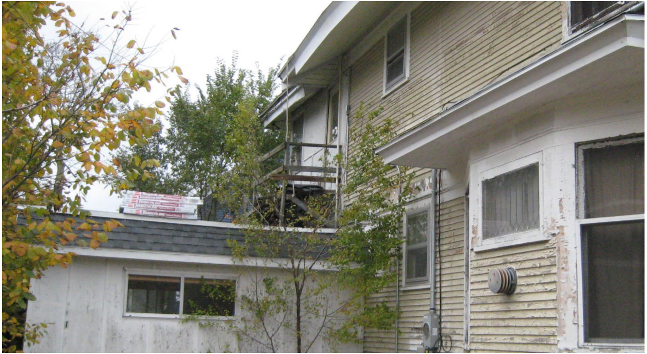
View of former second floor deck (photo from November 2019)
