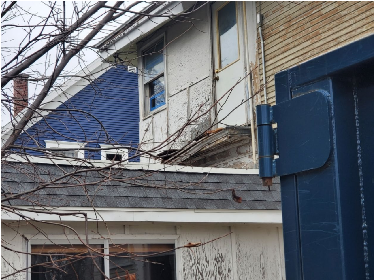
View of former location of second floor deck, and second floor exterior door to be removed
