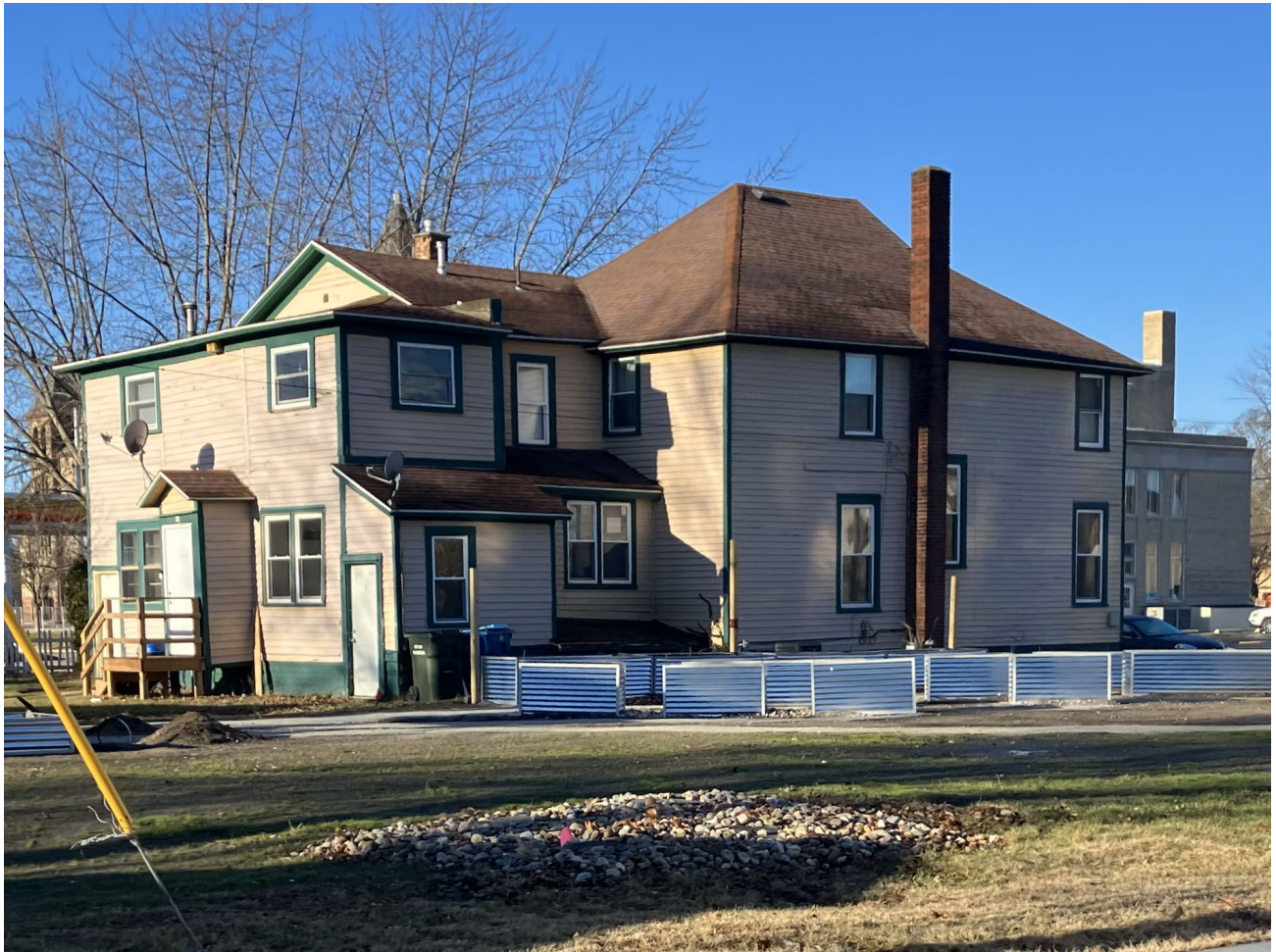
View of the south (rear) and east (side) elevations from rear alley, looking west.
