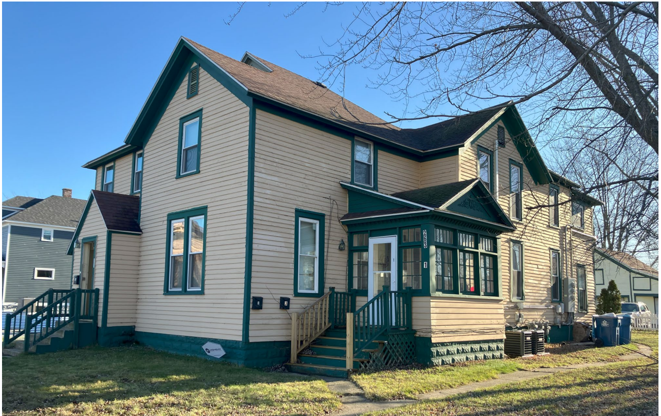
View of the north (front) and west (side) elevations from W. Muskegon Avenue, looking east.
