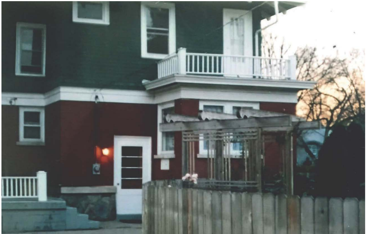
Photo showing old railing
