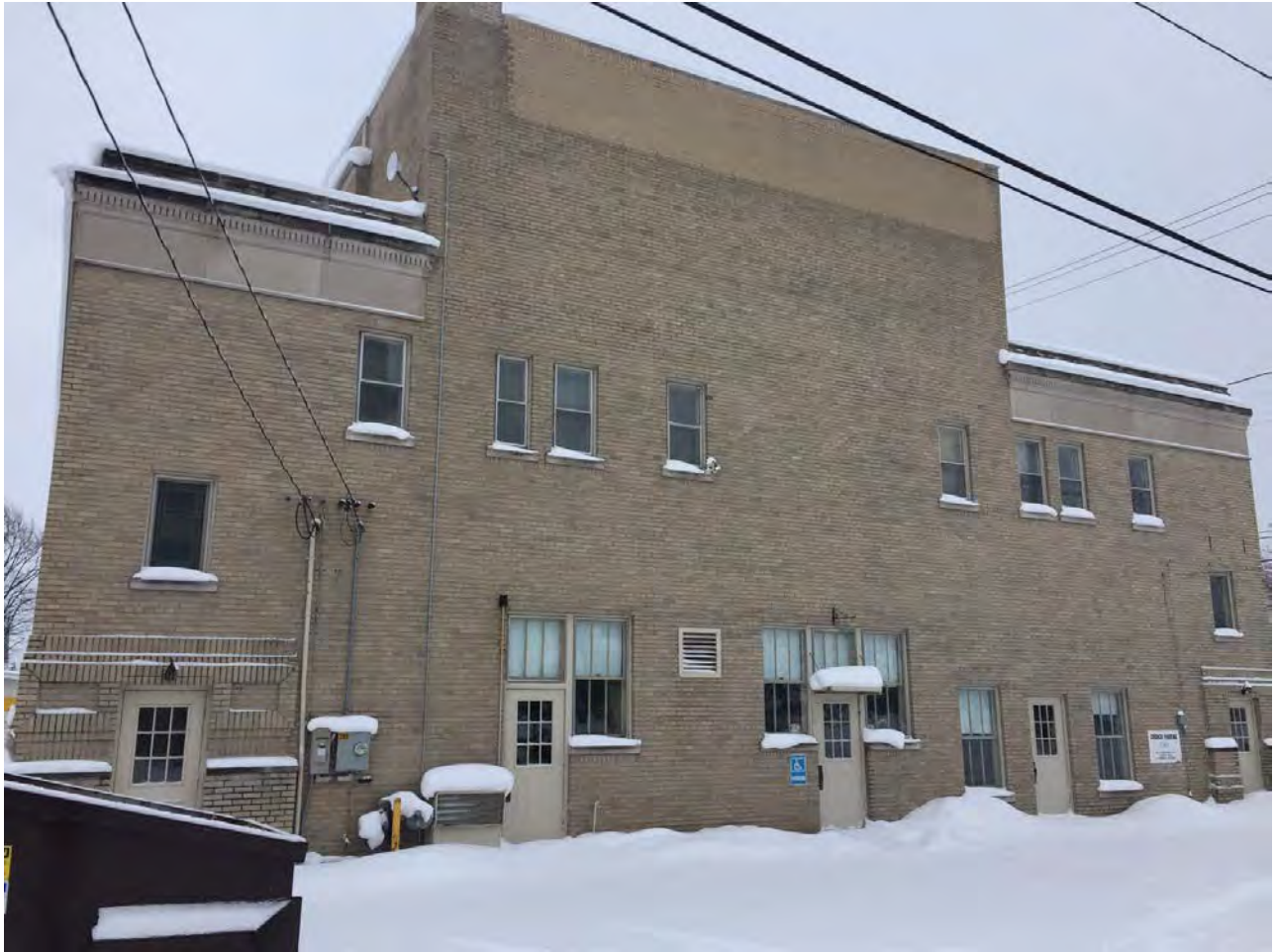
Rear of building (north), facing alley
