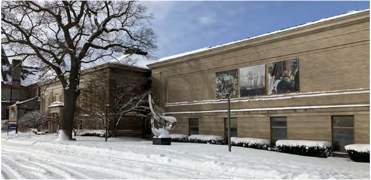
Current view of the original museum building (left) and its 1980s addition (right) from W. Webster Avenue, looking west.
