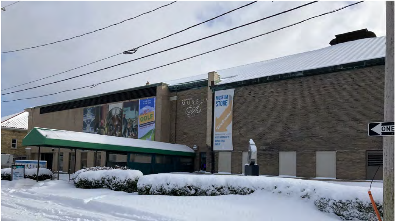
Current view of north entrance and alley, looking east.
