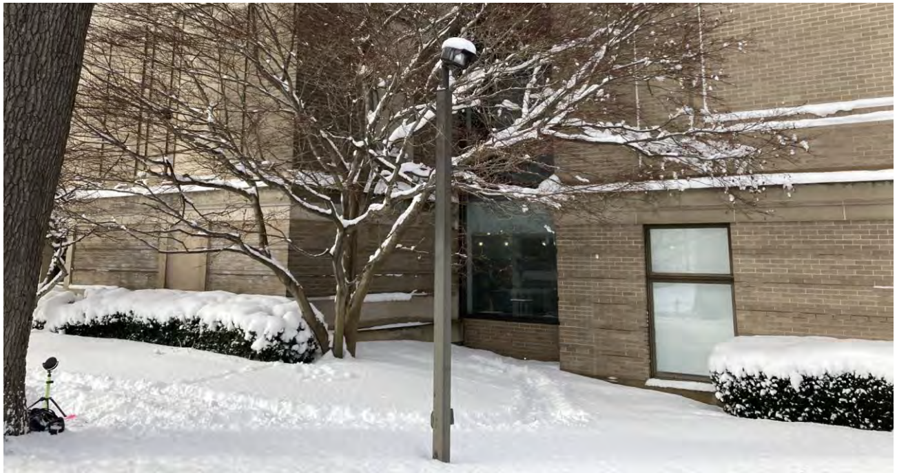
Current connection between original museum building and past building addition. Window on left is proposed to be replaced with a new entry door.
