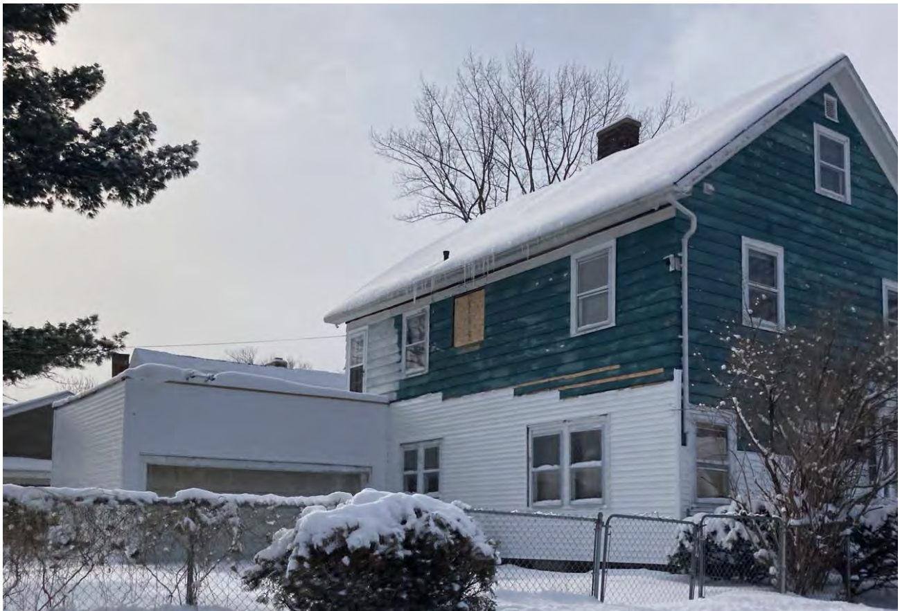
Current view of house from E. Grand, looking southwest. New vinyl siding being installed on the house and attached garage as well as a window that was removed from the second story are visible.
