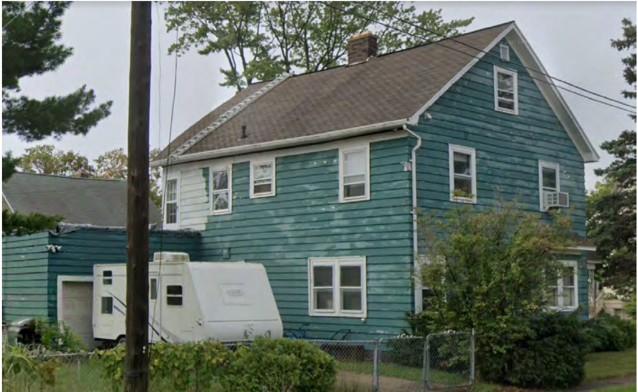
View of house from E. Grand Avenue, looking southwest (photo from October 2019)
