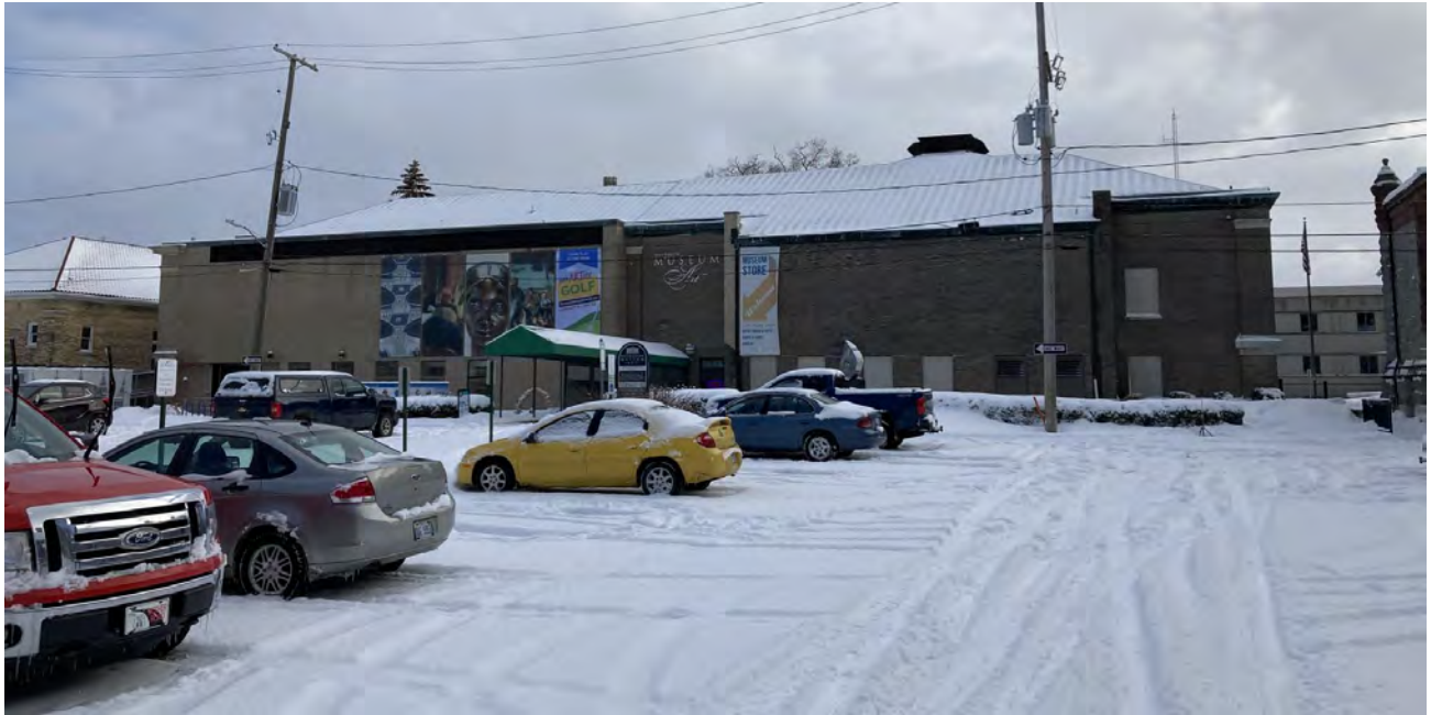
View of existing north elevation from W. Clay Avenue.
