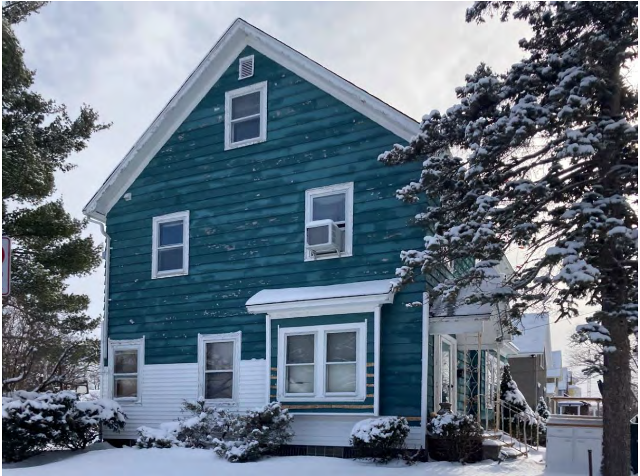
North elevation with vinyl siding being installed on the first floor.
