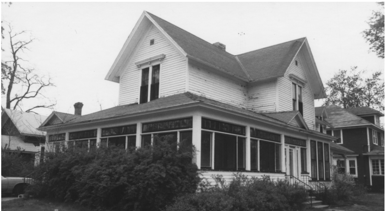
Historic photo of house showing original wood siding, entablature and brackets above second-story windows, and porch doors (photo from May 1984).
