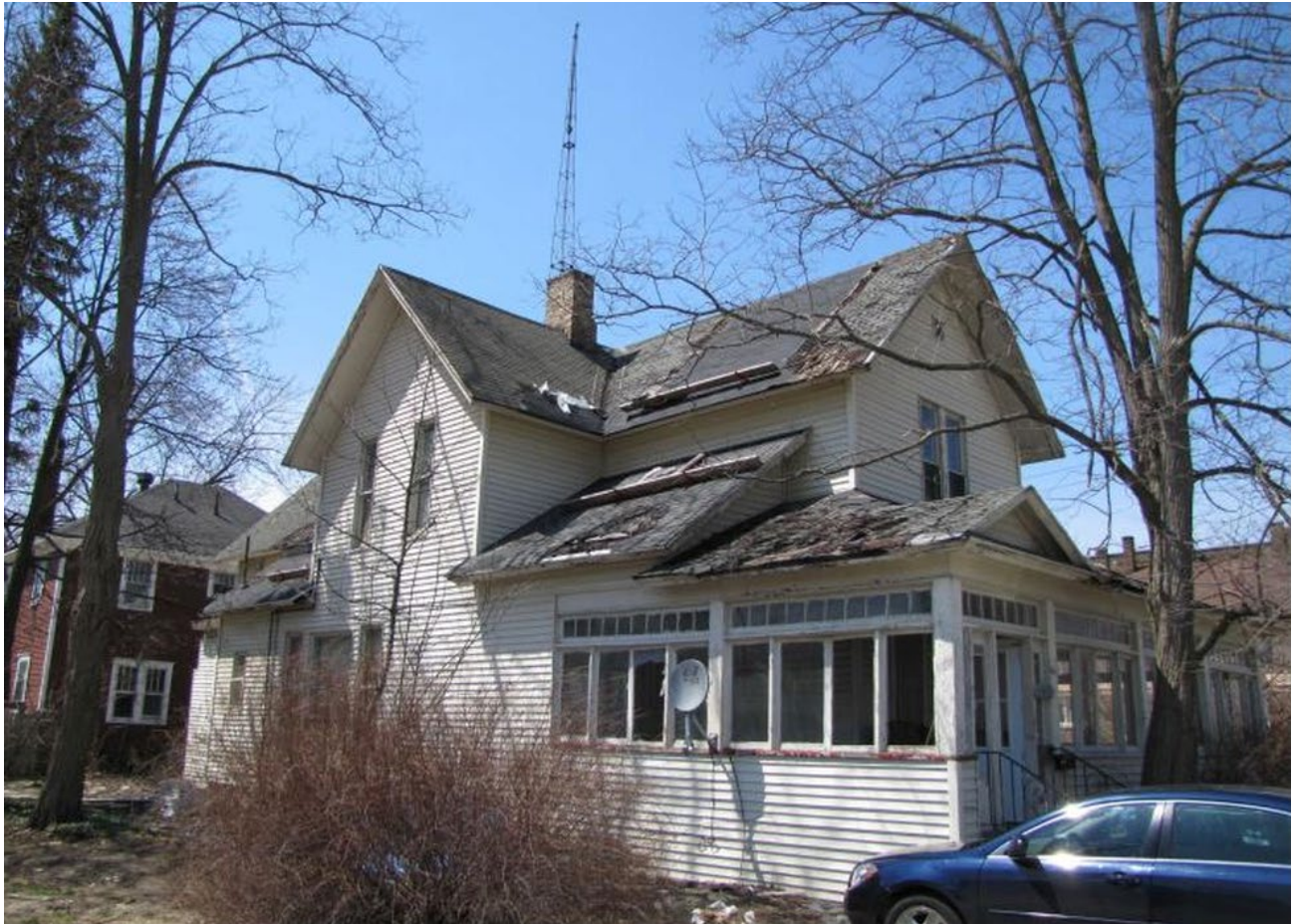
South elevation, looking west (photo from April 2013). Proposed attached garage would be at left.
