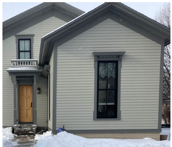
Photo of old siding (left) and new siding (right) on rear of house, facing alley
