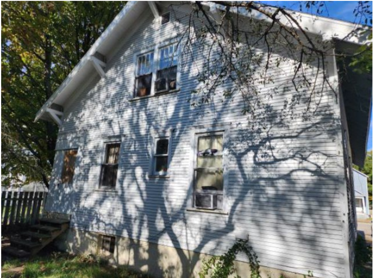
South (rear) elevation.
