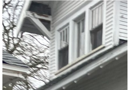
Fixed window on east elevation.
