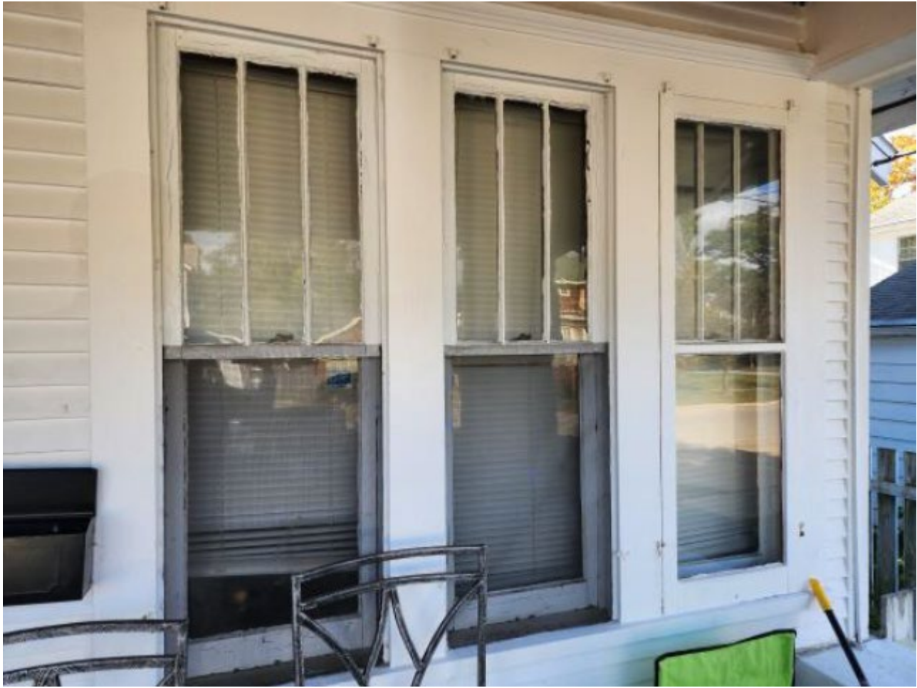
Detail of front porch windows.
