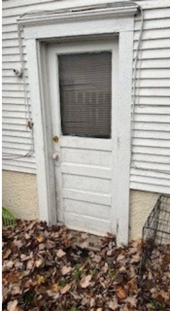
Door on west elevation.
