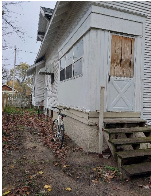
Enclosed rear porch and steps.
