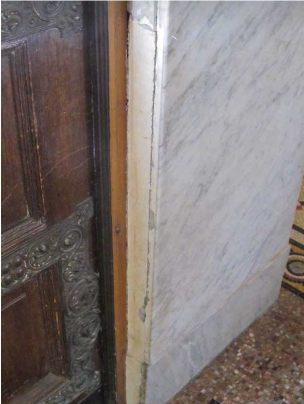
Front door, prior to refurbishing
