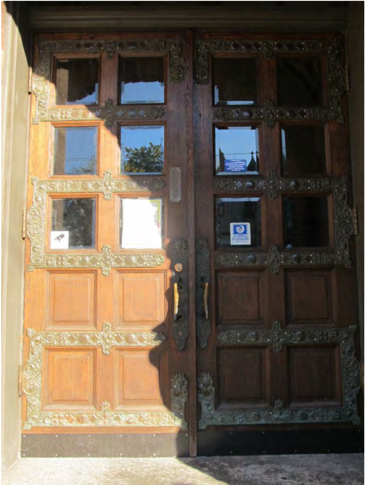
Front doors, prior to refurbishing.
