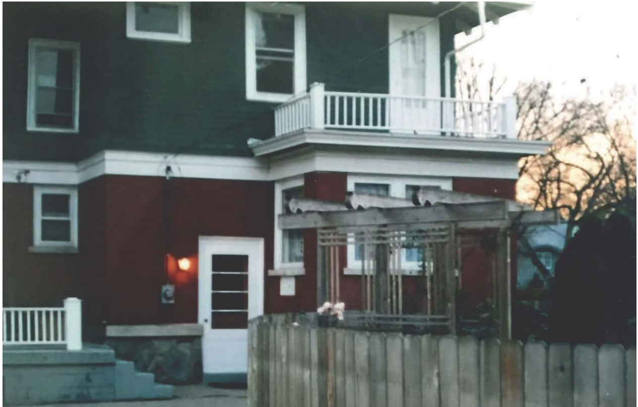
Photo showing old railing
