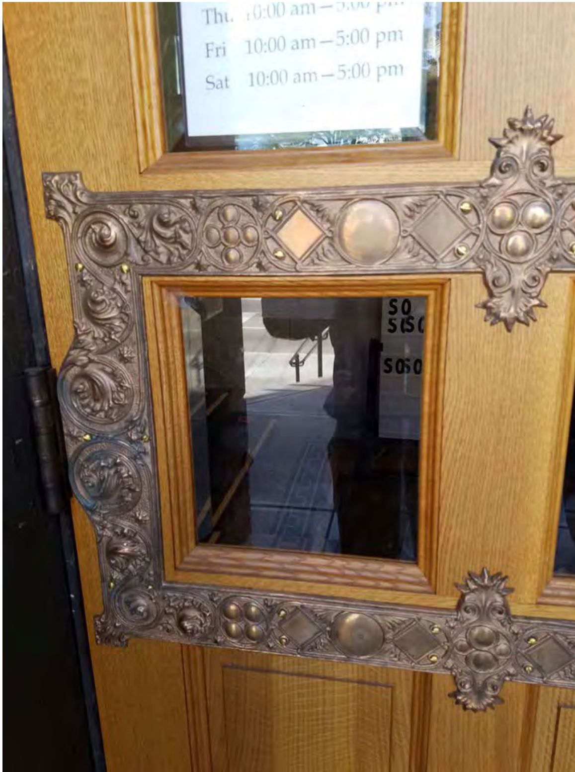
Front door, post refurbishing
