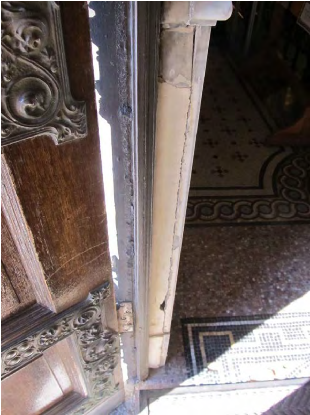
Front door, prior to refurbishing
