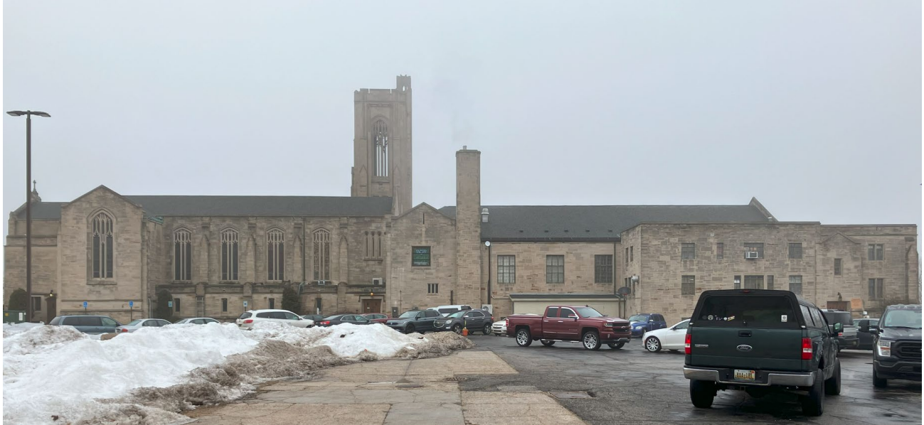
View of west (side) elevation from parking lot.
