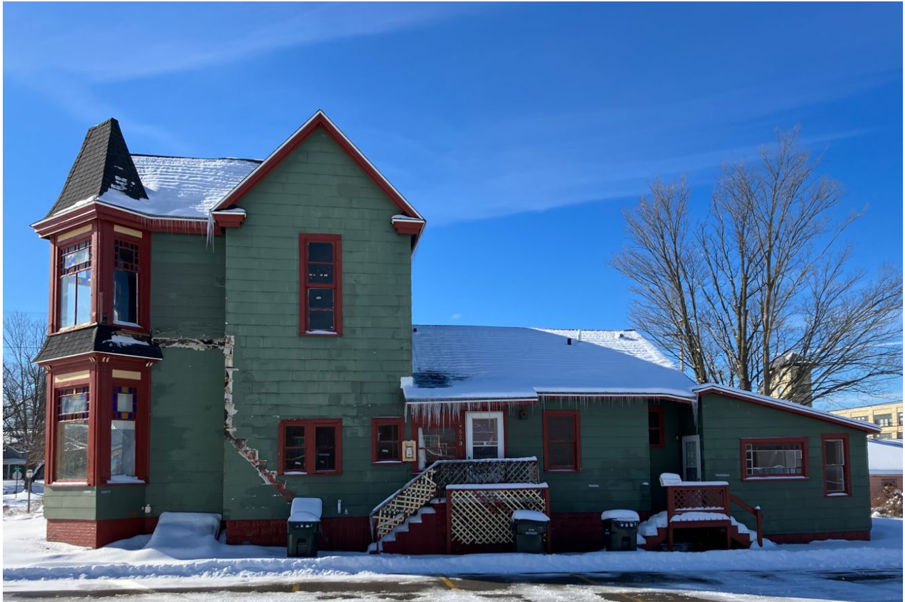
View of east elevation of house. Current cellar door visible in lower left (covered in snow).
