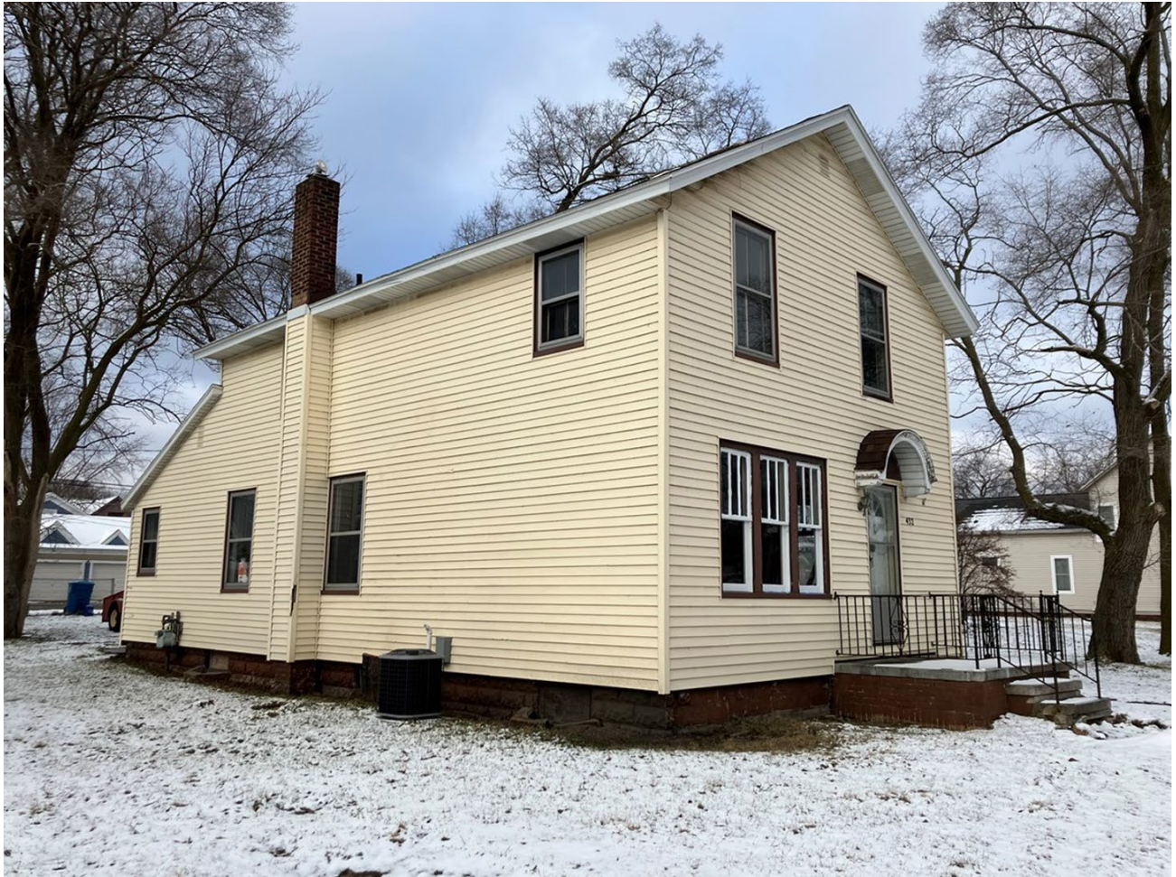
View from W. Muskegon Avenue, looking north. Visible are four windows on the west elevation to be replaced.
