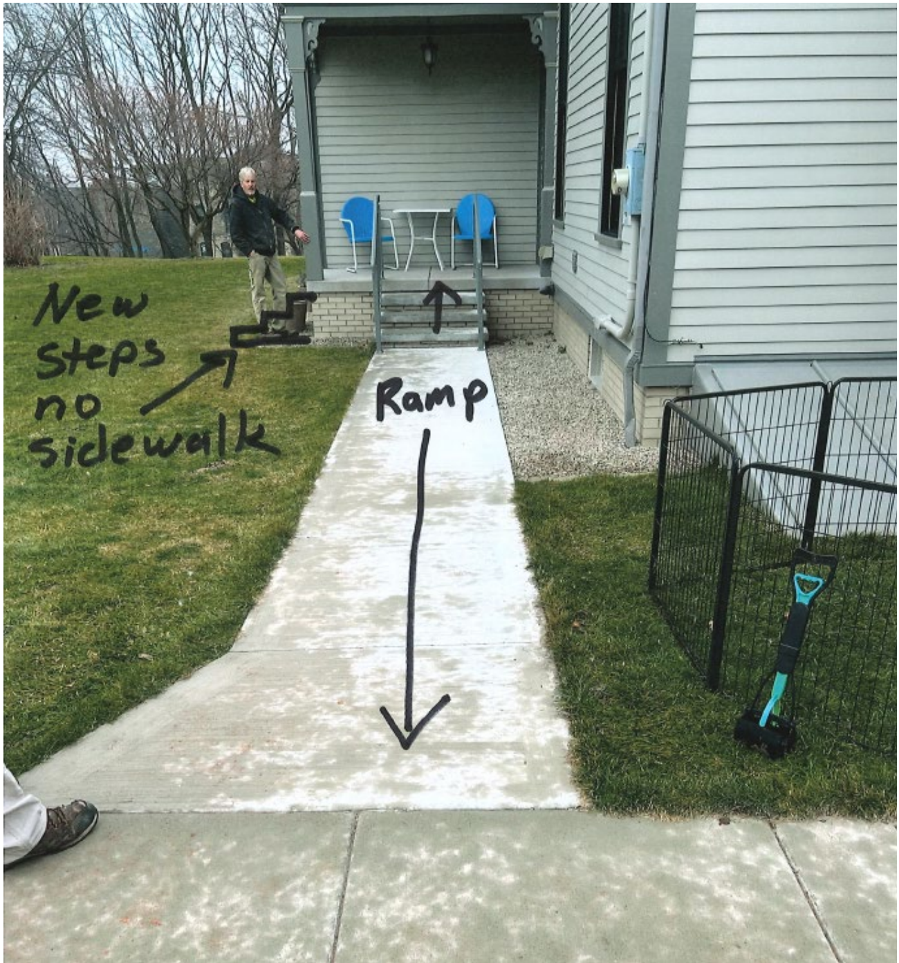
View of reach porch from the rear of the house noting the proposed ramp and stair location.
