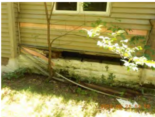
Foundation/siding deteriorating.
