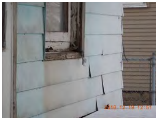
Siding coming up around the structure.
