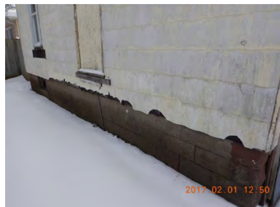
Foundation cracked/bowing.
