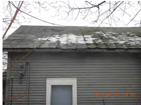
Deteriorated roofing.
