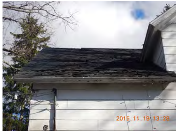
Deteriorated roof.
