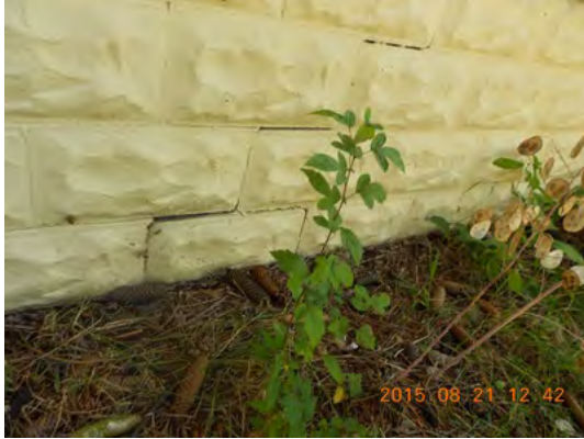
Cracked foundation.
