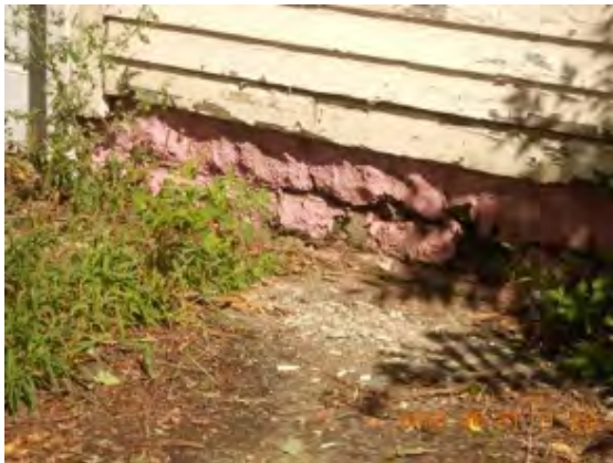
Foundation-holes/missing mortar/deteriorated.
