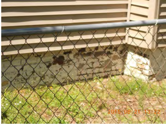
Foundation cracked/deteriorated.
