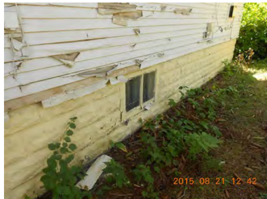
Foundation buckling/deteriorating.
