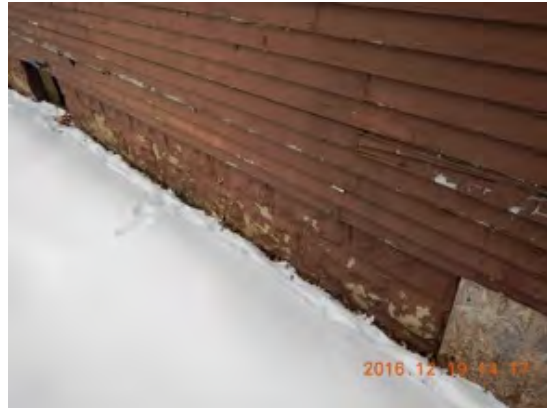
Foundation buckling.
