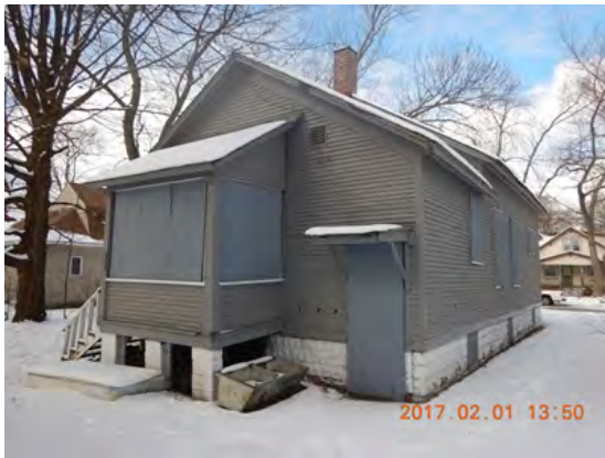
Rear of structure.
