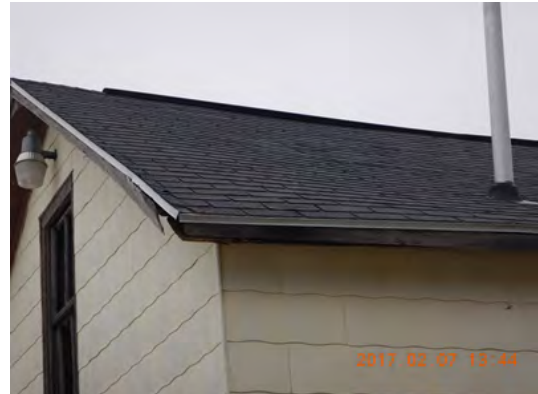
Warped roof.
