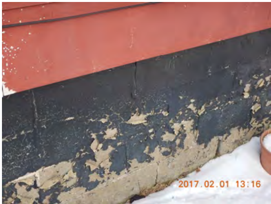
Foundation-cracked/deteriorated/buckling.
