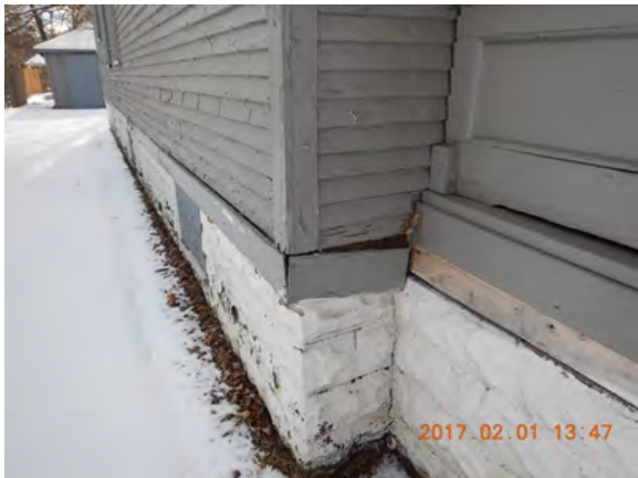
Foundation deteriorated-wood siding falling.
