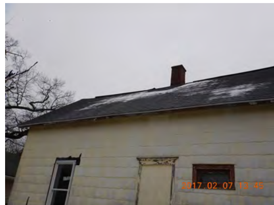
Warped roof.
