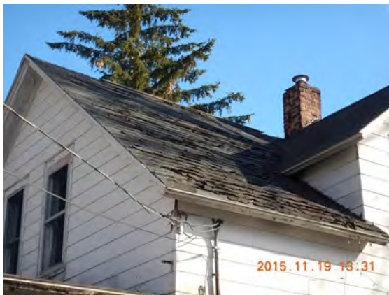
Deteriorated roof.
