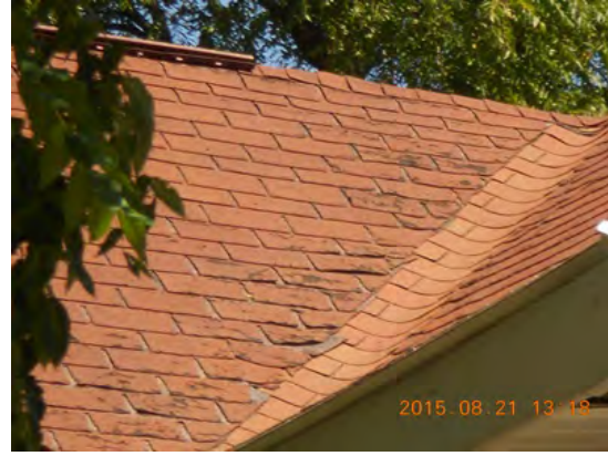
Deteriorated roofing.
