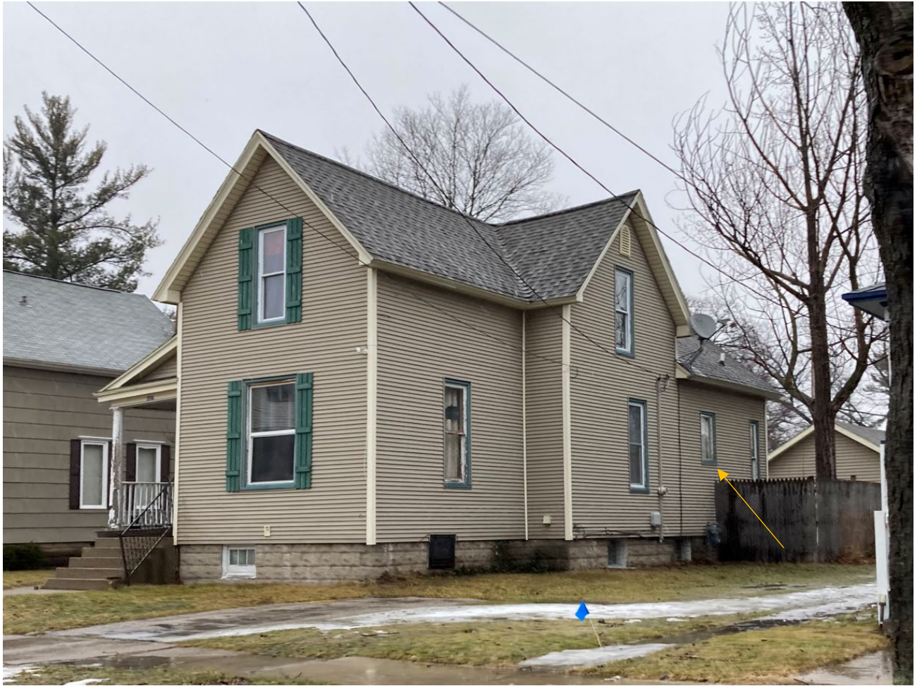
View of house from Clinton Street showing the single window on the south elevation to be replaced.
