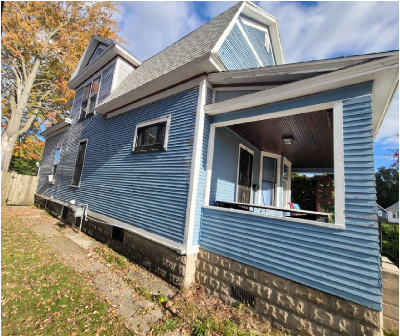
View of west elevation.
