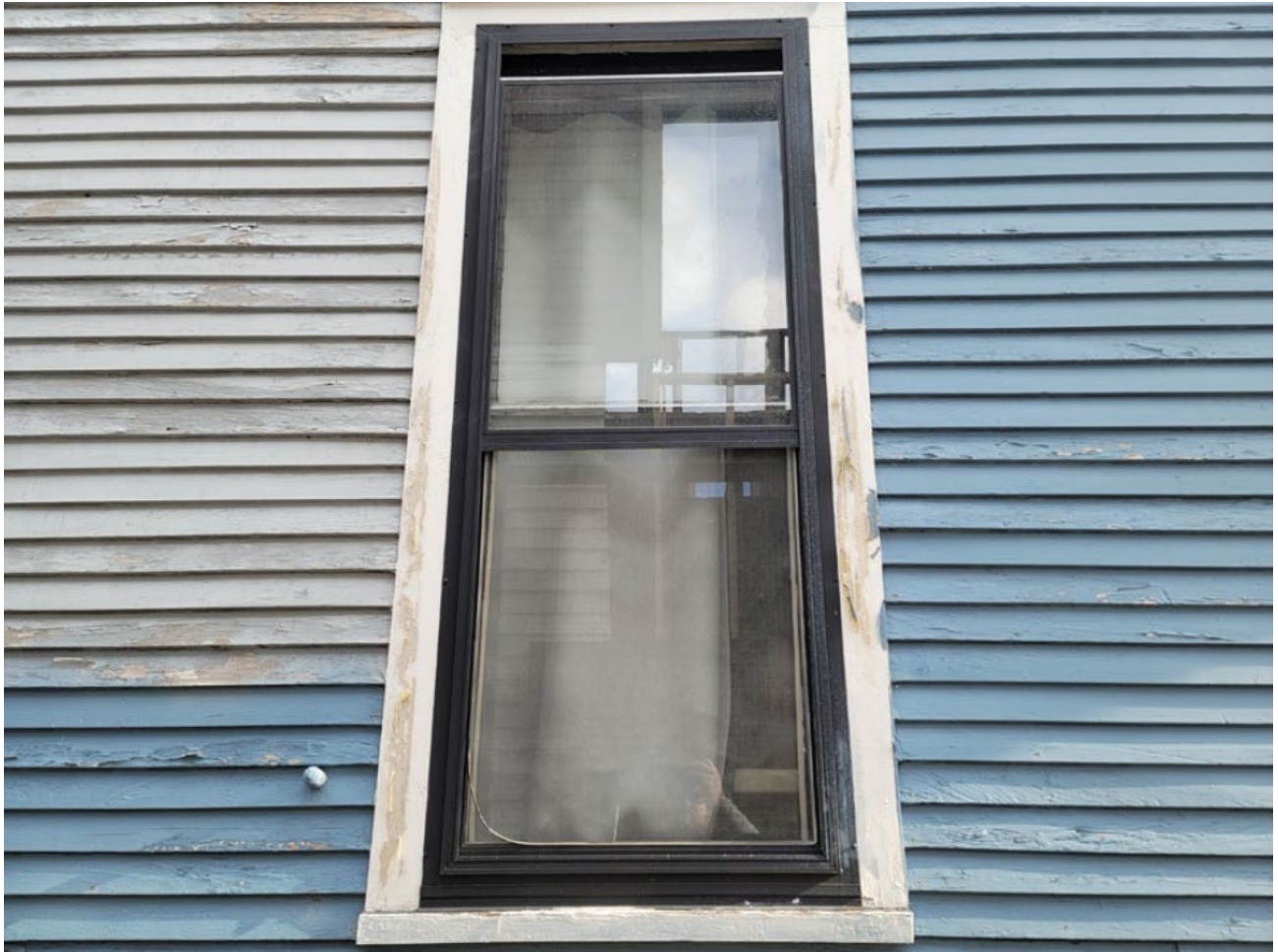
Detail of window on west elevation.
