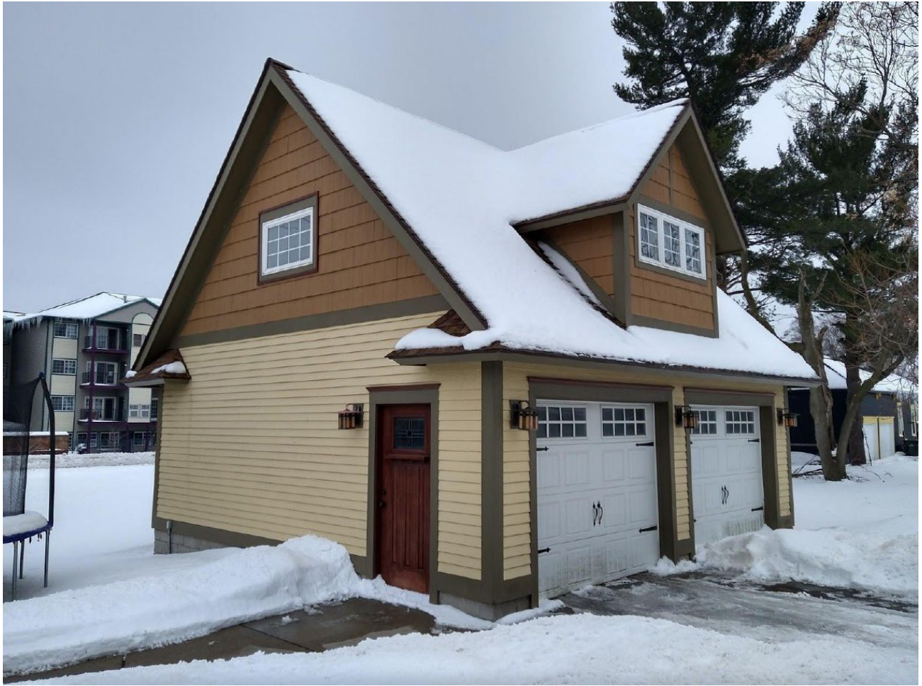
Garage viewed from rear alley, looking south. Proposed new entry door will replicate existing door
