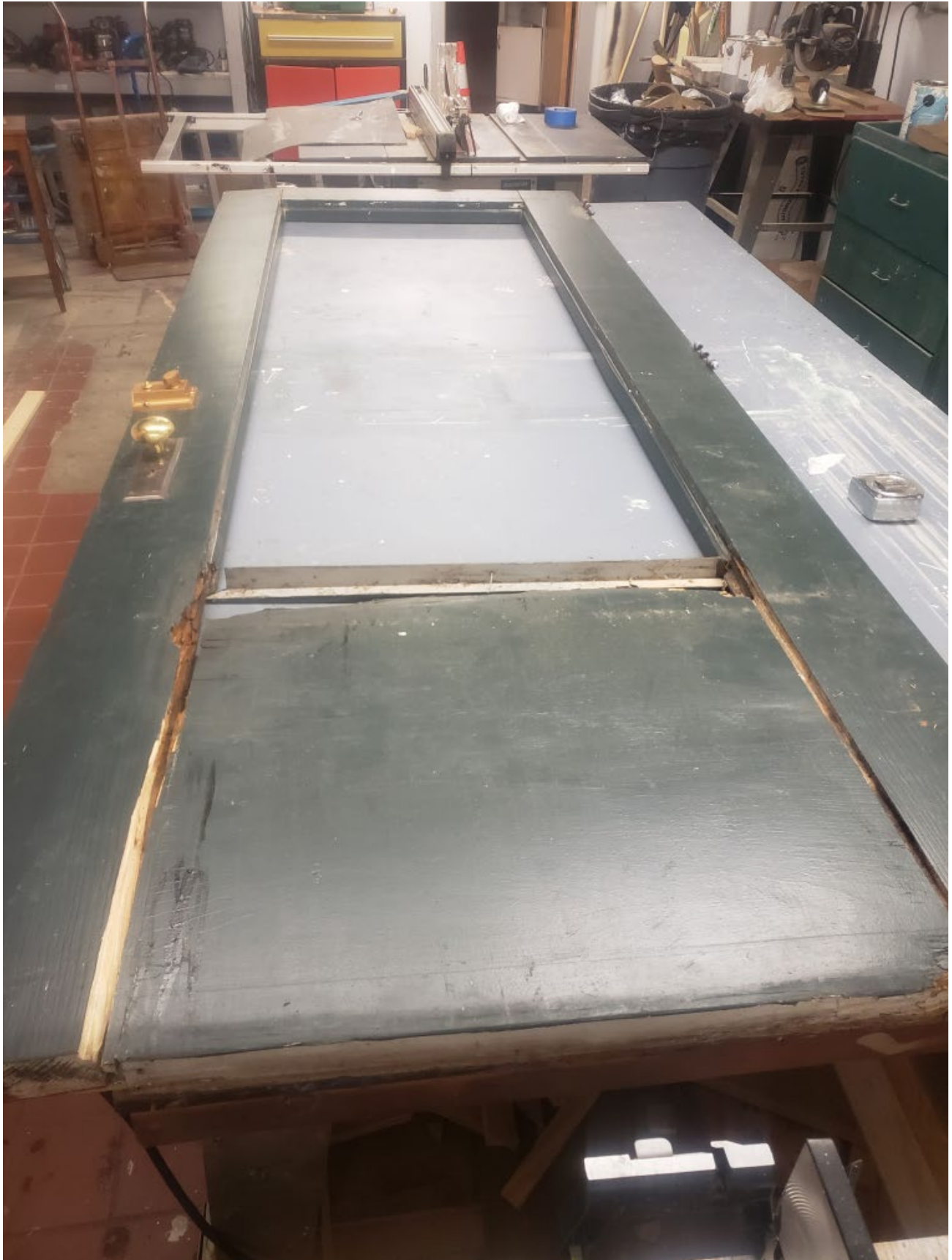
Existing wood door (presently removed from building)
