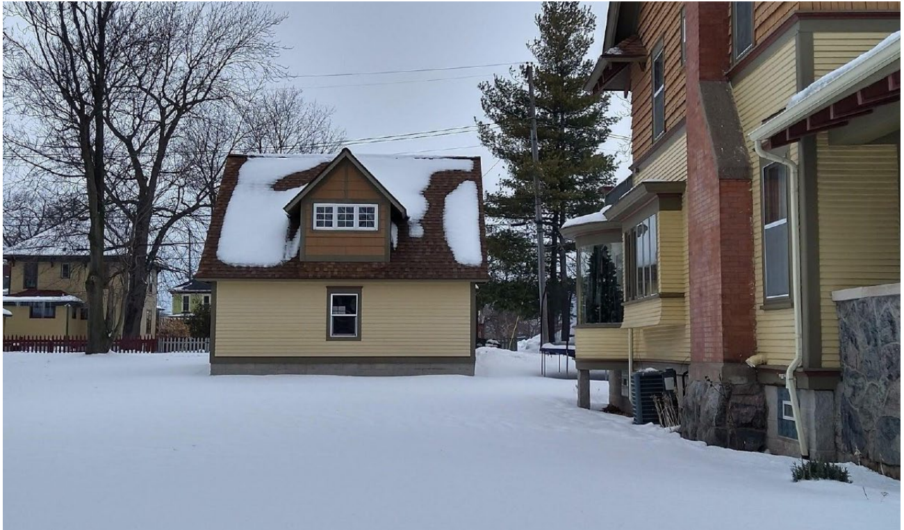
Detached garage viewed from W. Muskegon Avenue, looking northwest. Main house visible at right
