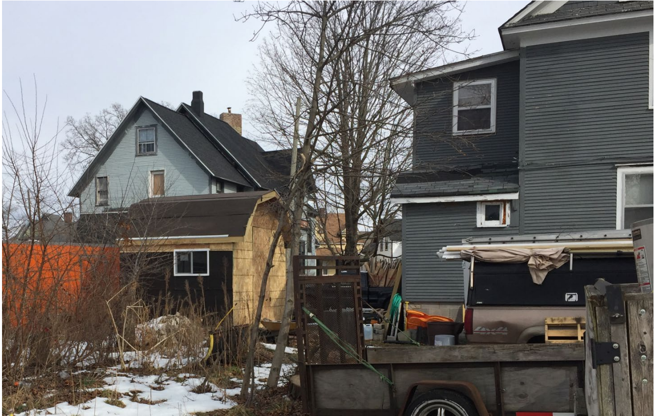
Shed in rear yard of 24 Morrall Avenue (view from street was obstructed by parked trailer)
