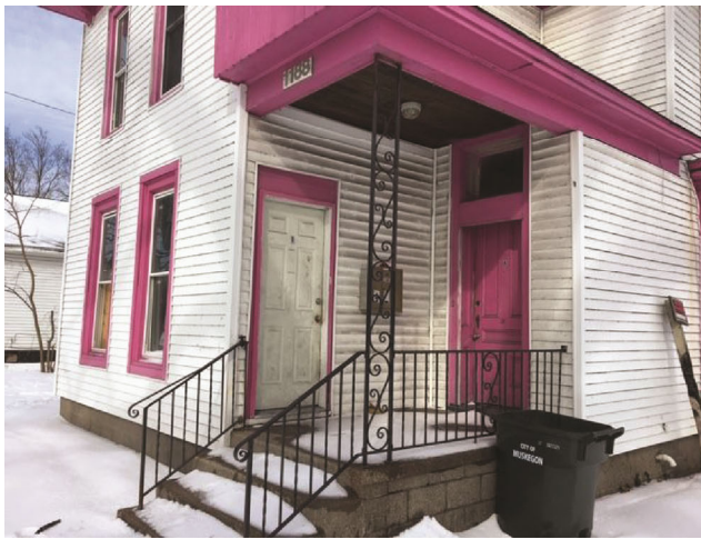
Left-hand door on porch to be removed, all concrete porches to be covered with wood. Iron railings to be replaced with wood railings
