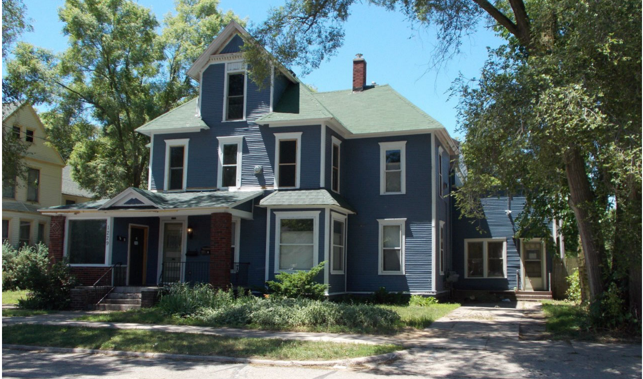
June 2016 photo (prior to window replacement work)
