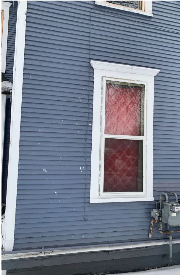
Window on north façade to be replaced
