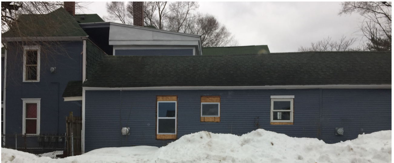
North façade window replacement, far left, first floor window proposed to be replaced
