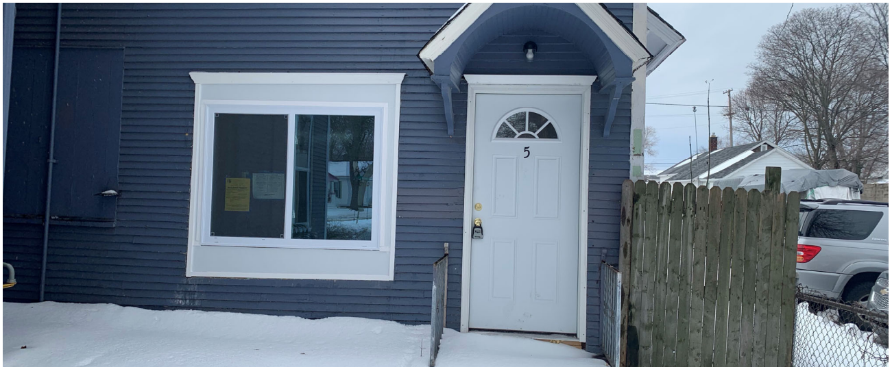
New window installed on east façade
