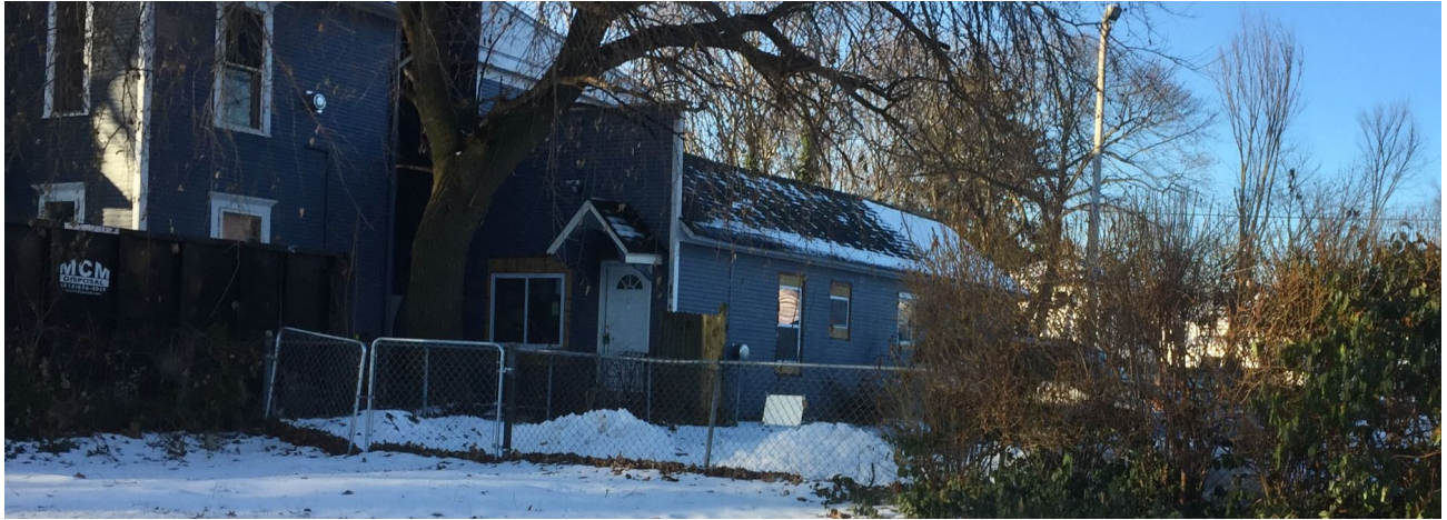
Photo showing north and east façade window replacement work in process
