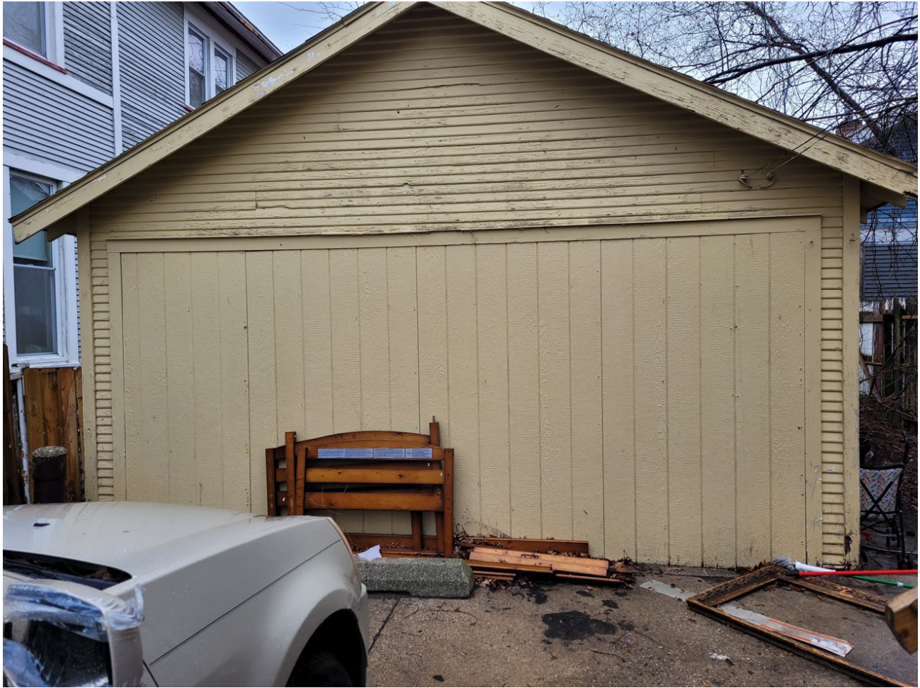
View of detached garage proposed to be demolished.
