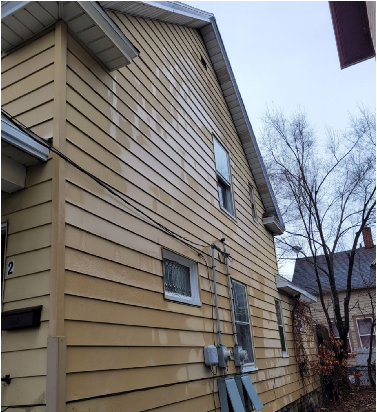
View of south elevation. All windows visible except the fixed, decorative window are to be replaced.
