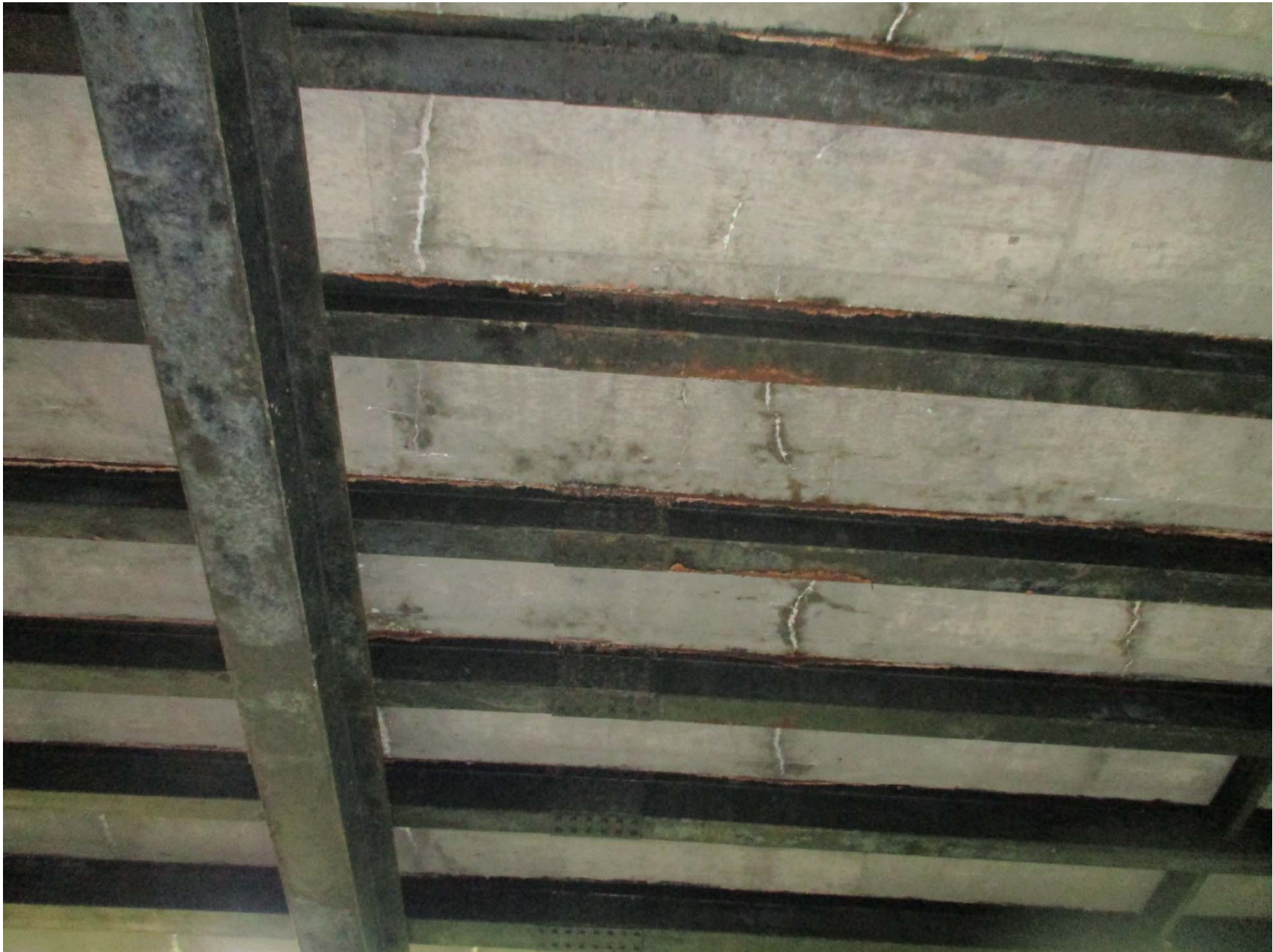
Light rust along beam flanges, splices remain good
