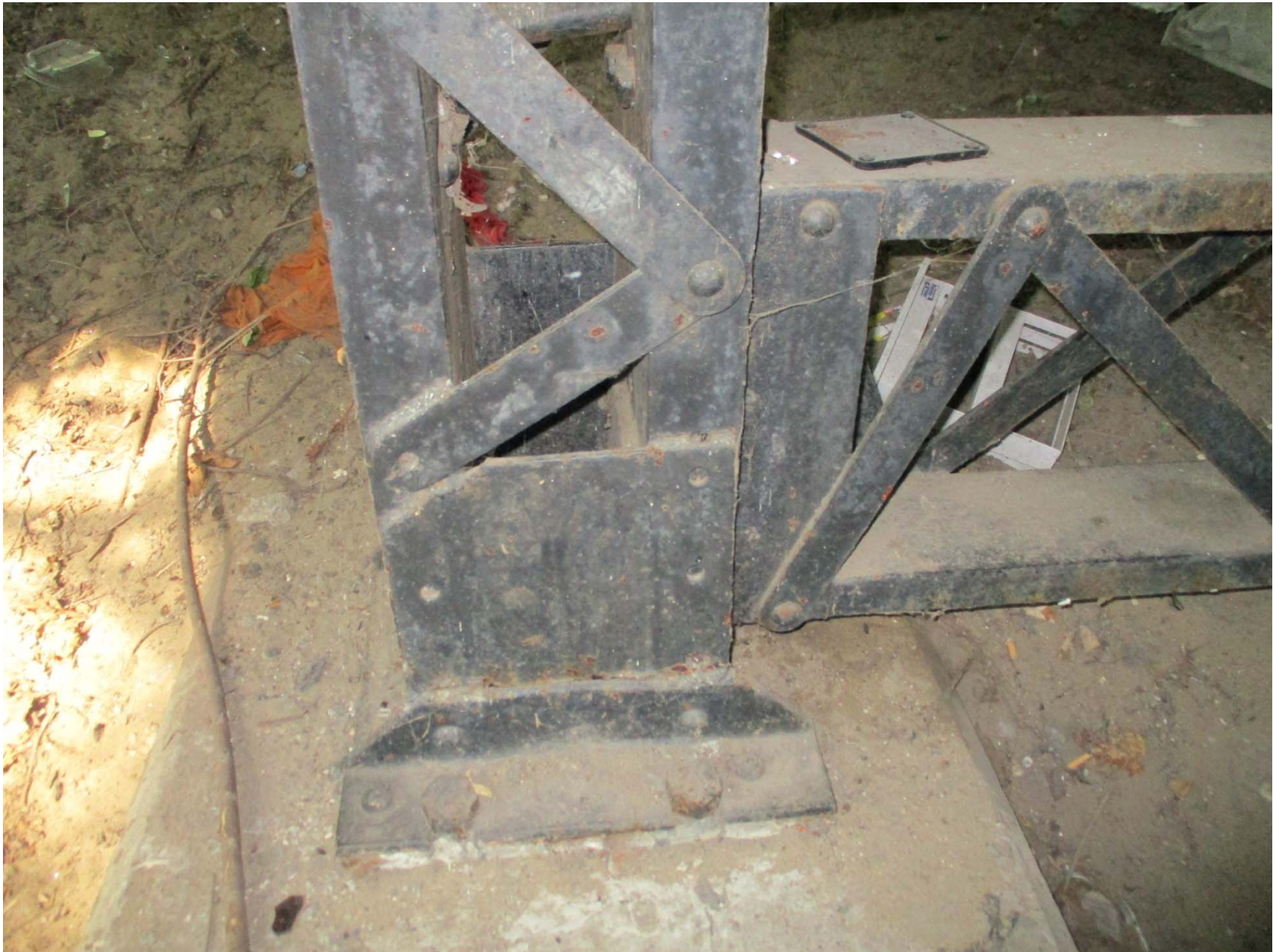
Lower plate are welded at each pier column
