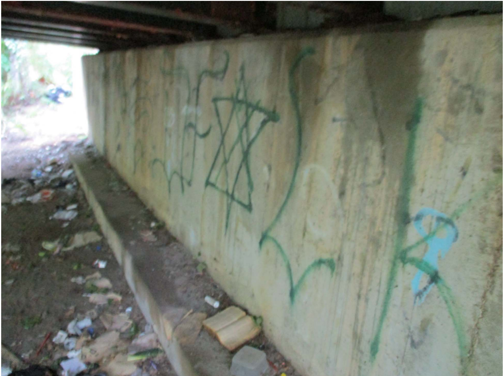
West abutment elevation, exposed footing, no undermining
