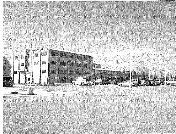
1050 W. Western Ave. – Rear view
