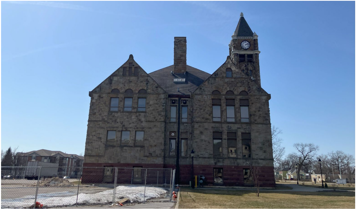
View from 3 rd Street, looking southwest.
