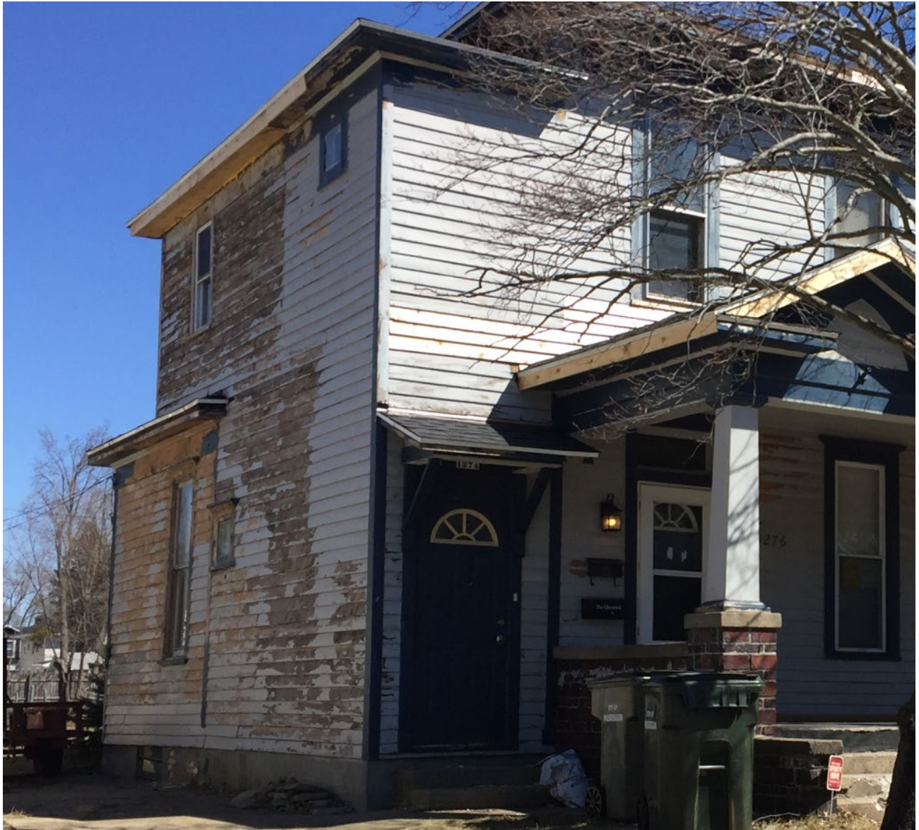
View of northwest façade showing repairs made to cornice and eaves
