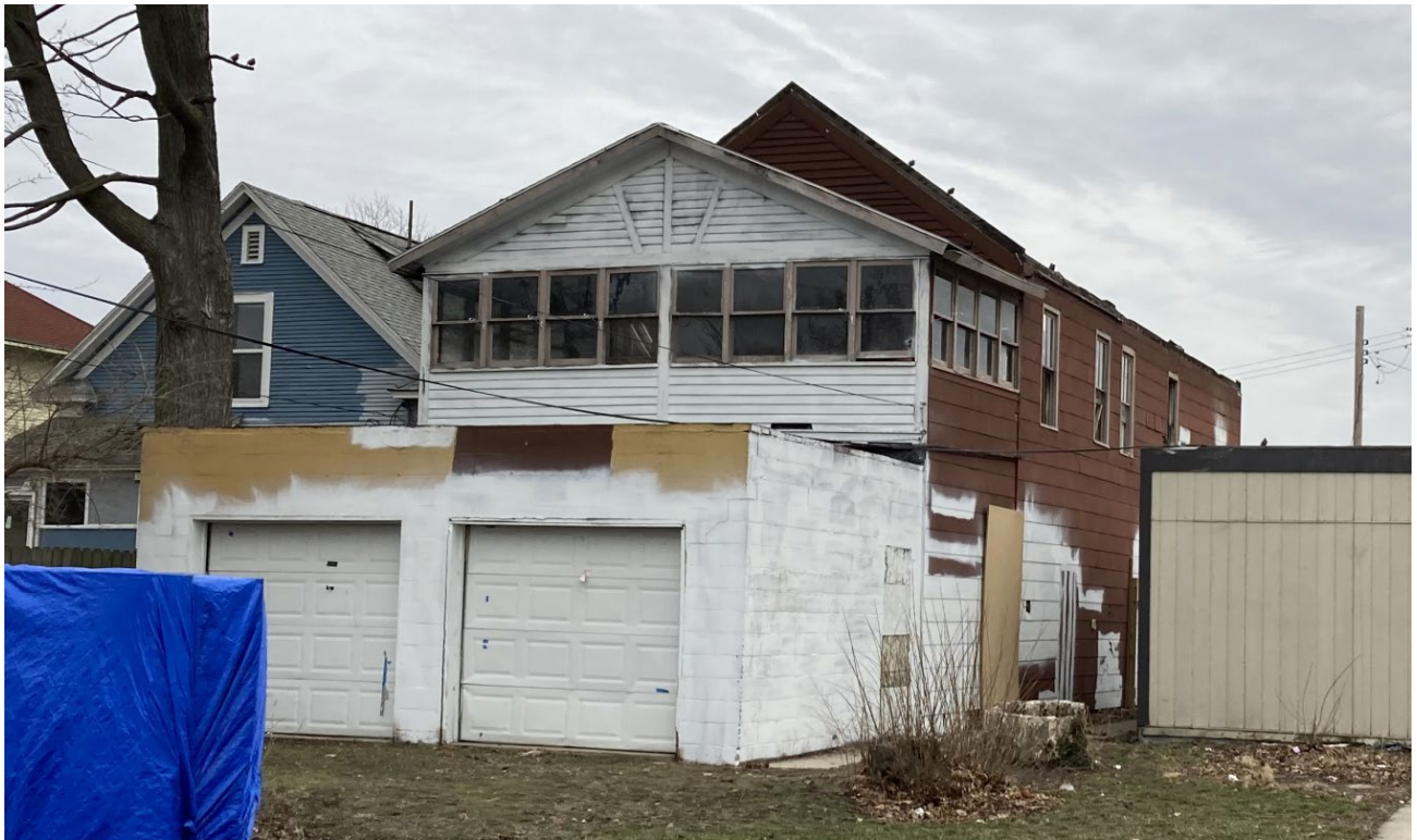
View of building from rear alley, looking east.
