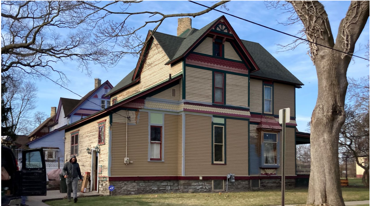
View of house from W. Larch Avenue looking south. Windows from (1) and (2) visible on rear of house. (3) and (4) are around the back corner of the house near where the white fence is visible
