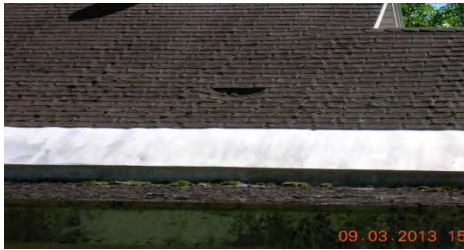
Roof-North side of home.
