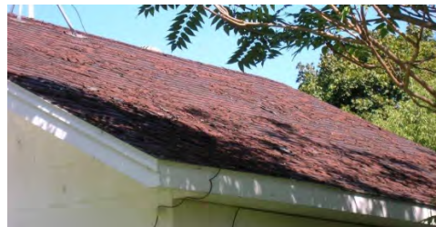
Roof-South side of home.
