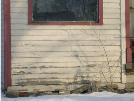
Foundation and exposed wood.
