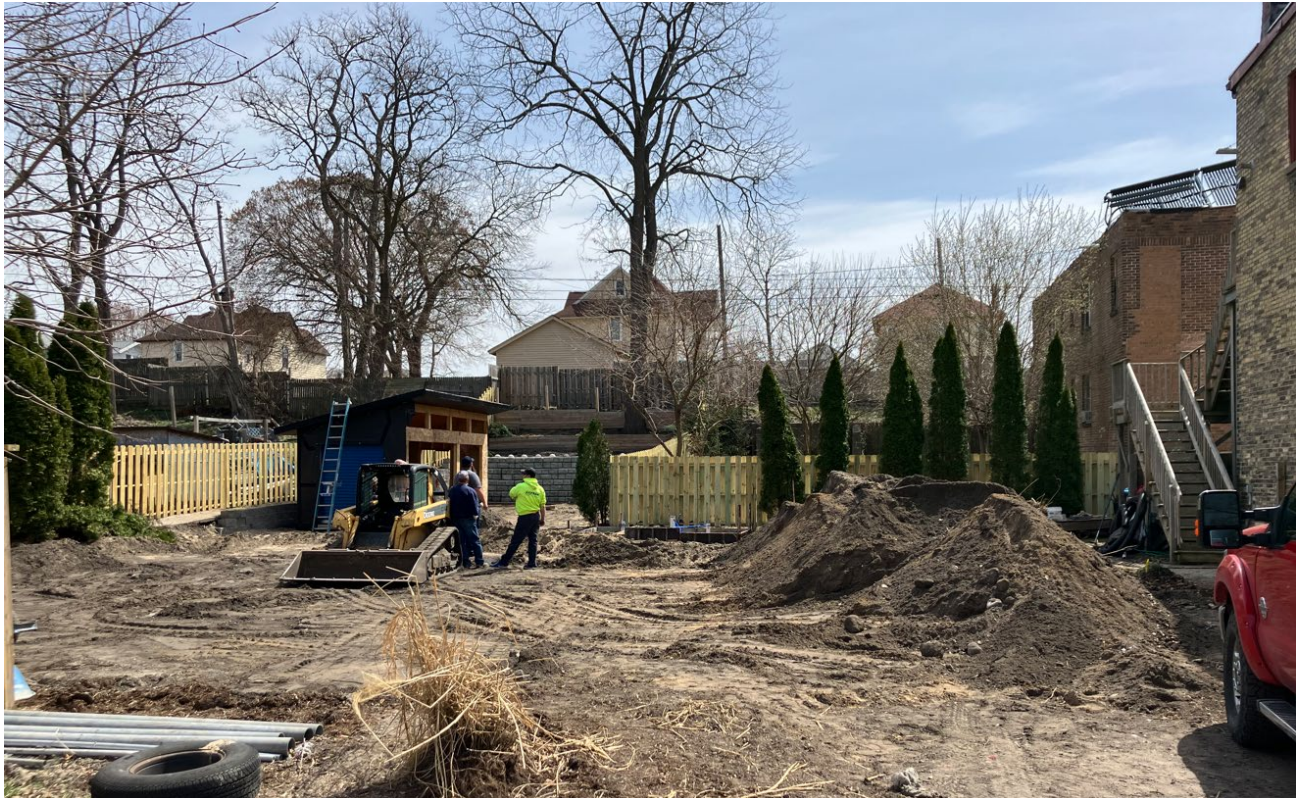
View of open space from W. Clay Avenue, looking east. Existing building visible at far right.
