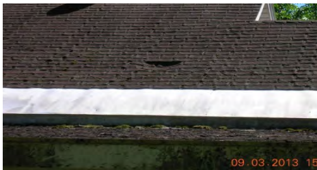
Roof-North side of home.
