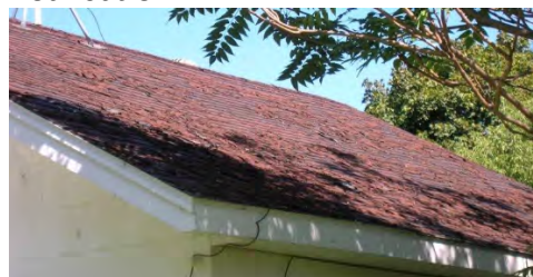
Roof-South side of home.
