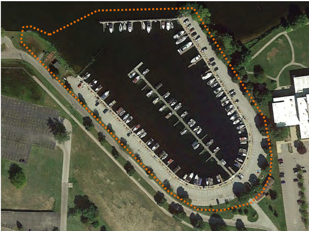
Figure 1: 2018 Google aerial image; Main basin survey limits shown in orange (approx. 3 AC)
