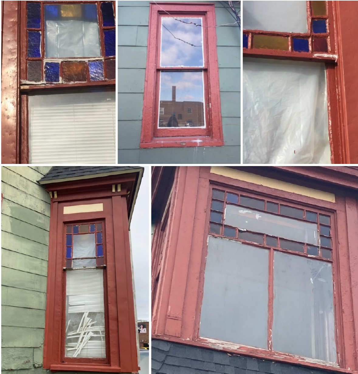
Detail of existing window conditions (photos from June 2022).
