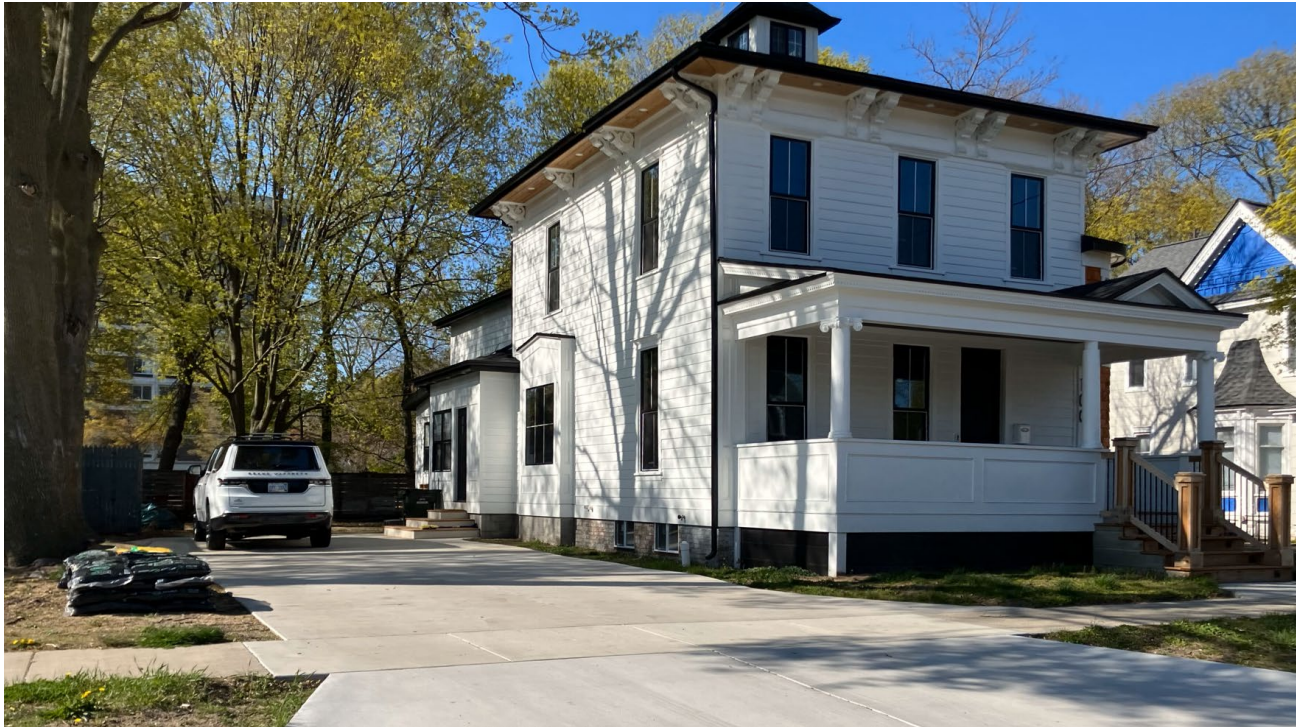
View of house from Diana Avenue, looking north. Proposed location of new two stall garage visible at left.
