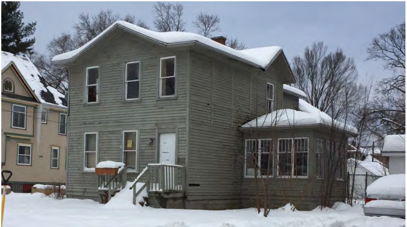
Same view as above, but from March 2018 showing former windows on enclosed porch on the northwest side of the house.
