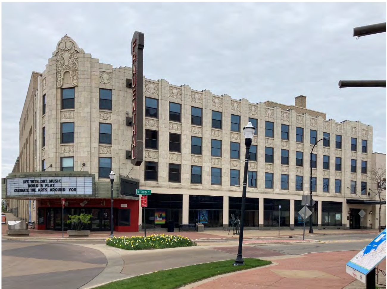
View of building from W. Western Avenue.
