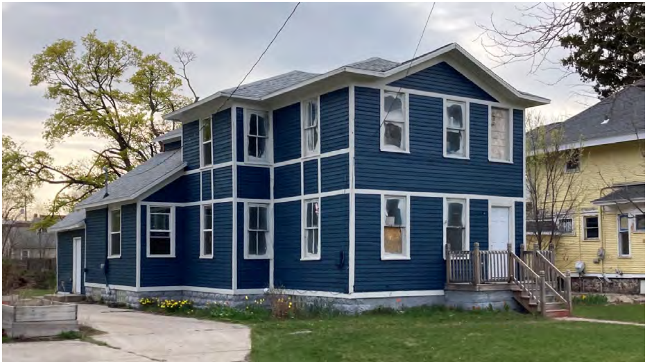
View from Ransom Street, looking west.
