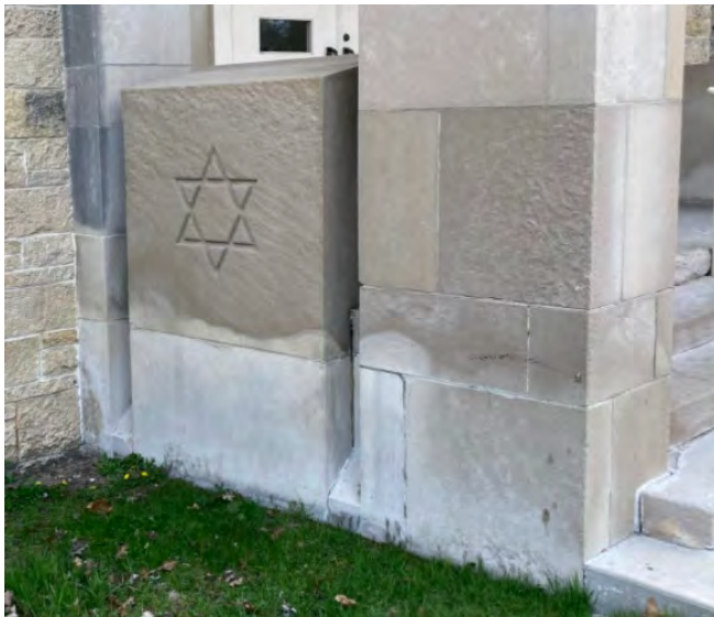
Stone proposed to be removed and reset, view from both sides.
