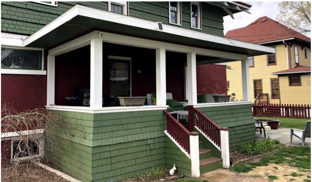
View of rear porch from backyard.
