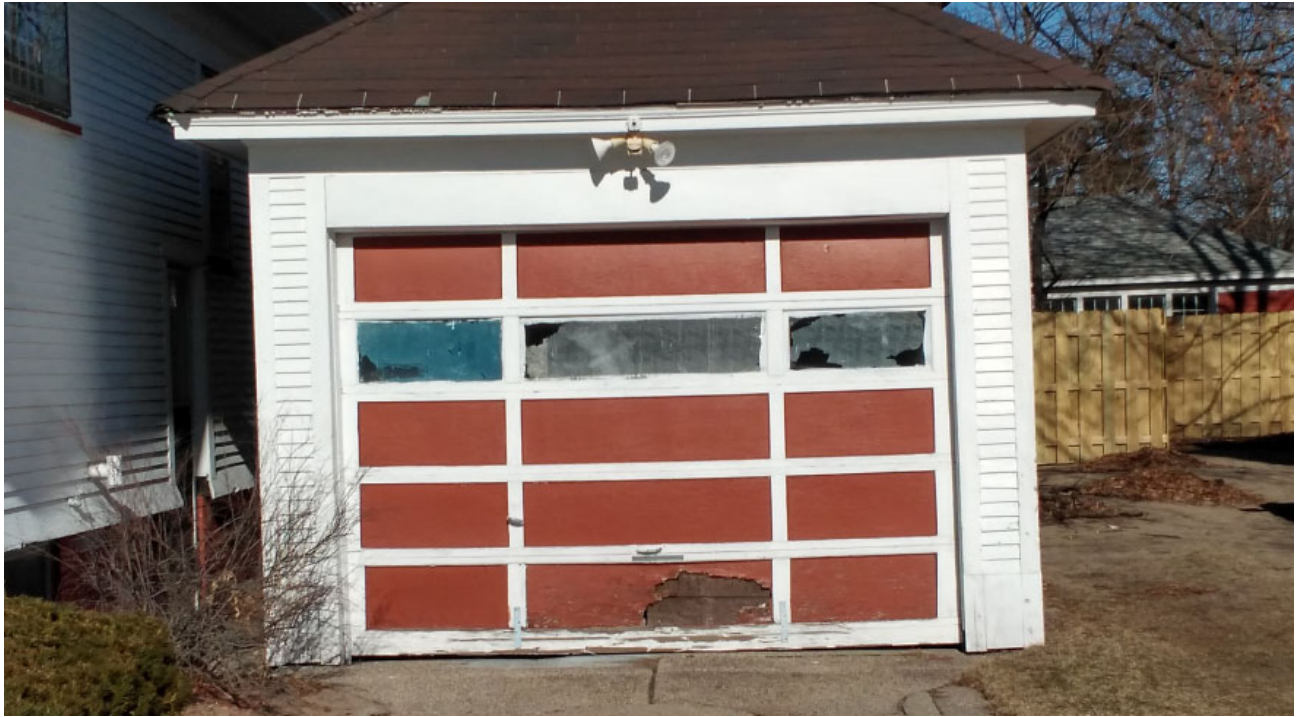
Existing garage door at 1140 Terrace
