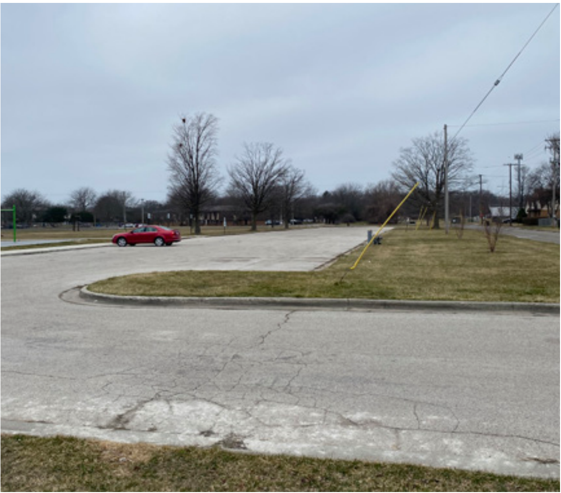
EXISTING PARKING LOT -Paving is in poor condition.
