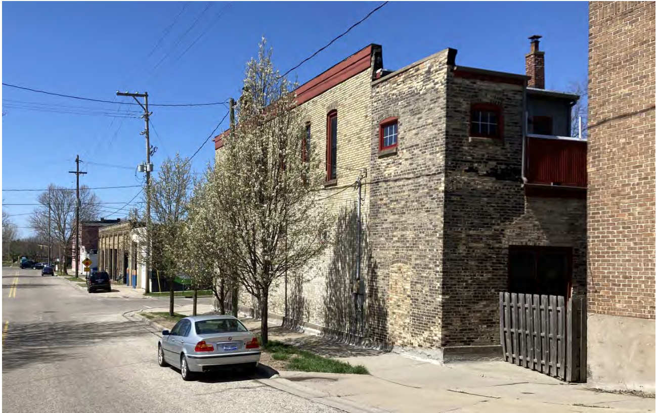
View of building from 7 th Street, looking north.
