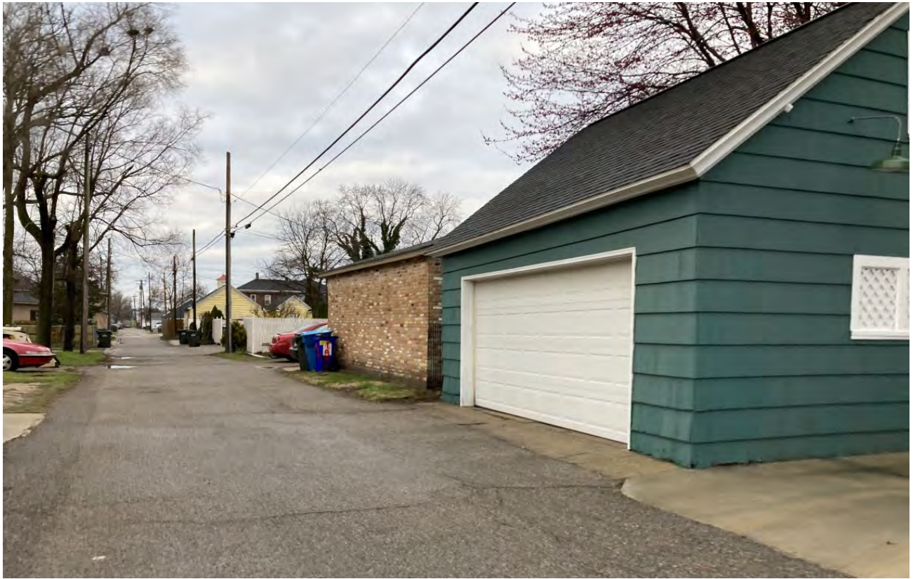
View of detached garage (brick) from rear alley, looking west.
