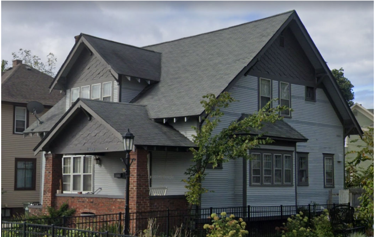
View of north and east elevation from Jefferson Street (photo taken October 2019).
