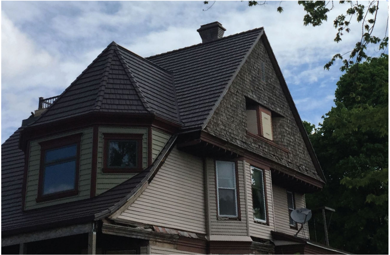
View of south façade from Terrace Street showing existing shingles and three of the six total windows (covered by tan panels in this photo) to be replaced on the third floor.
