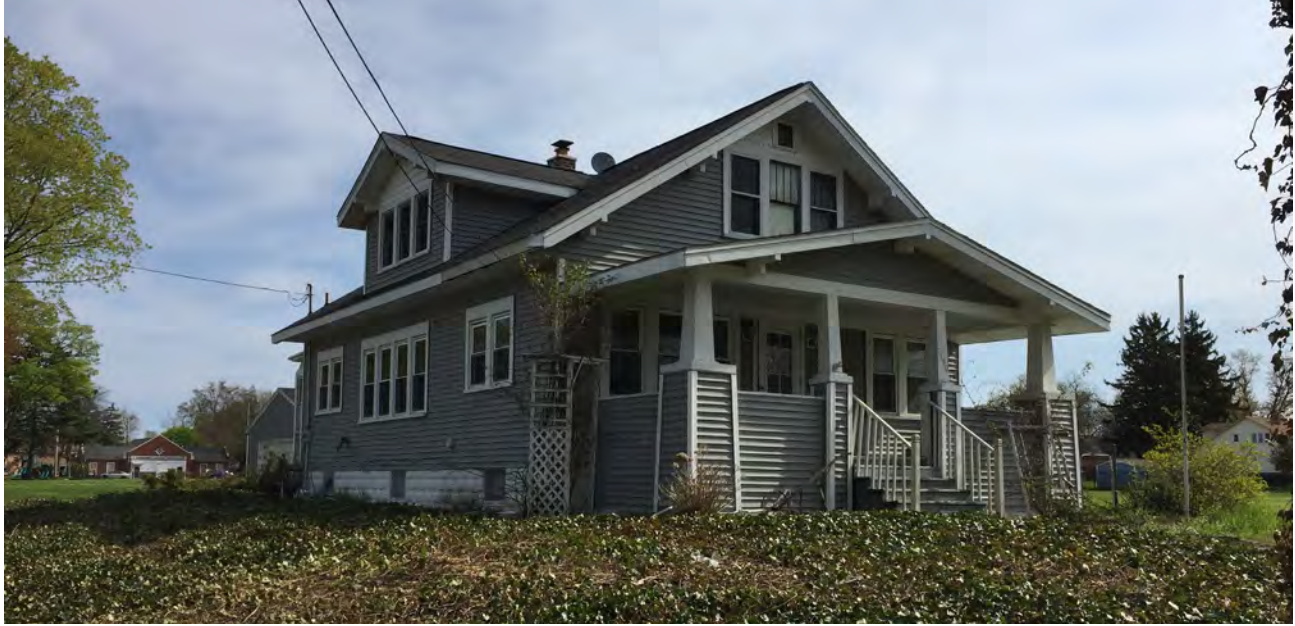
House at 1190 Ireland
