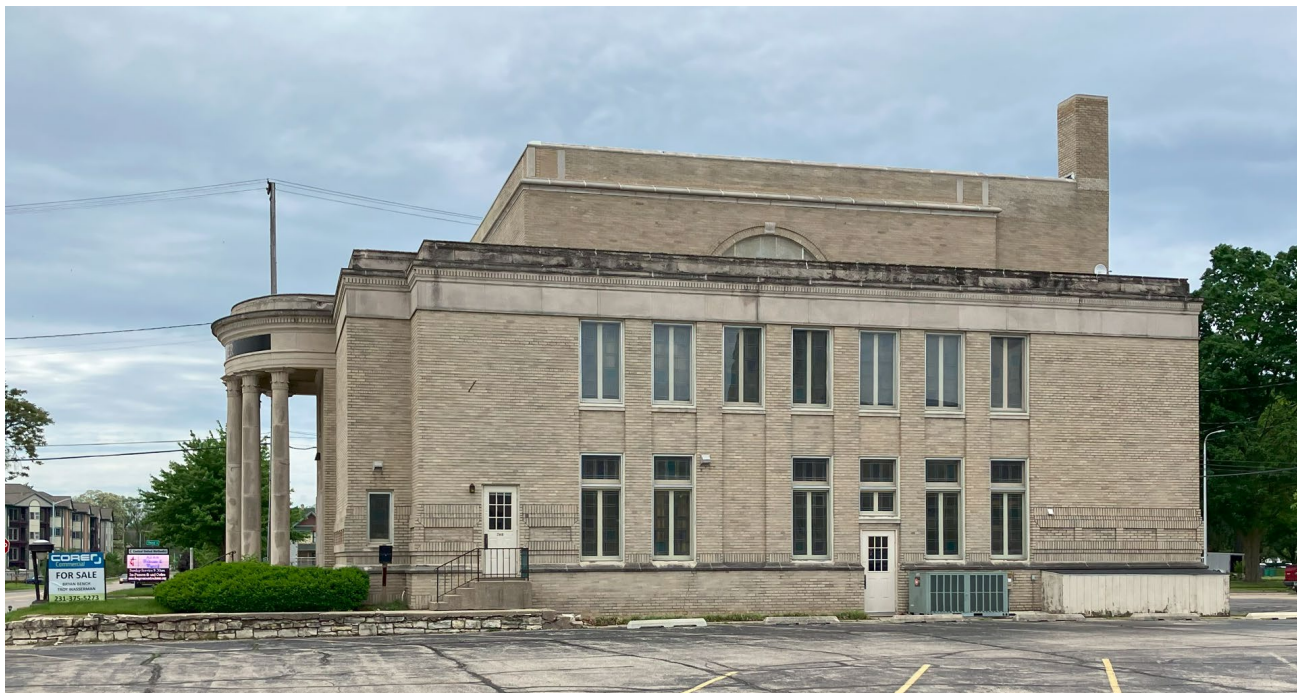
View of the east (side) elevation from W. Muskegon Avenue.
