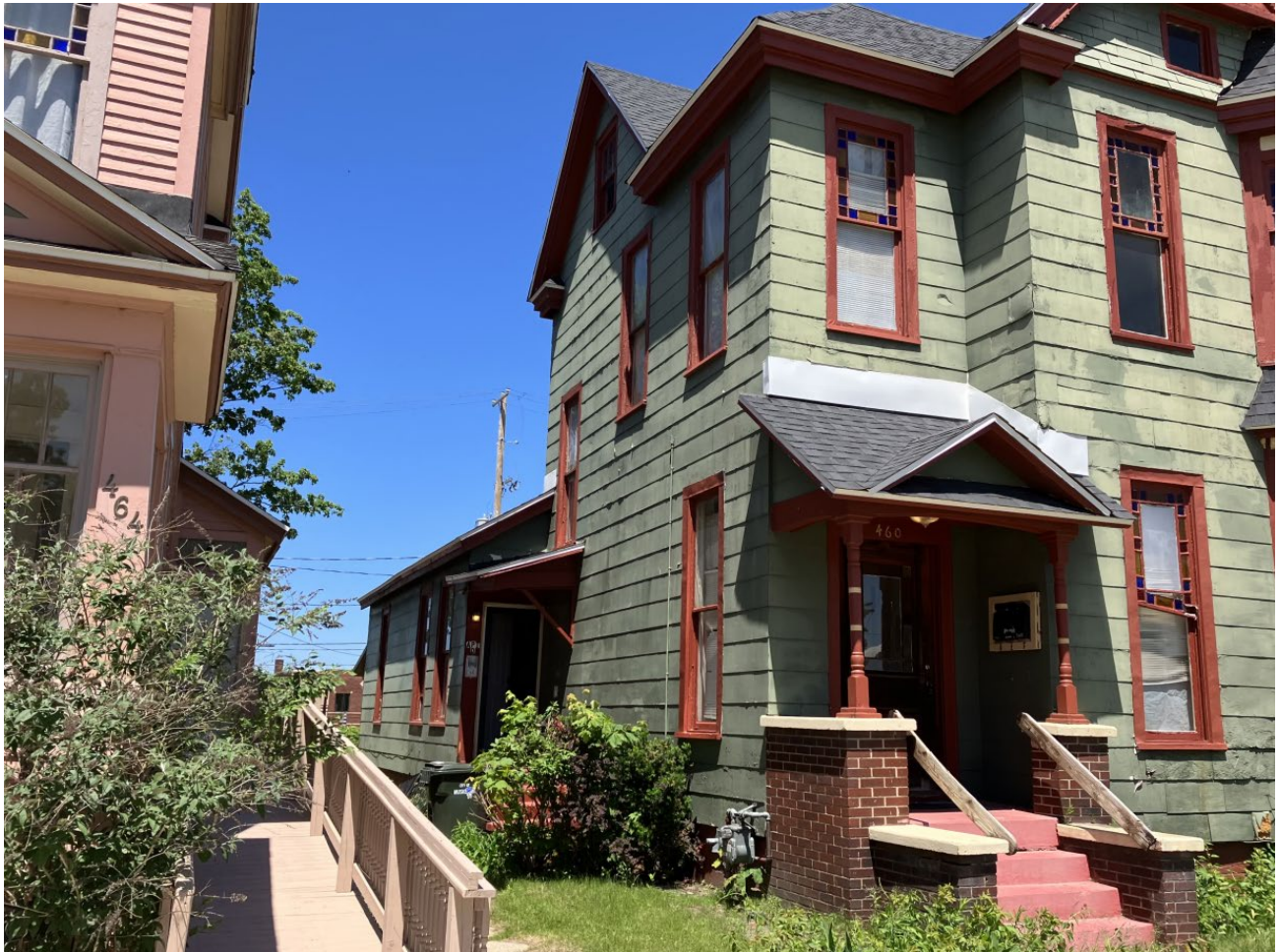
View of front porch and west elevation from W. Clay Avenue, looking north.
