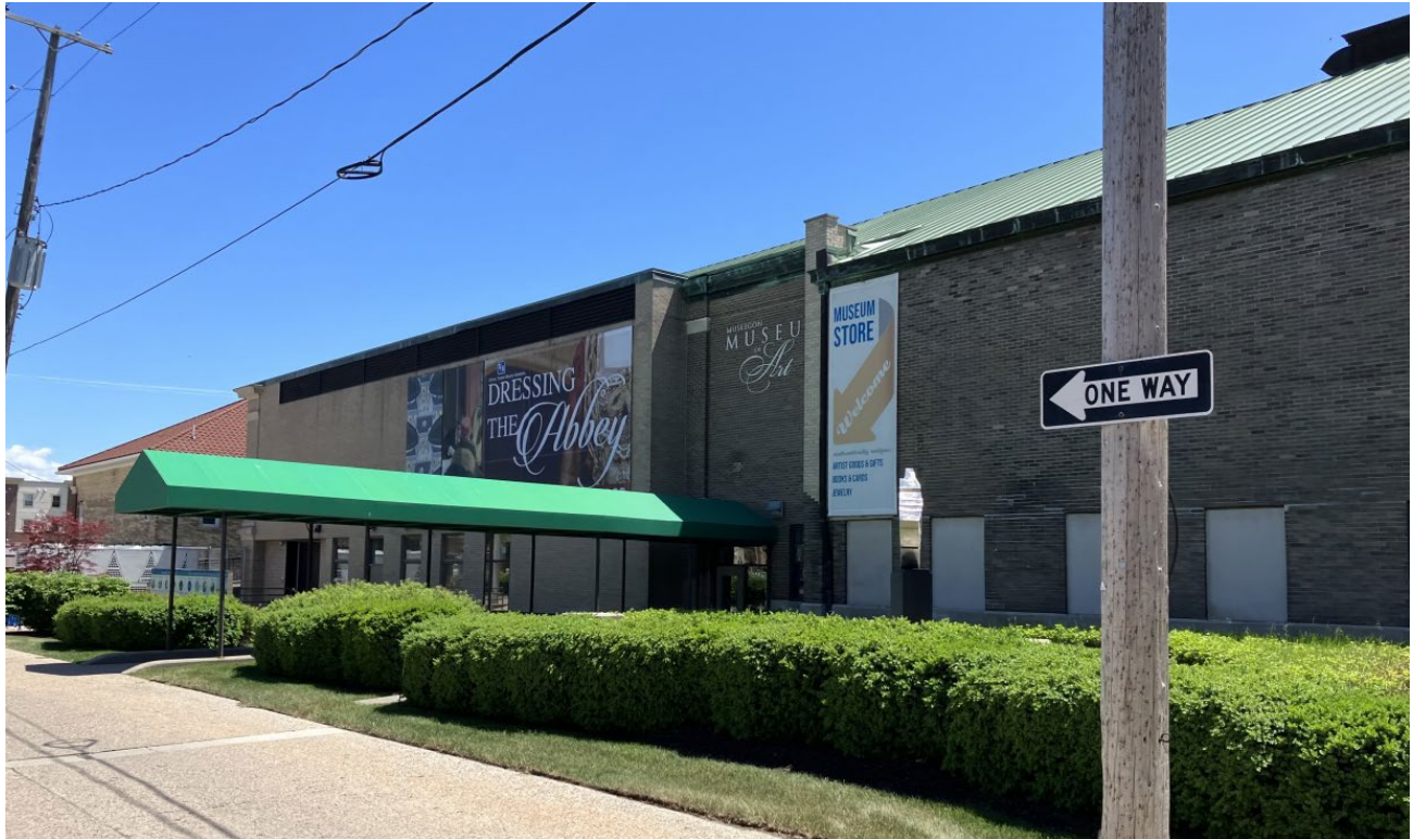
Current view of north entrance and alley, looking east.
