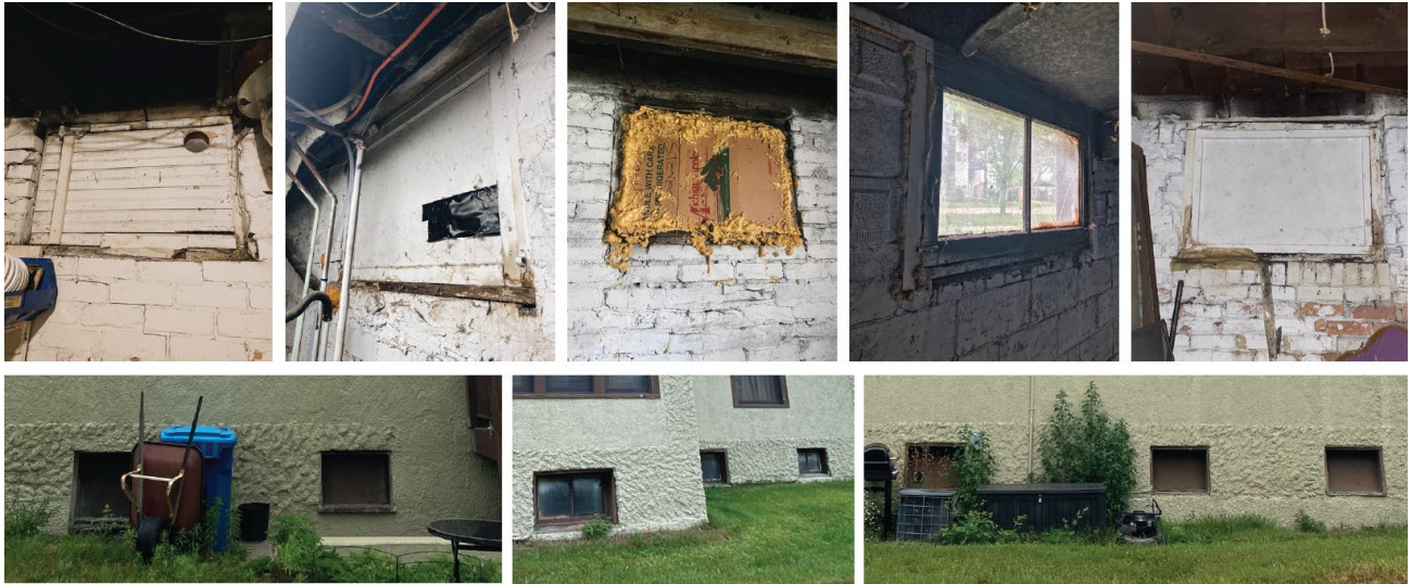
Existing conditions of basement windows. Boarded windows are often missing entirely, as depicted in interior photos.
