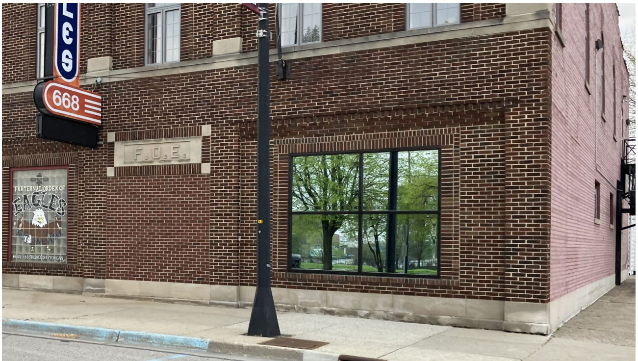
View of replacement window from W. Western Avenue.
