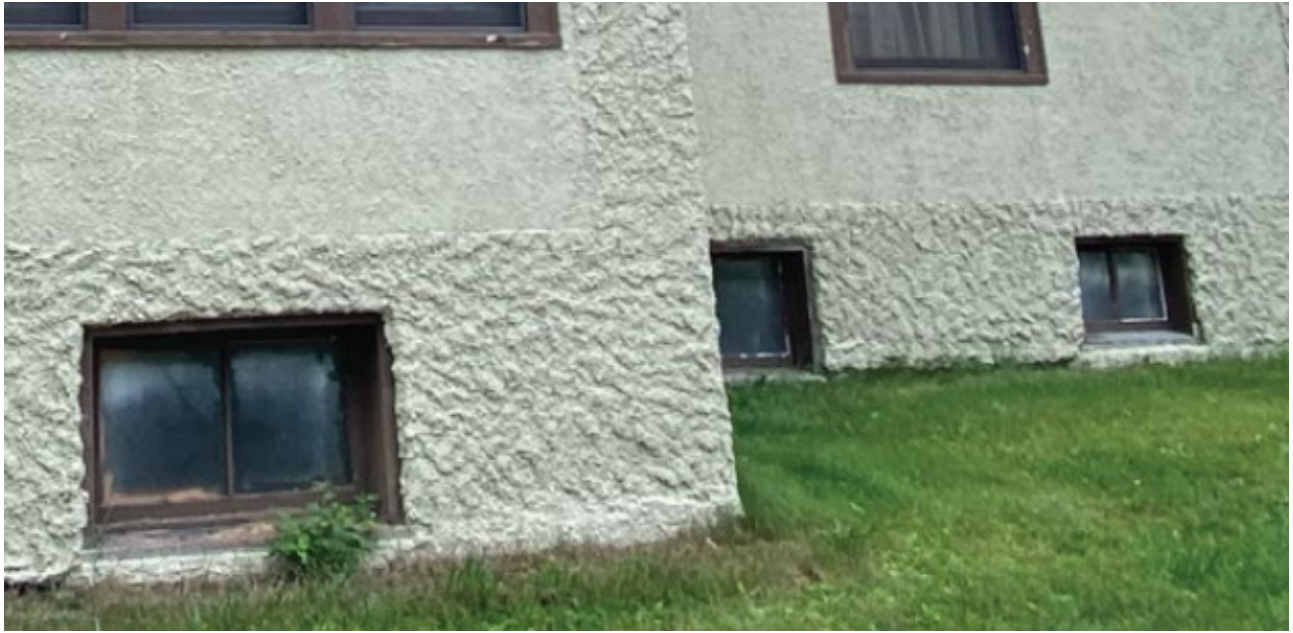
View of the three remaining basement windows on the east elevation, as viewed from 5 th Street.
