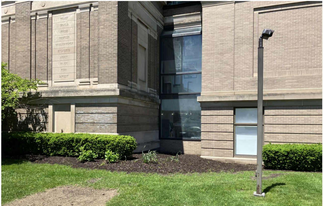
Current connection between original museum building and past building addition. Window on left is proposed to be replaced with a new entry door.
