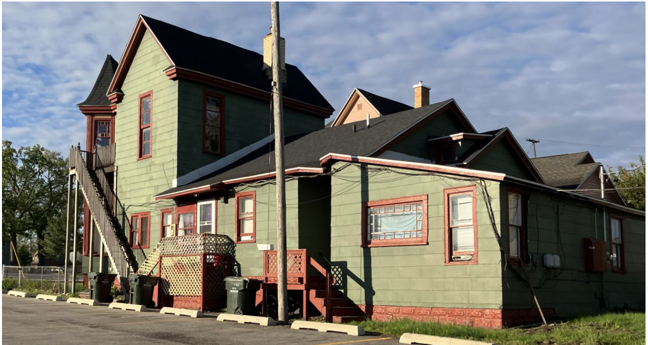
View of east elevation from rear alley, looking south.
