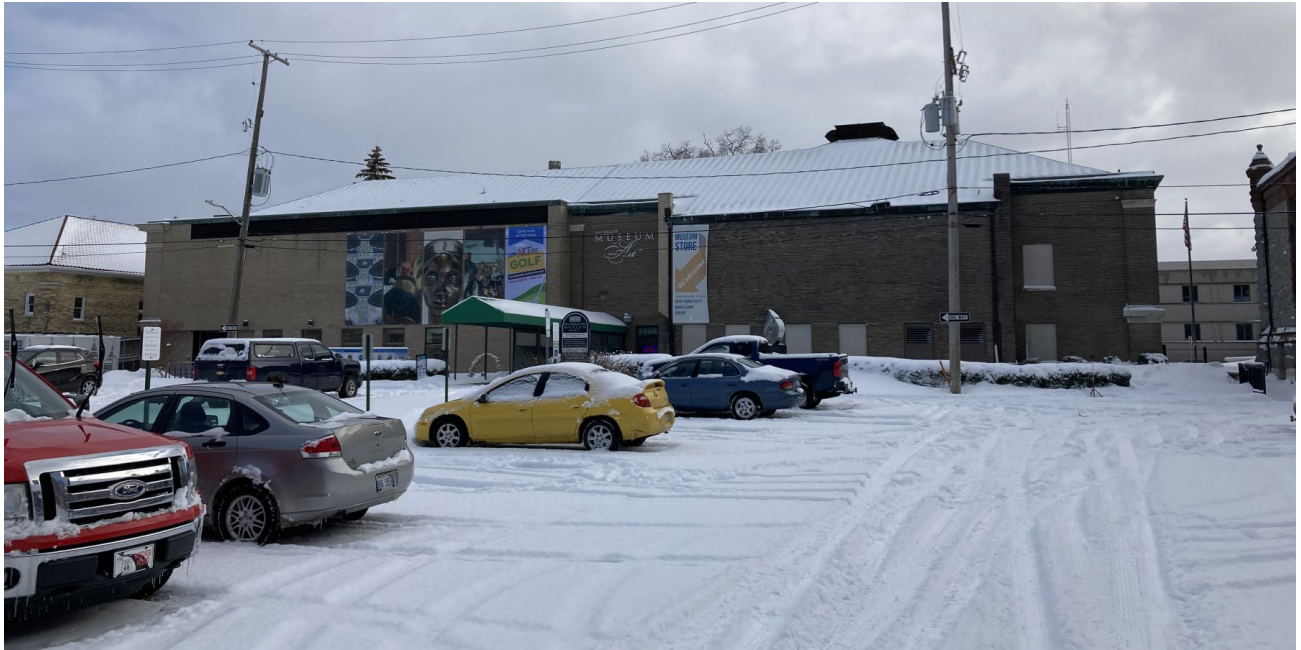
View of existing north elevation from W. Clay Avenue (January 2022).
