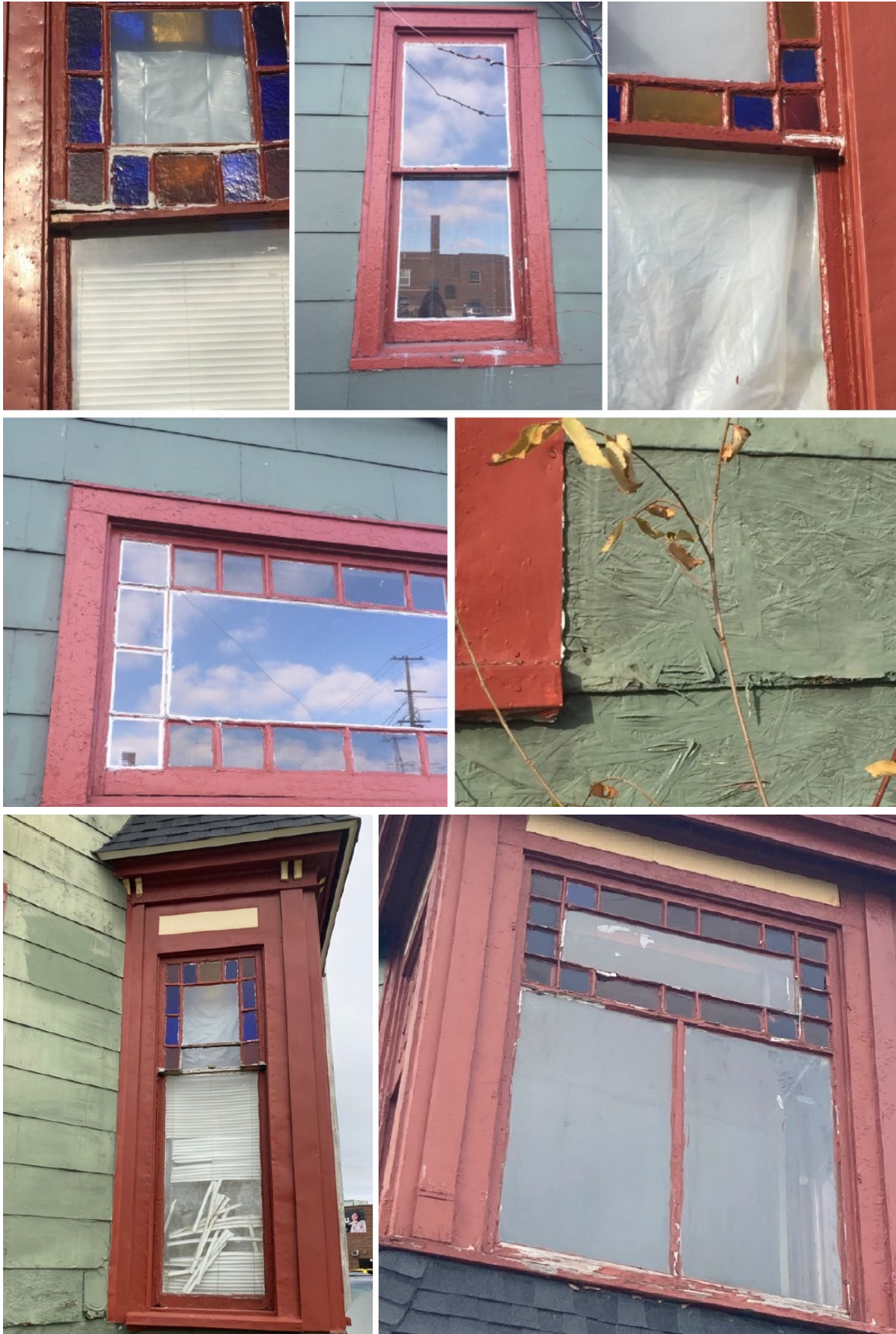
Existing window and siding conditions.
